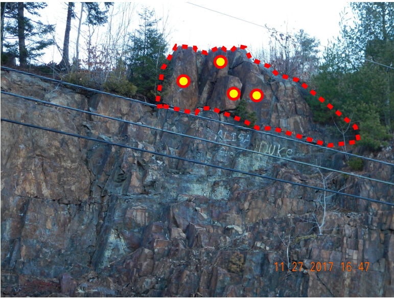
PHOTO 3 (ABOVE): CLOSEUP VIEW.
