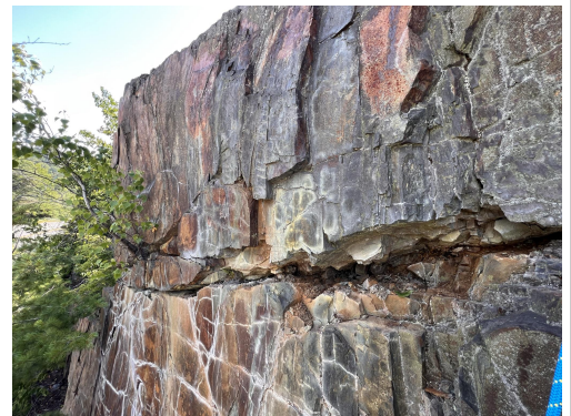
PHOTO 3 (ABOVE): SIDE VIEW OF NORTHERN PORTION OF AREA 3A (LOOKING SOUTH) WITH OPEN BASAL JOINT VISIBLE.
