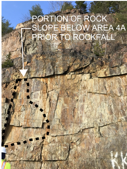
PHOTO 3 (ABOVE): ROCK SLOPE BELOW AREA 4A AS IT EXISTED ON 29 NOVEMBER 2017.
