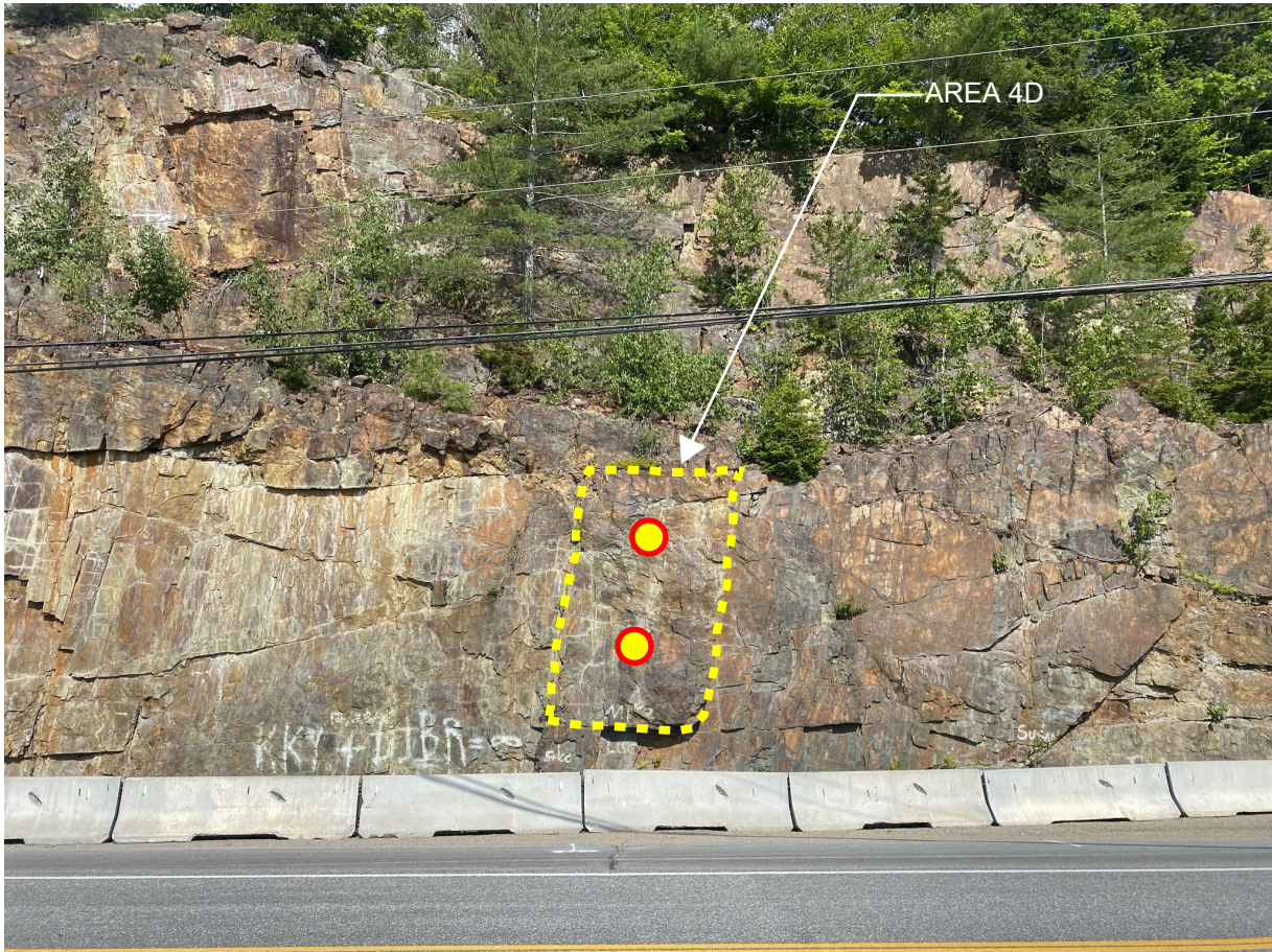
PHOTO 1 (ABOVE): OVERALL VIEW.
