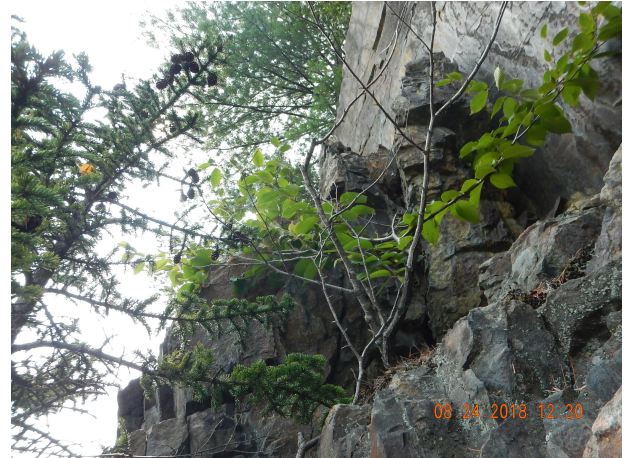
PHOTO 2 (ABOVE LEFT): SIDE VIEW (LOOKING NORTH) WITH OPEN BACK JOINT VISIBLE.
