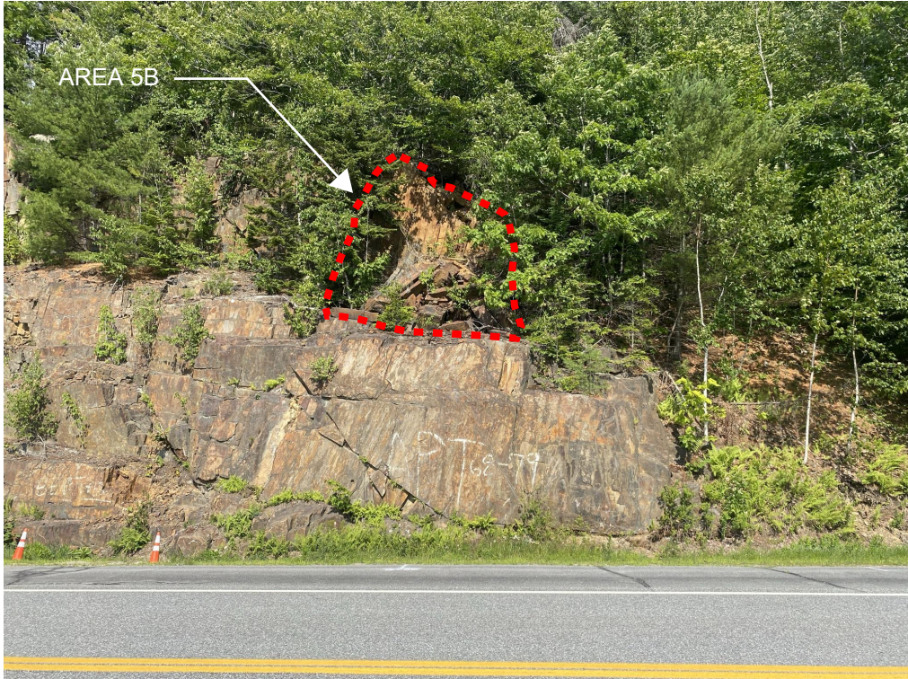
PHOTO 1 (ABOVE): OVERALL VIEW.
