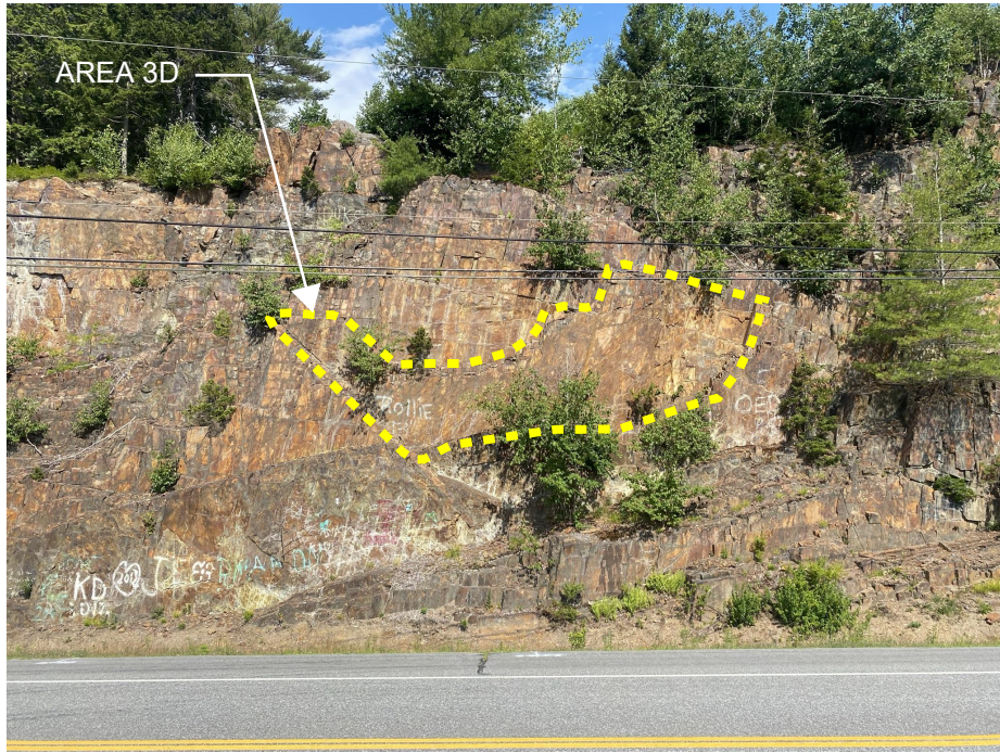
PHOTO 1 (ABOVE): OVERALL VIEW.
