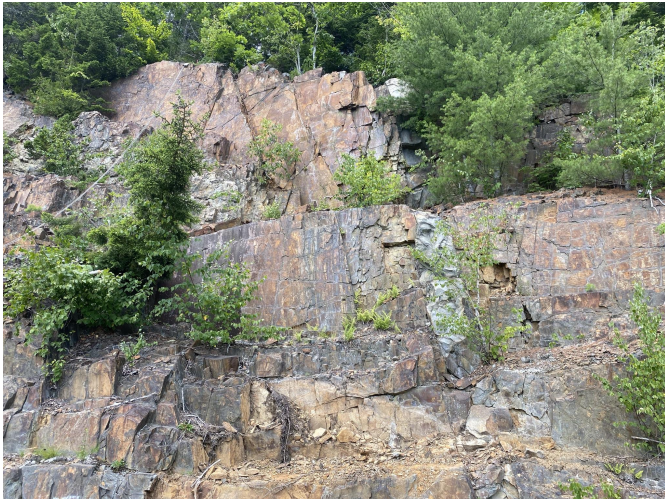
PHOTO 2 (ABOVE): CLOSEUP VIEW.
