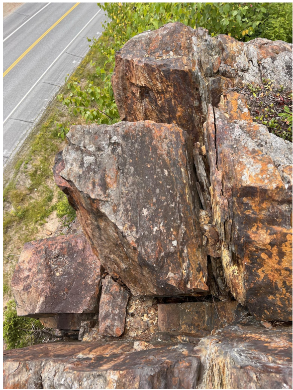
PHOTO 4 (RIGHT): TOP VIEW LOOKING DOWN WITH OPEN BACK AND SIDE JOINTS VISIBLE.
