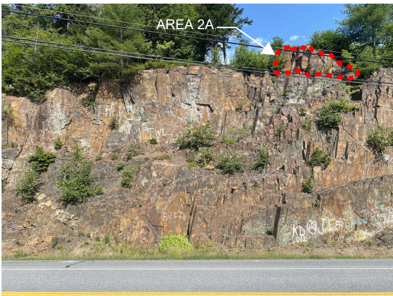
PHOTO 1 (ABOVE): OVERALL VIEW.
