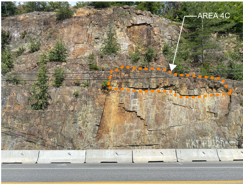
PHOTO 1 (ABOVE): OVERALL VIEW.
