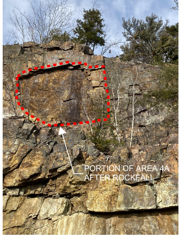
PHOTO 2 (ABOVE): AREA 4A AS IT EXISTED ON 18 MARCH 2022.
