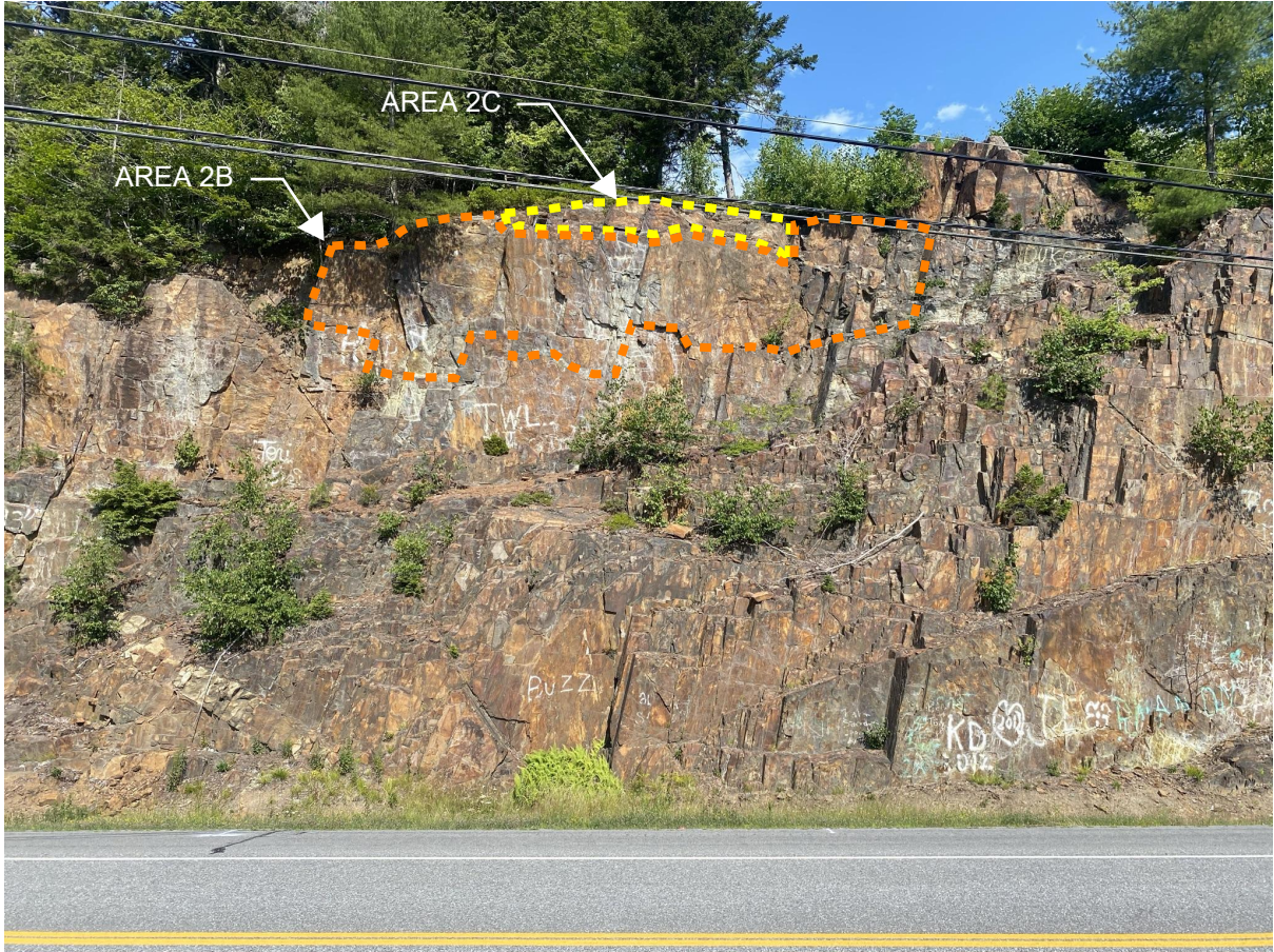
PHOTO 1 (ABOVE): OVERALL VIEW.
