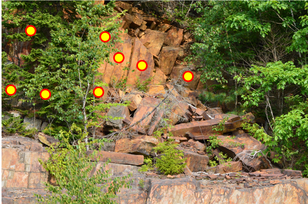
PHOTO 2 (ABOVE): CLOSEUP VIEW.
