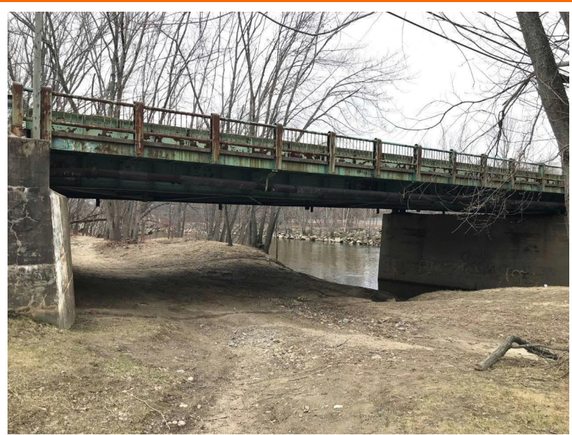
Photograph 4: Mexico side of the bridge, view from the north
