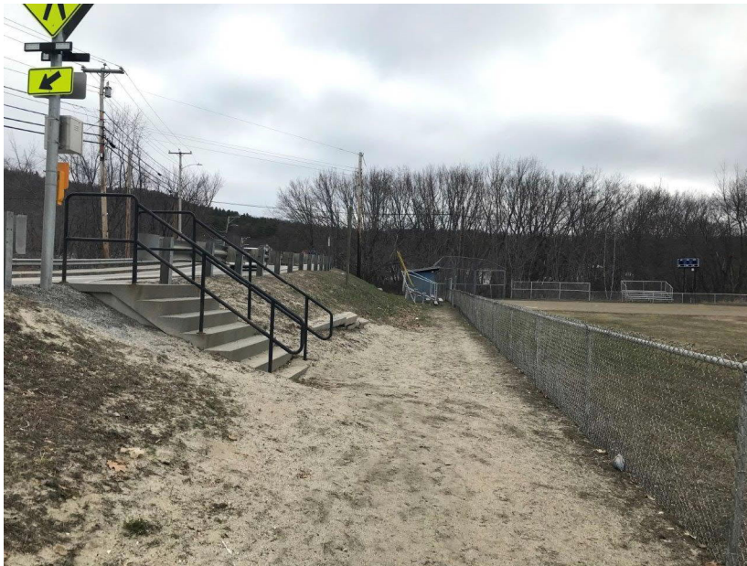
Photograph 1: Existing ballpark access stairs (to be replaced with stairs and ramp)
