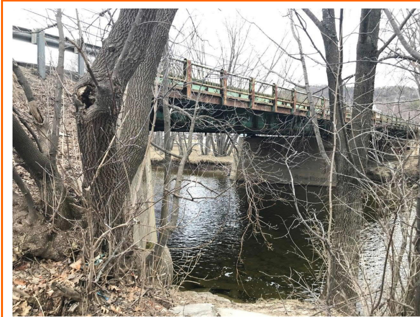
Photograph 3: Rumford side of the bridge, view from the south
