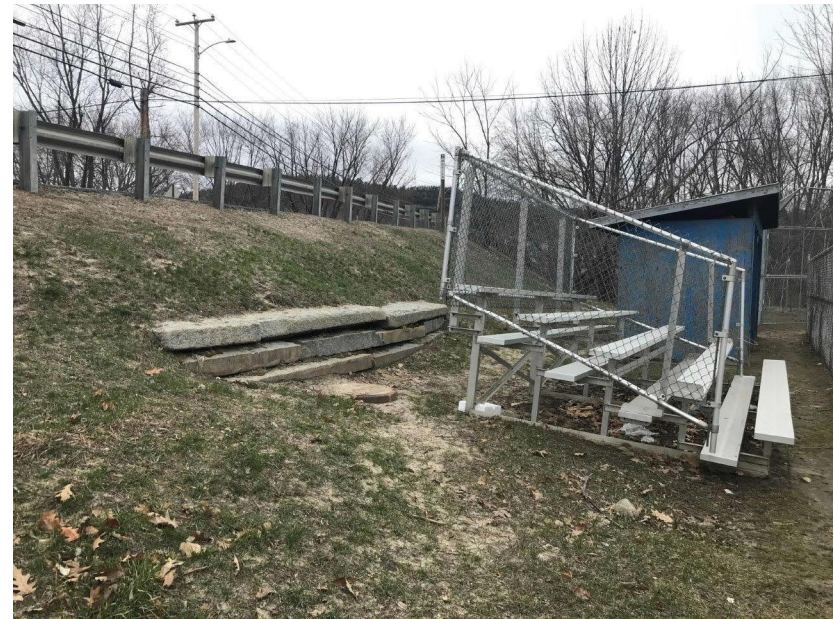
Photograph 2: Existing ballpark structures to be demolished for bridge construction
