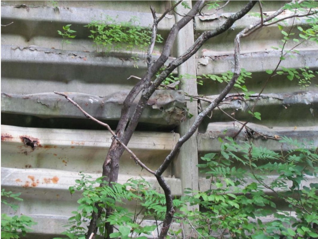
Deteriorated steel
