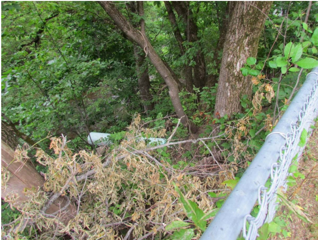
Drain pipe over bin wall
