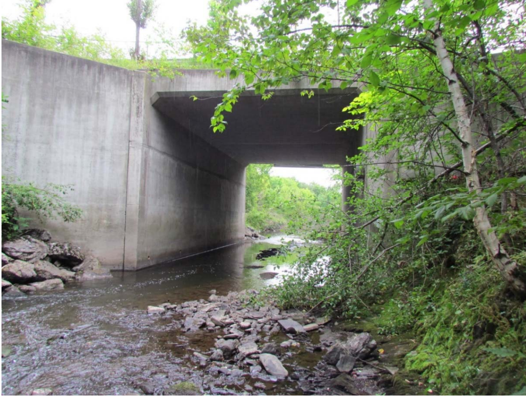
Looking downstream at Bridge 0181
