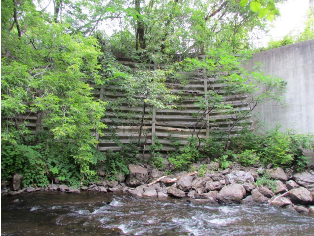
Downstream portion of bin wall
