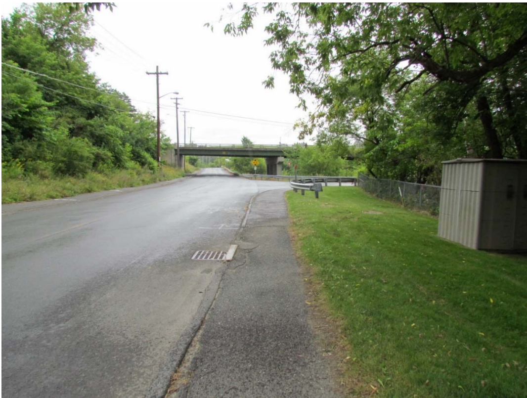
Roadside adjacent to bin wall looking east
