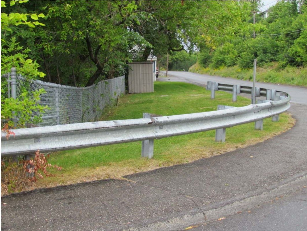
Roadside adjacent to bin wall looking west
