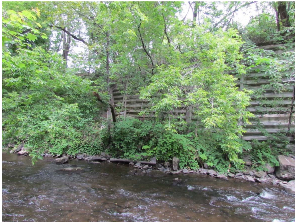
Upstream portion of bin wall
