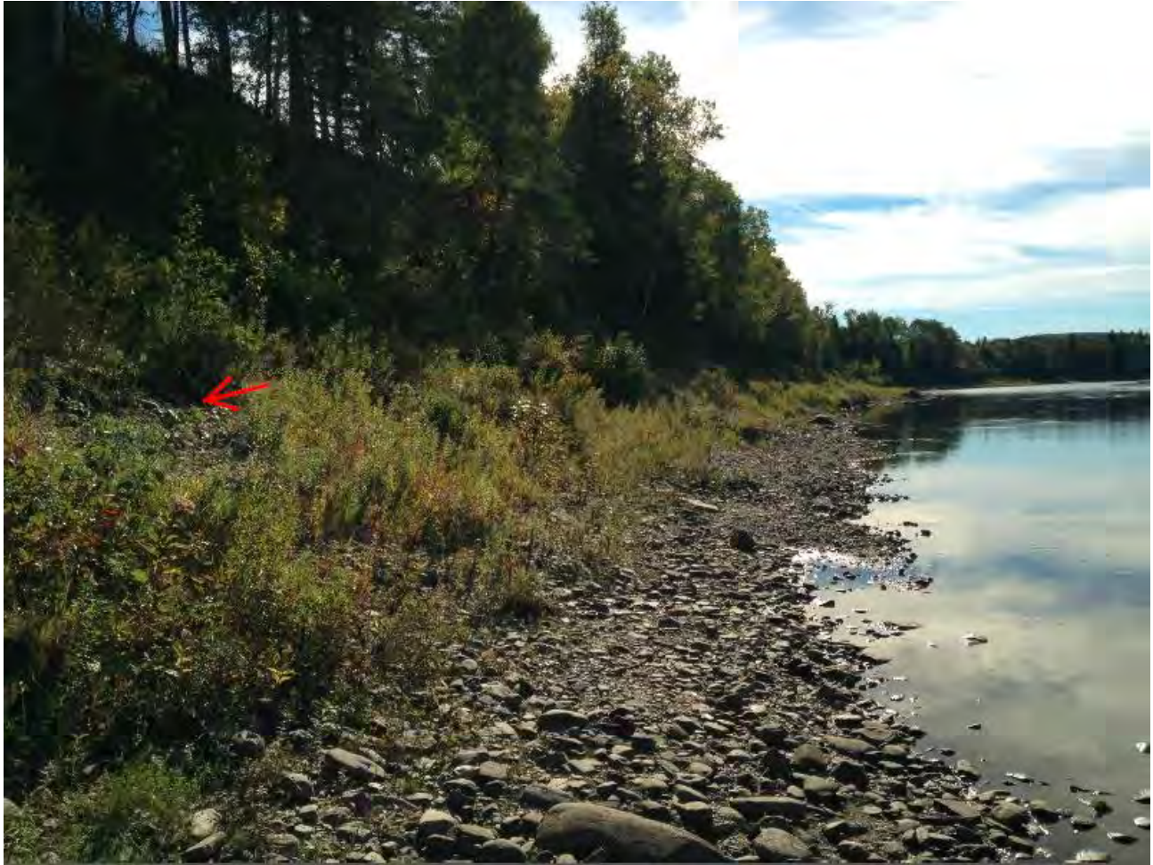
Figure 1. Eroding bank at Allagash site.
