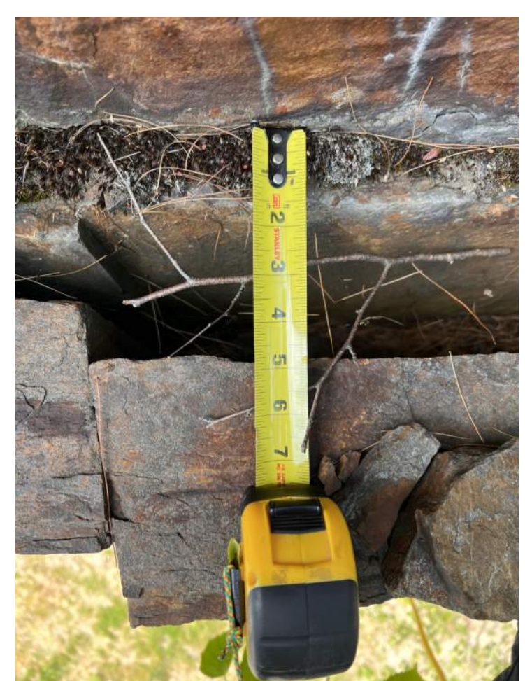
AREA 3B SEPARATION OF FOLIATION PLANES (TYP.; LOOKING DOWN)
