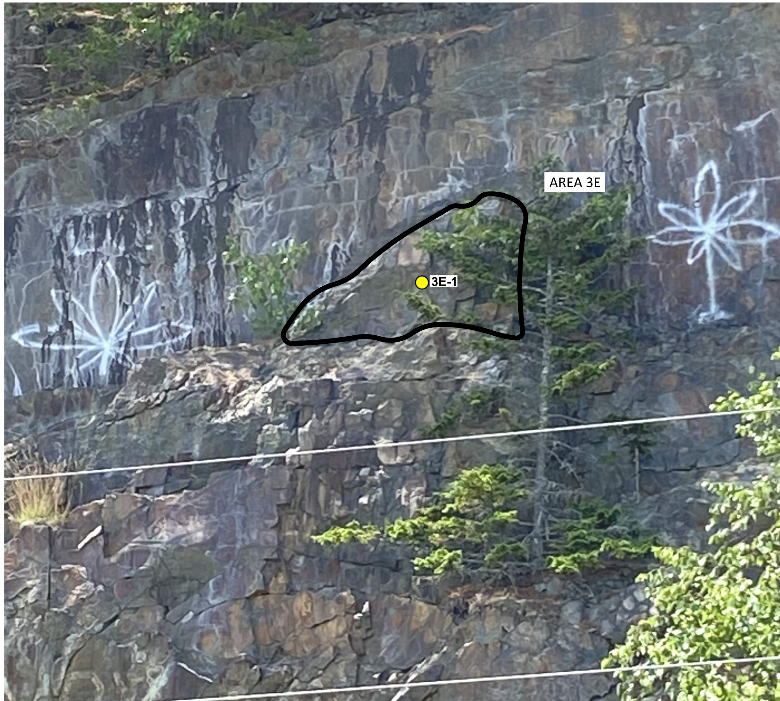
CLOSEUP VIEW (LOOKING WEST)
