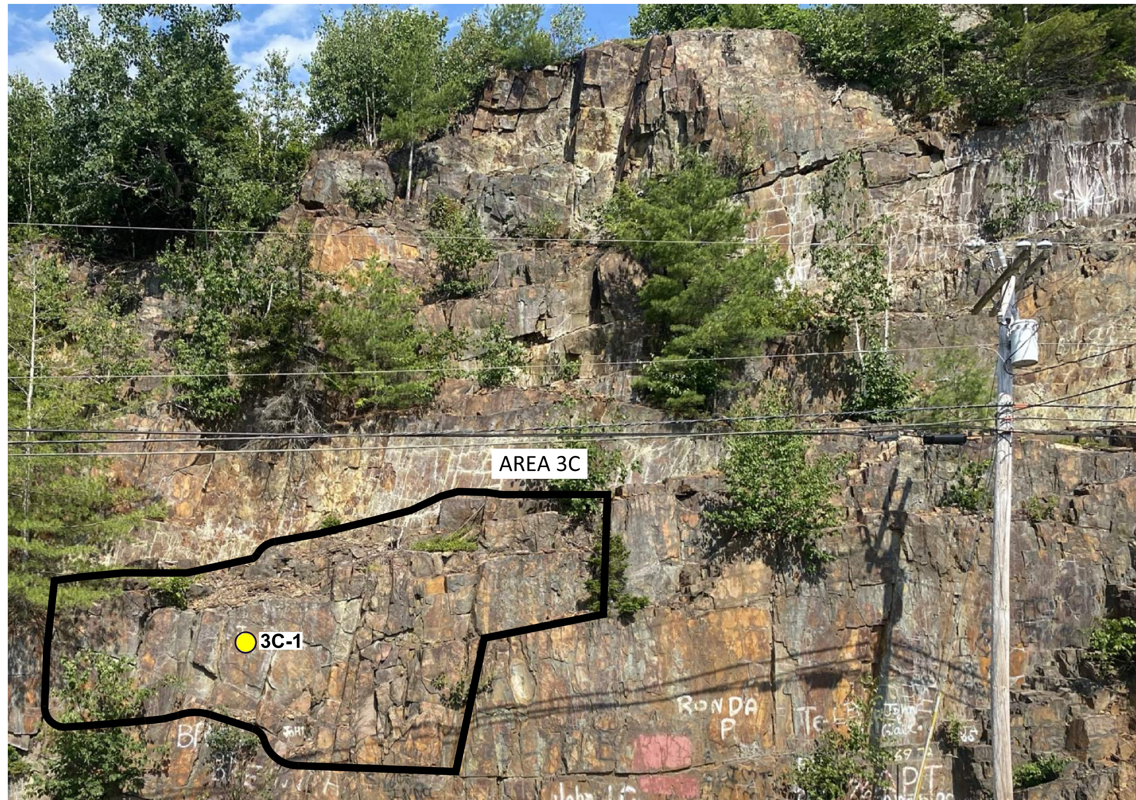
AREA 3C OVERALL VIEW (LOOKING WEST)
