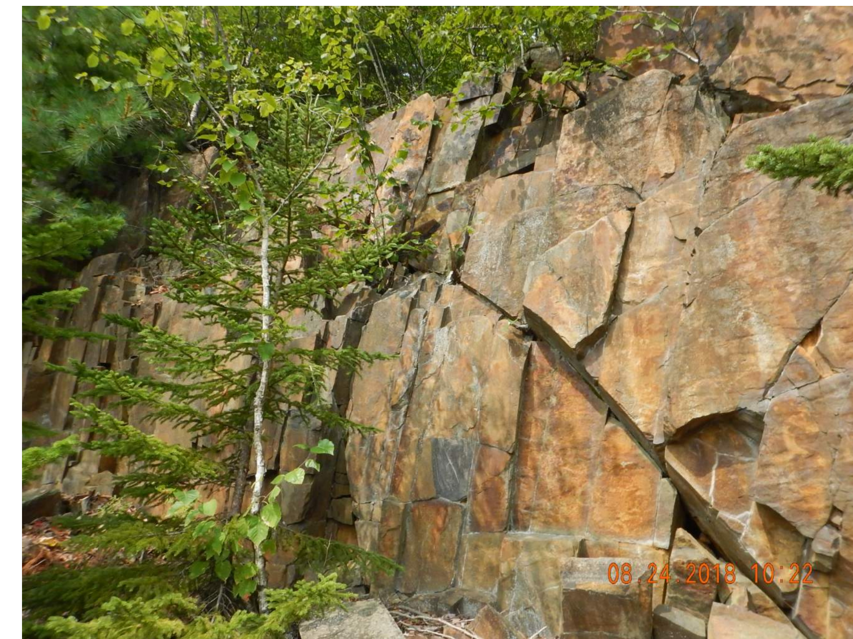
CLOSEUP / SIDE VIEW (LOOKING SOUTH)
