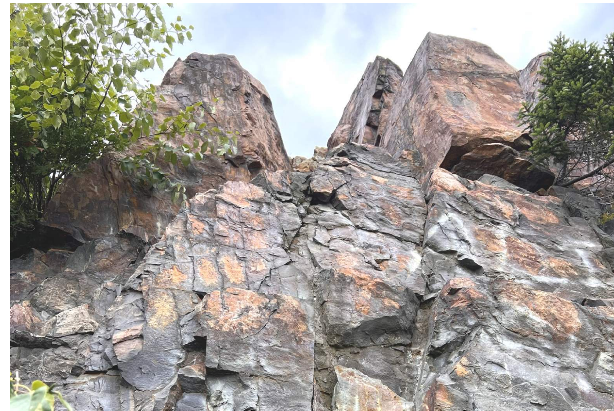
BOTTOM / CLOSEUP VIEW (LOOKING UP AND WEST)
