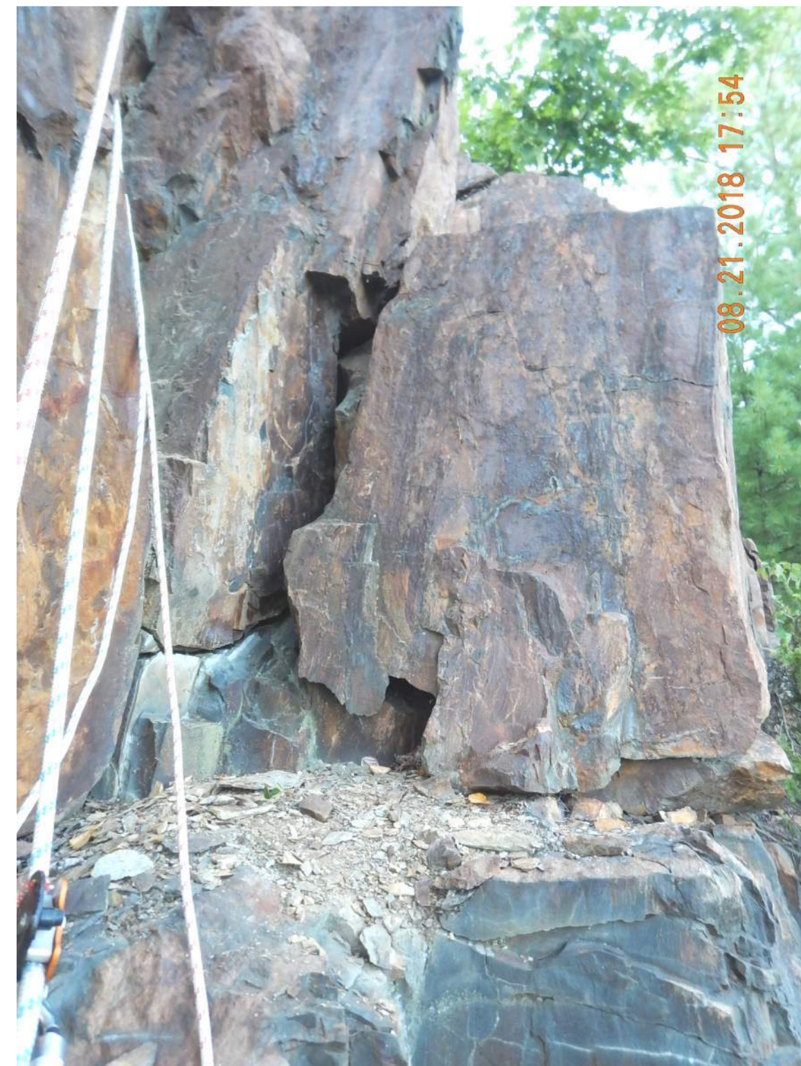
SIDE VIEW (LOOKING NORTH)
