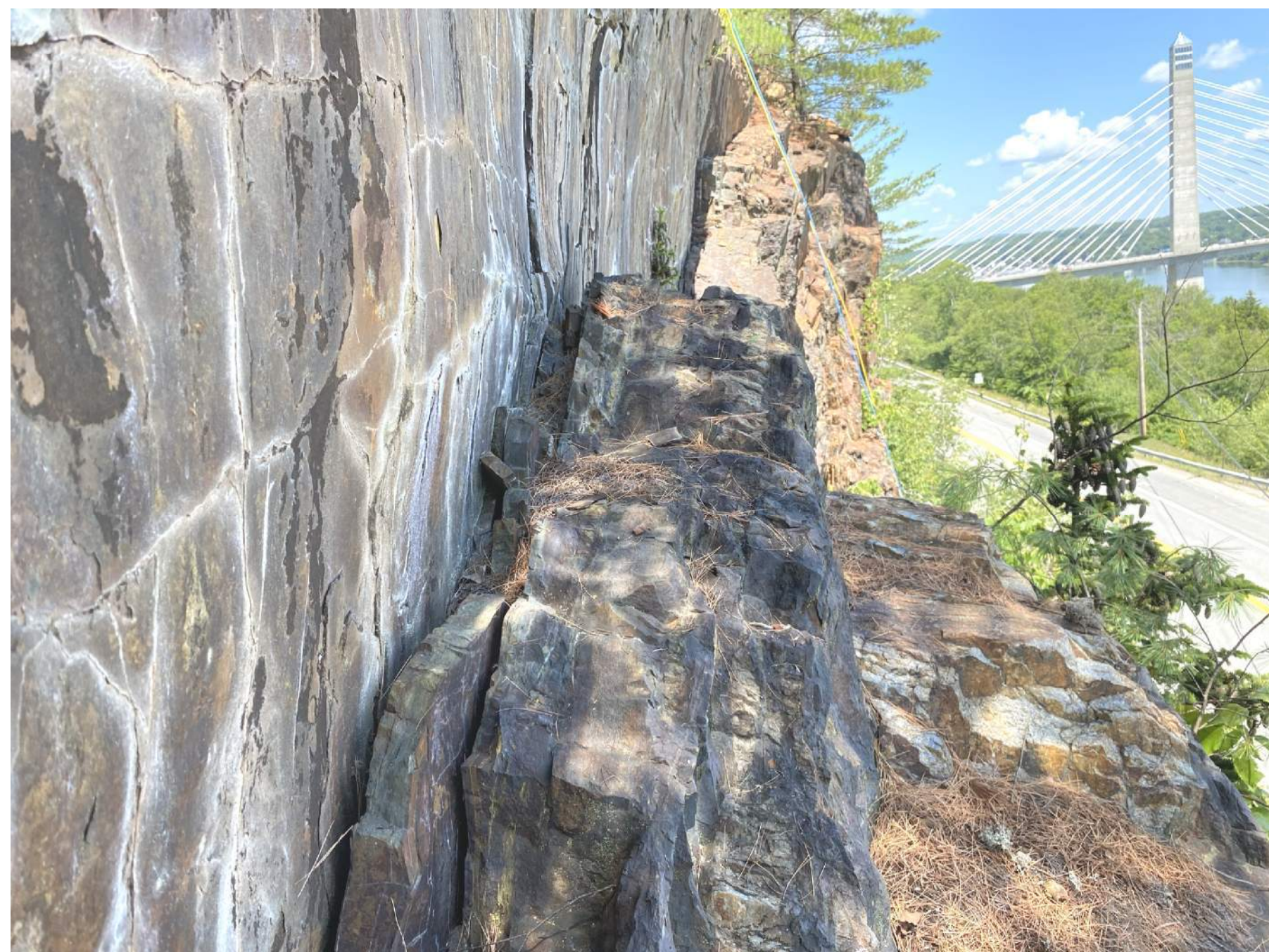
CLOSEUP VIEW (LOOKING NORTH)
