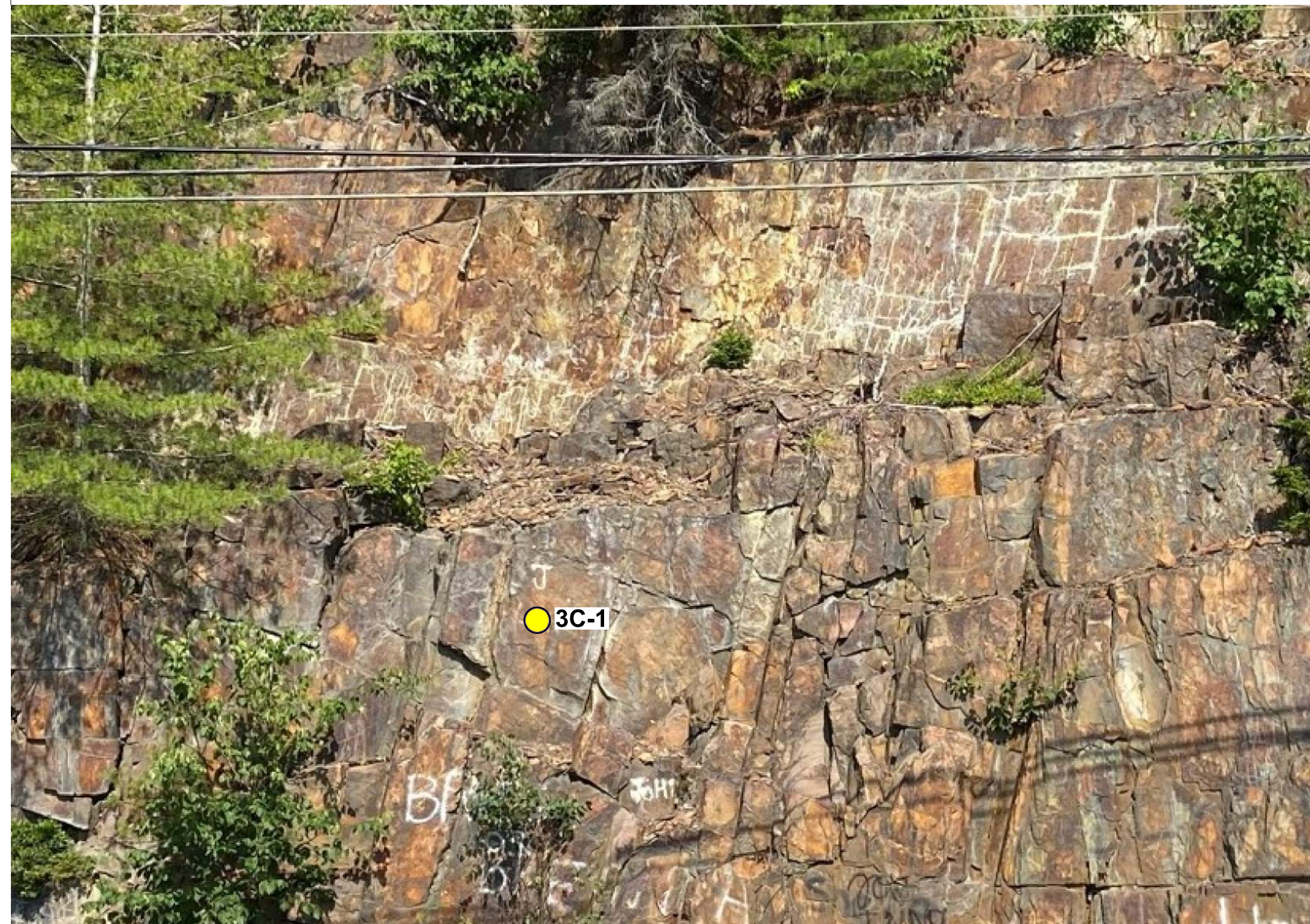
AREA 3C CLOSEUP VIEW (LOOKING WEST)
