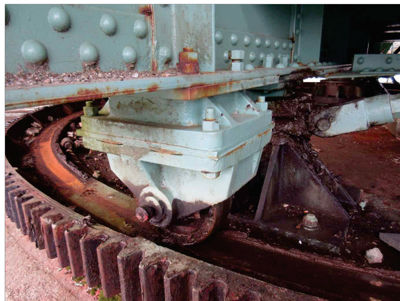
P2 BALANCE WHEEL ASSEMBLY
