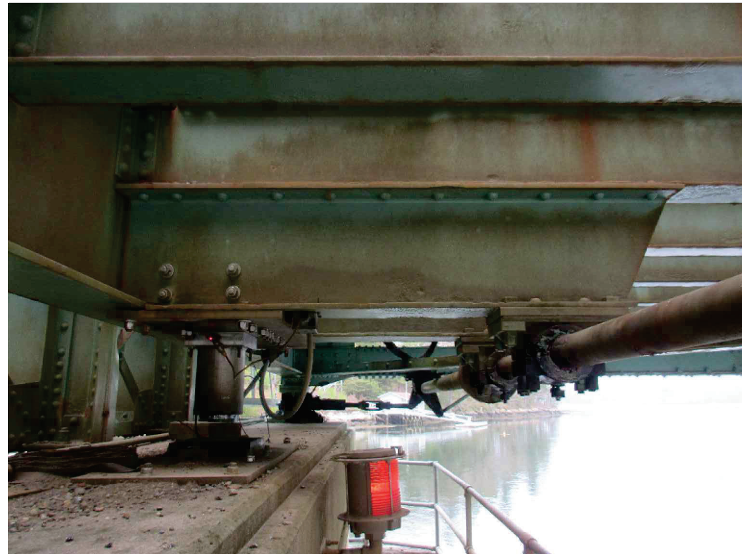
P2 END WEDGE SHAFT ASSEMBLY
