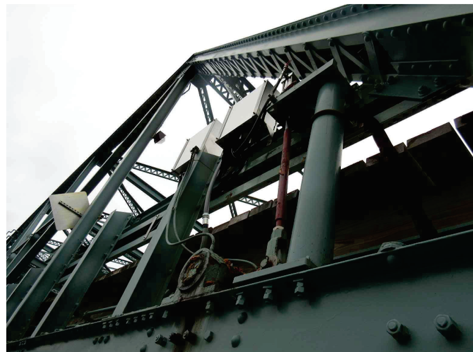
P3 END WEDGE ACTUATOR & CONTROLS
