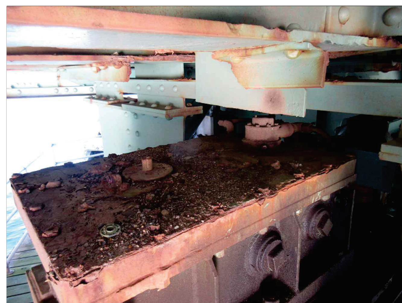
P5 ENCLOSED GEAR REDUCER (SOUTHPORT)
