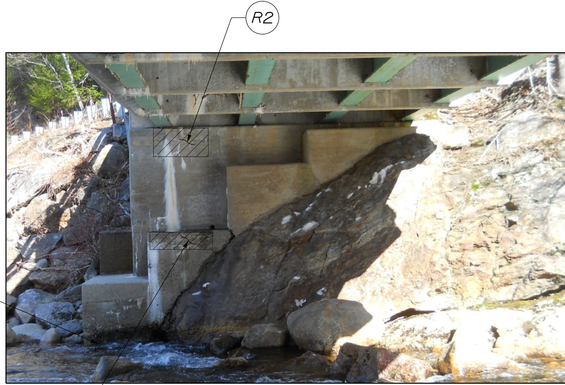
NORTH ABUTMENT ELEVATION
