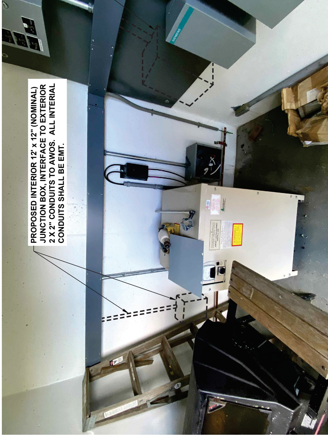
5 ELECTRICAL VAULT MODIFICATIONS 2
