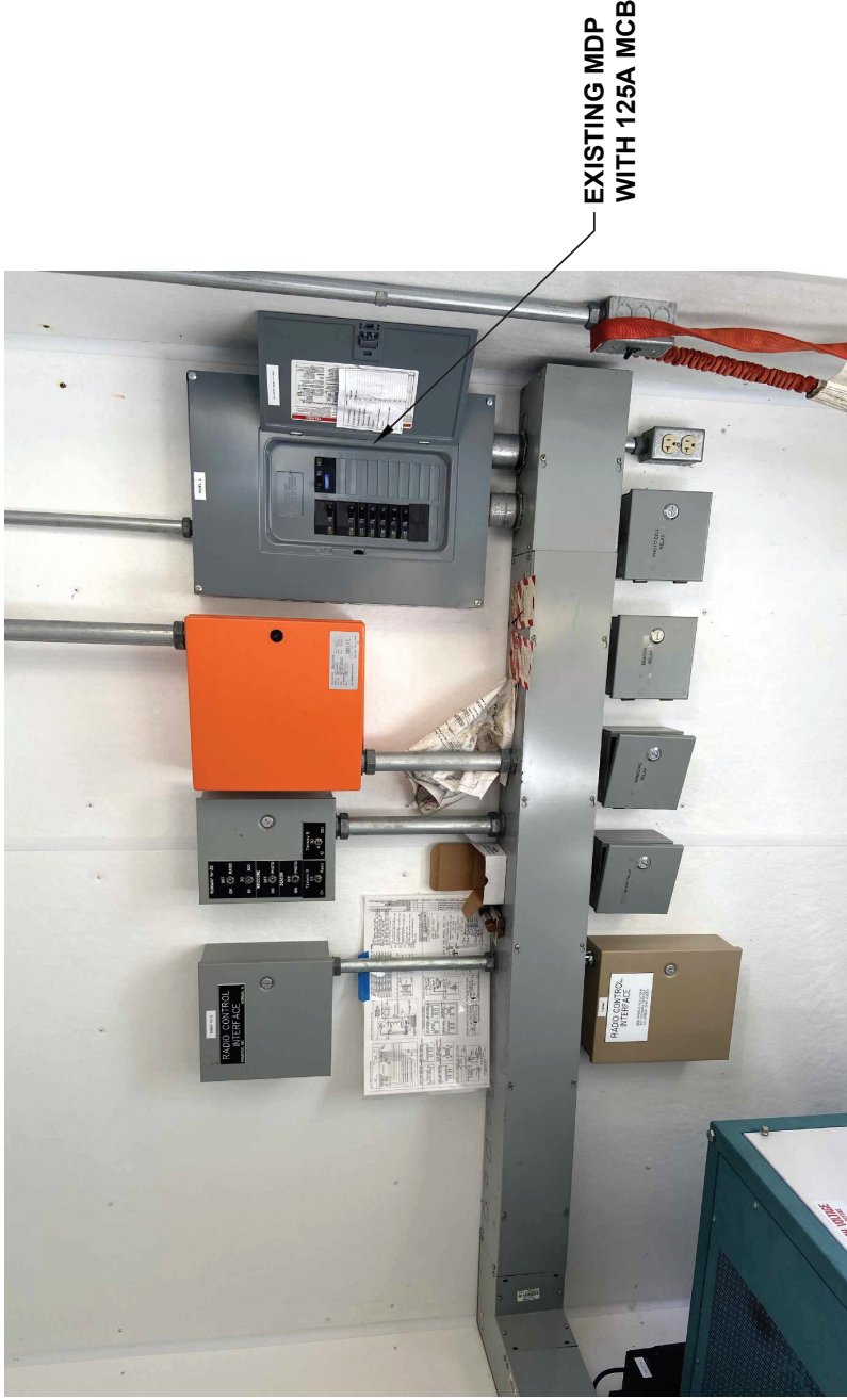
4 EXISTING JUNCTION BOX DETAIL
