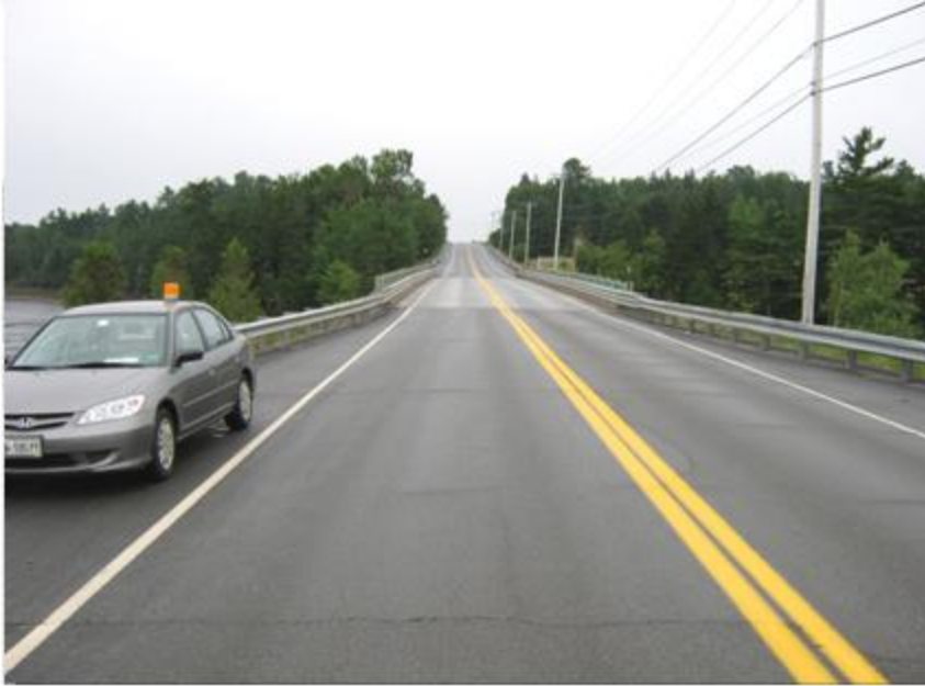
Roadway looking South
