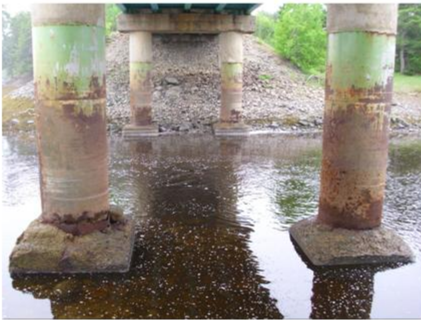
Looking south Piers
