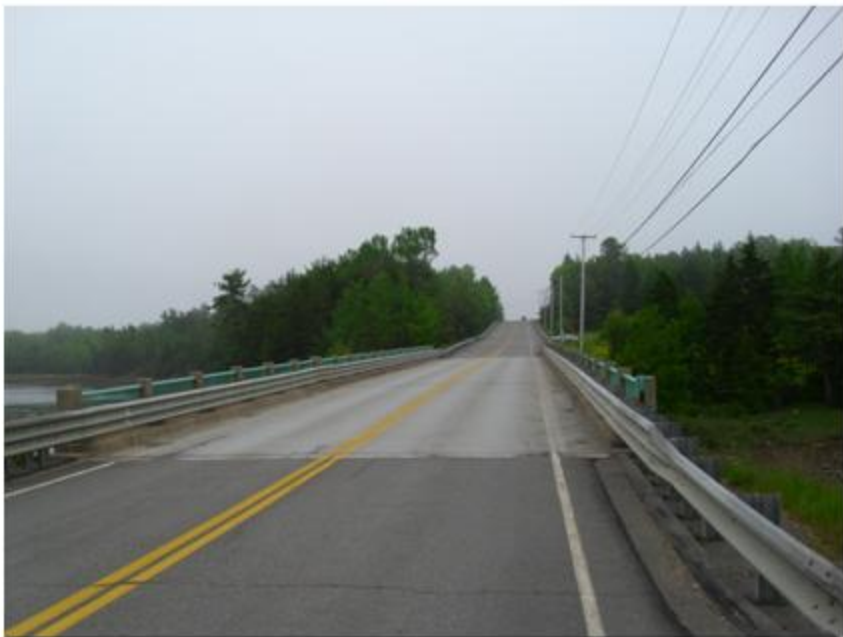
North Approach Looking South
