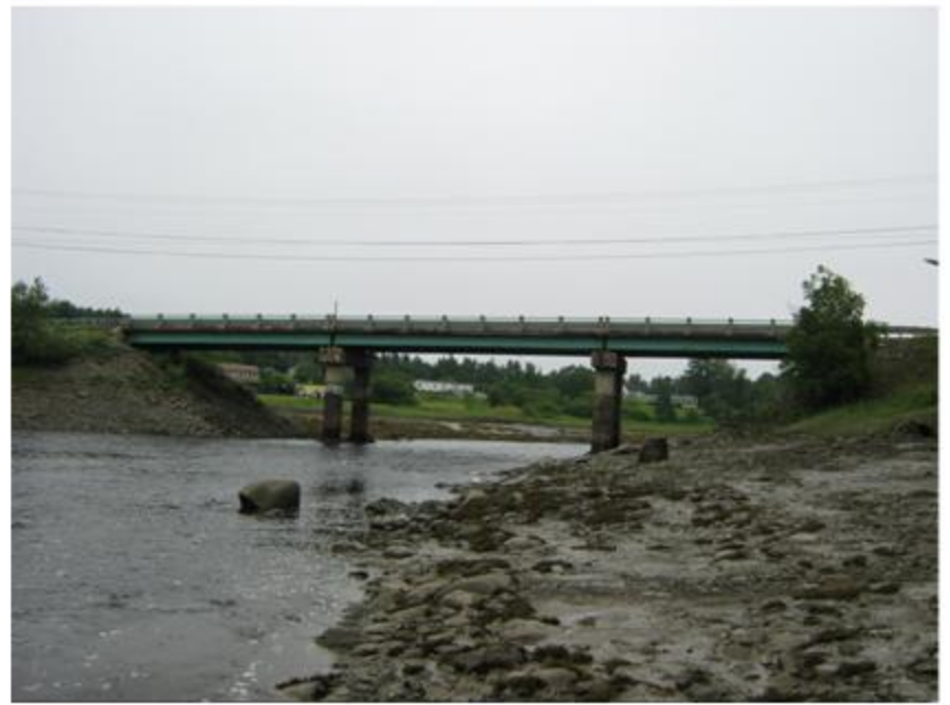
Looking down stream
