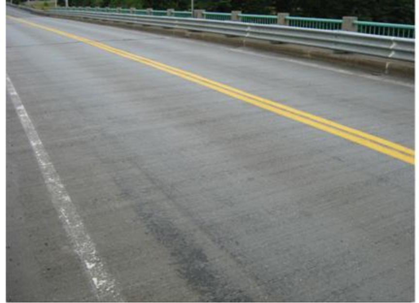
General view of wearing surface
