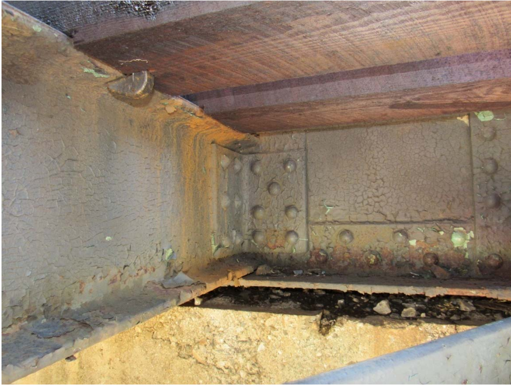
MP 113.14 – Grindstone Approach – Stringer Connection
