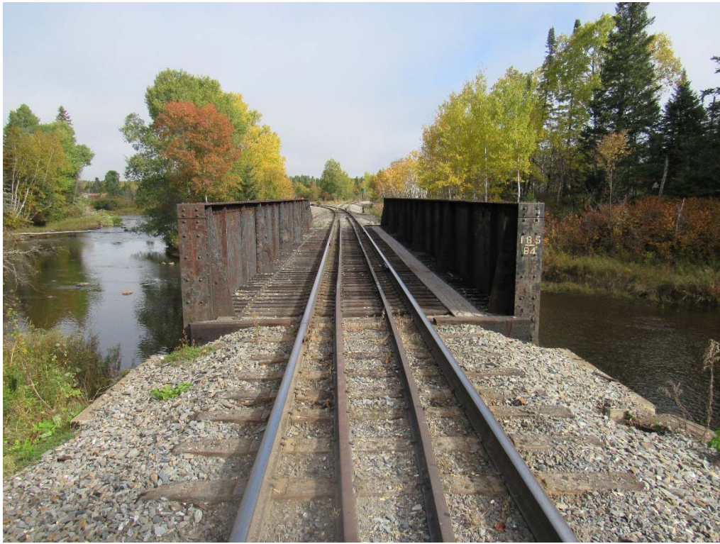
MP 185.84 – Squapan Stream – Looking North
