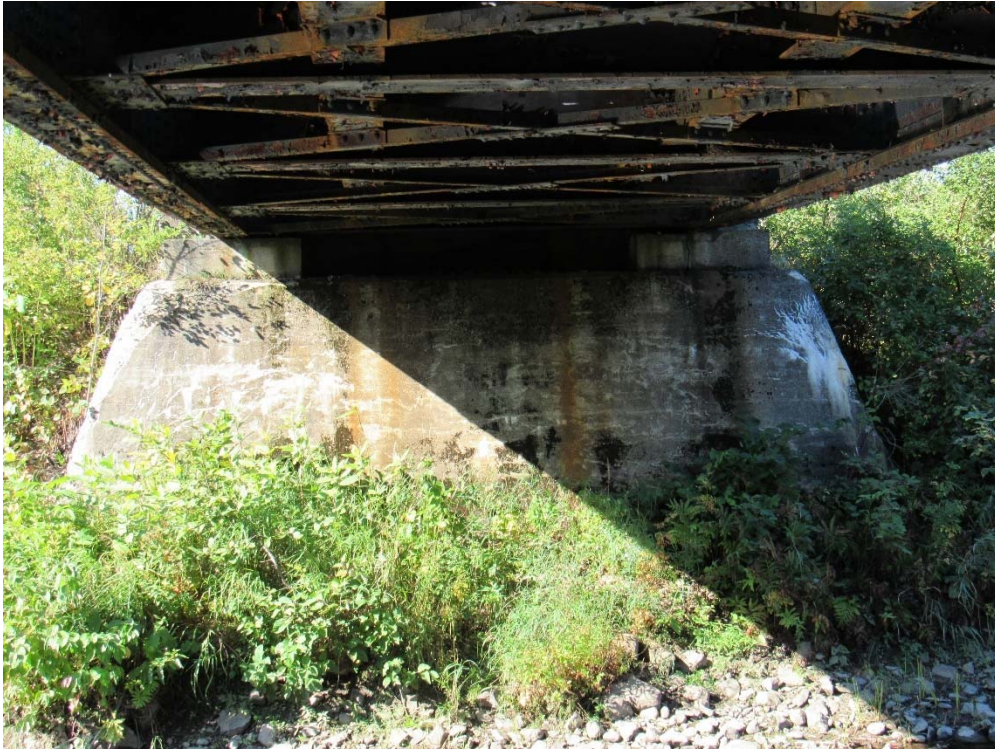
MP 139.66 – W. Branch Mattawamkeag River – South Abutment
