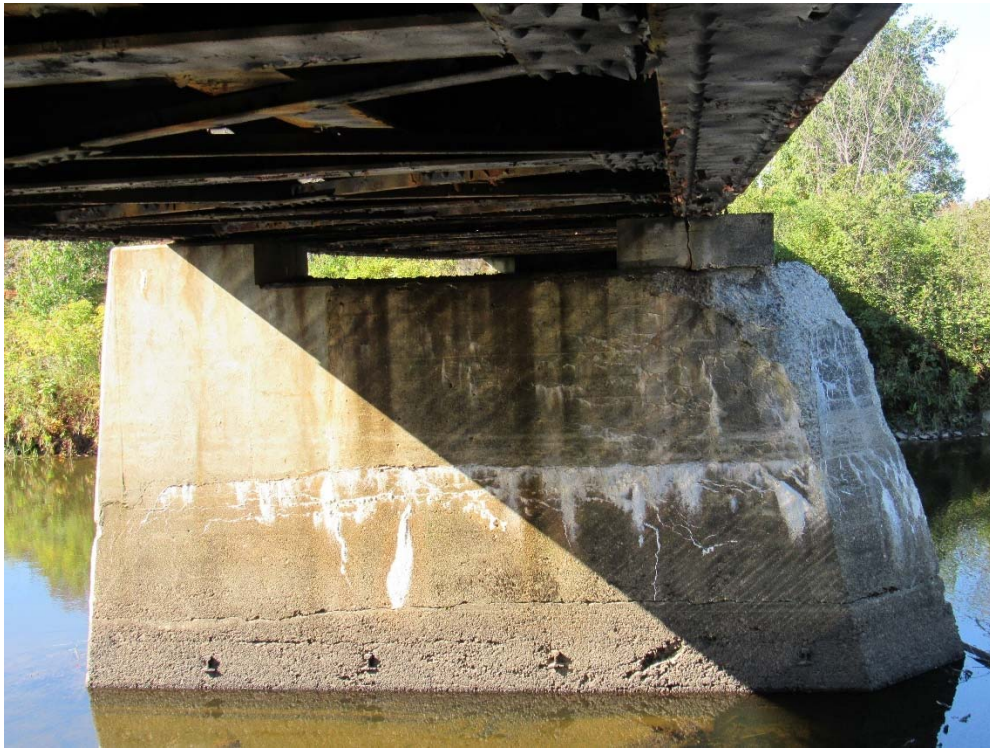
MP 139.66 – W. Branch Mattawamkeag River – Center Pier, Looking South
