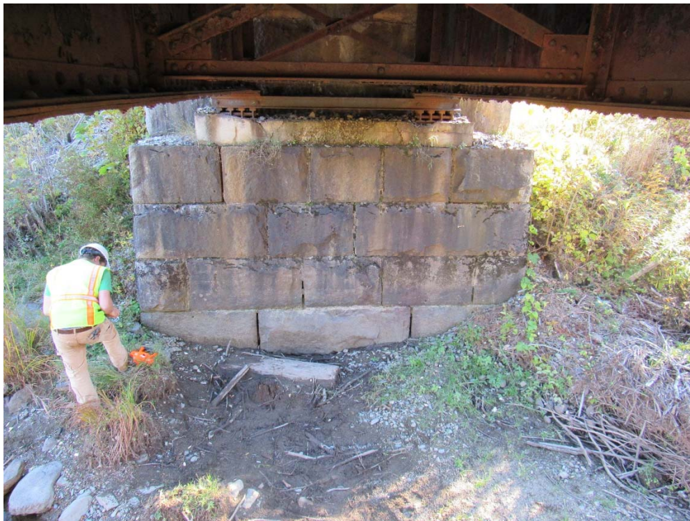
MP 179.34 – N. Branch Blackwater River – South Abutment
