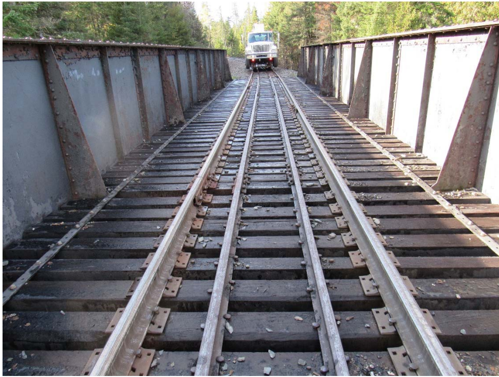
MP 161.03 – Smith Brook – Looking South
