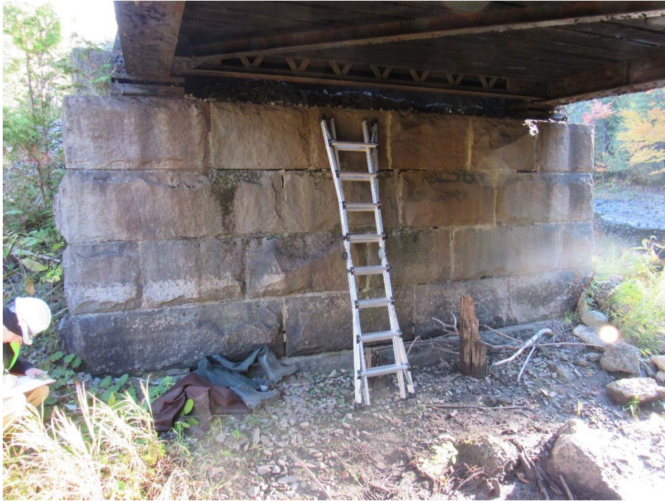
MP 151.54 – E. Branch Mattawamkeag River – North Abutment
