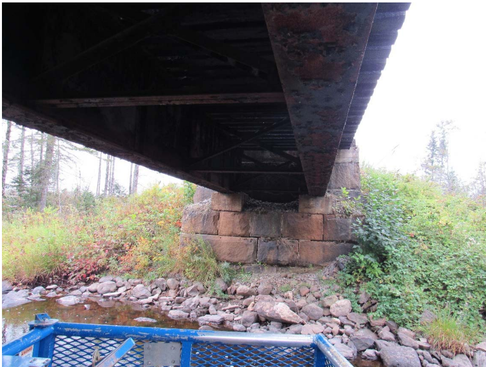
MP 167.76 – Beaver Brook – North Abutment
