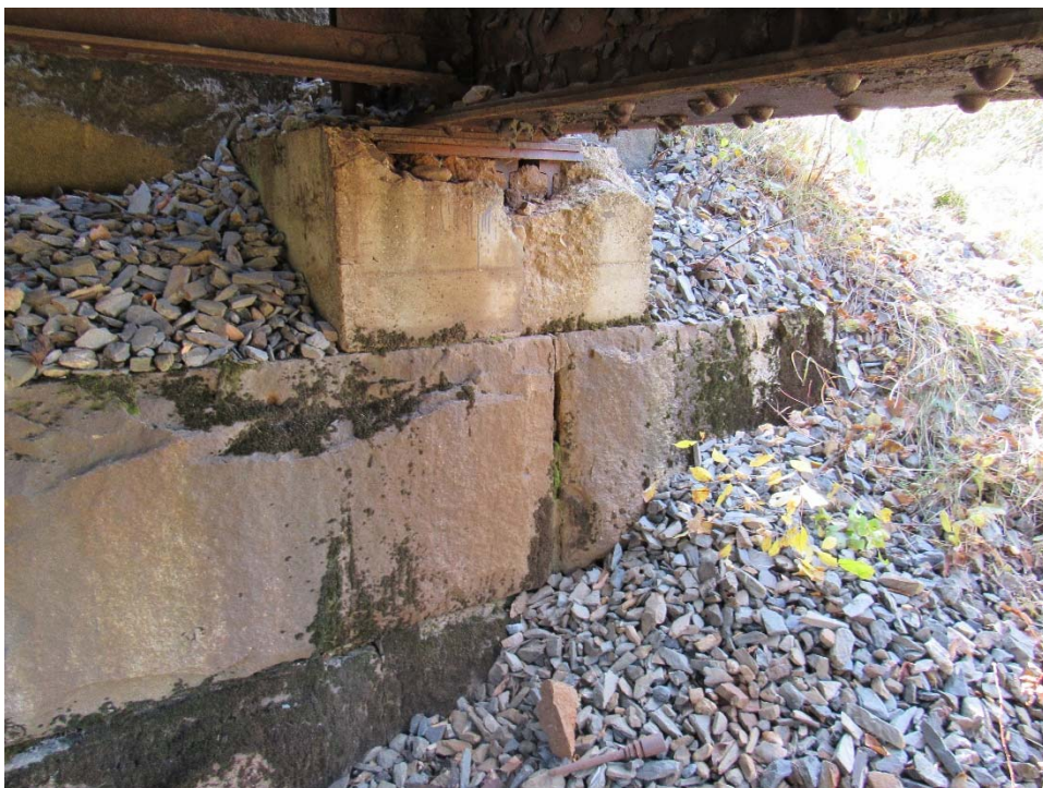
MP 167.76 – Beaver Brook – Typical Bearing Pedestal
