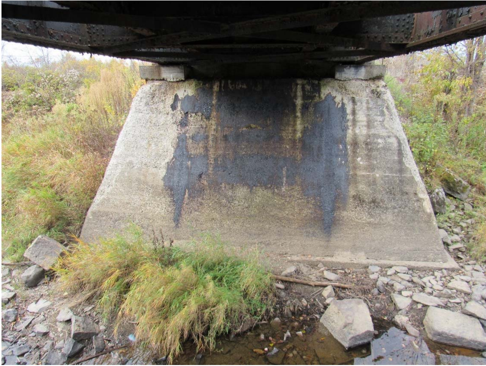
MP 139.56 – Fish River – South Abutment
