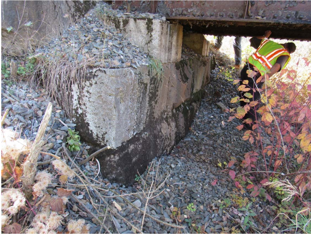
MP 167.76 – Beaver Brook – South Abutment
