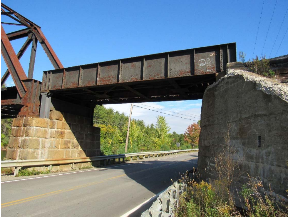
MP 113.14 – Grindstone Approach – Looking North
