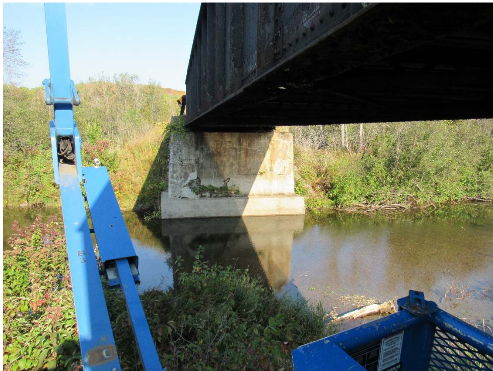
MP 236.44 – Wallagrass Stream – North Abutment
