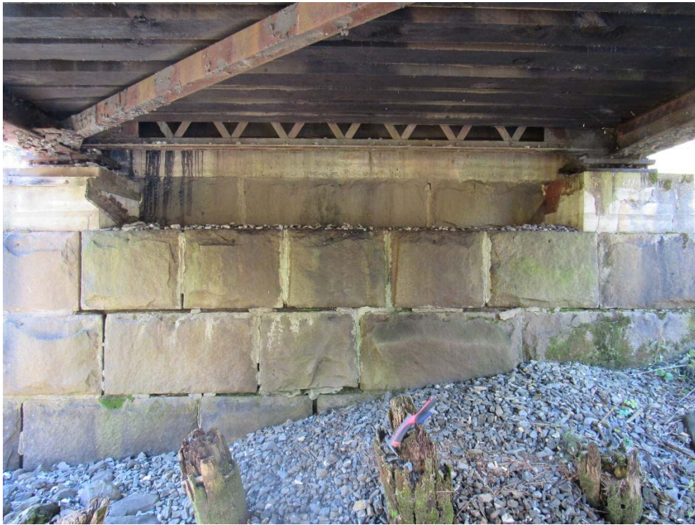
MP 185.84 – Squapan Stream – South Abutment
