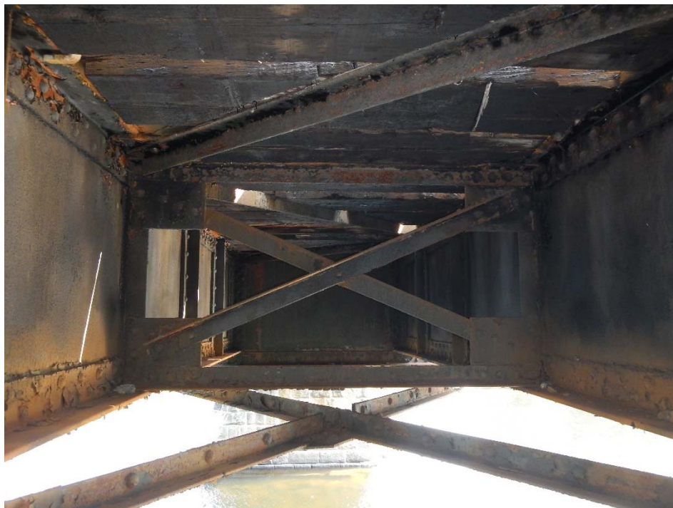
MP 113.14 – Grindstone Truss – Between Stringers
