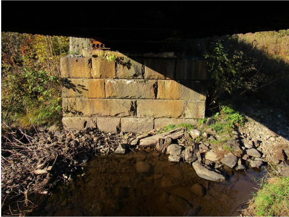
MP 179.34 – N. Branch Blackwater River – North Abutment
