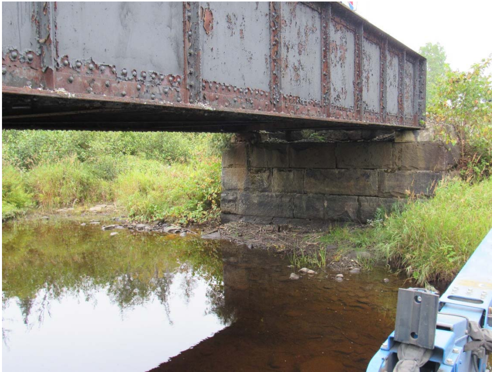
MP 164.74 – Howe Brook – South Abutment
