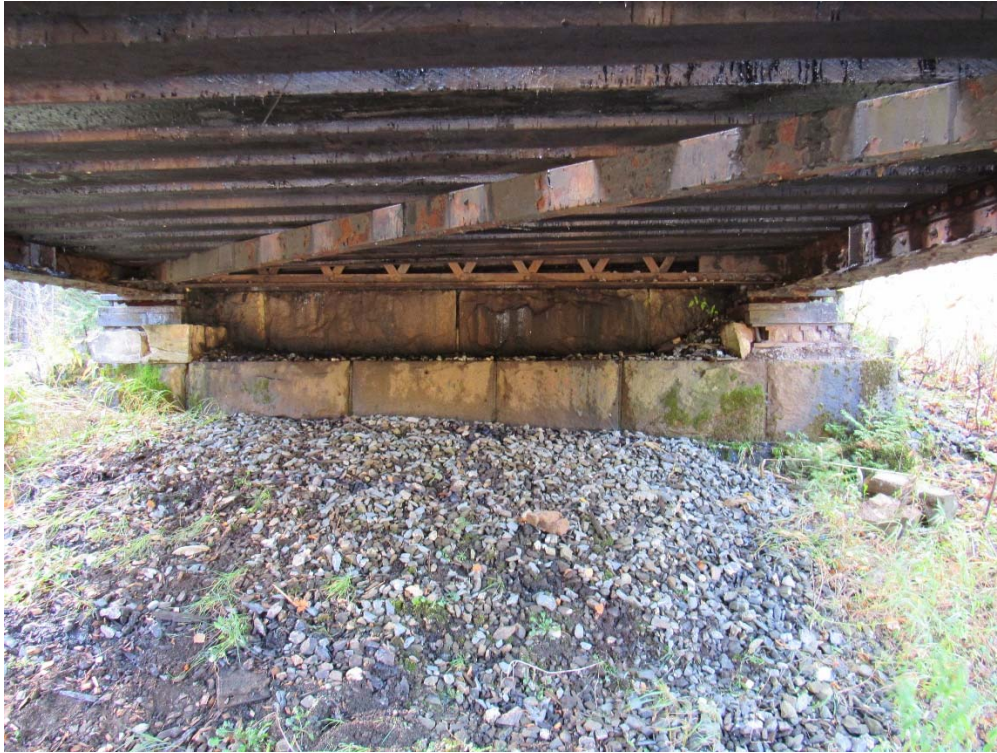
MP 161.03 – Smith Brook – South Abutment
