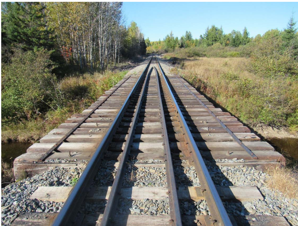
MP 179.34 – N. Branch Blackwater River – Looking North
