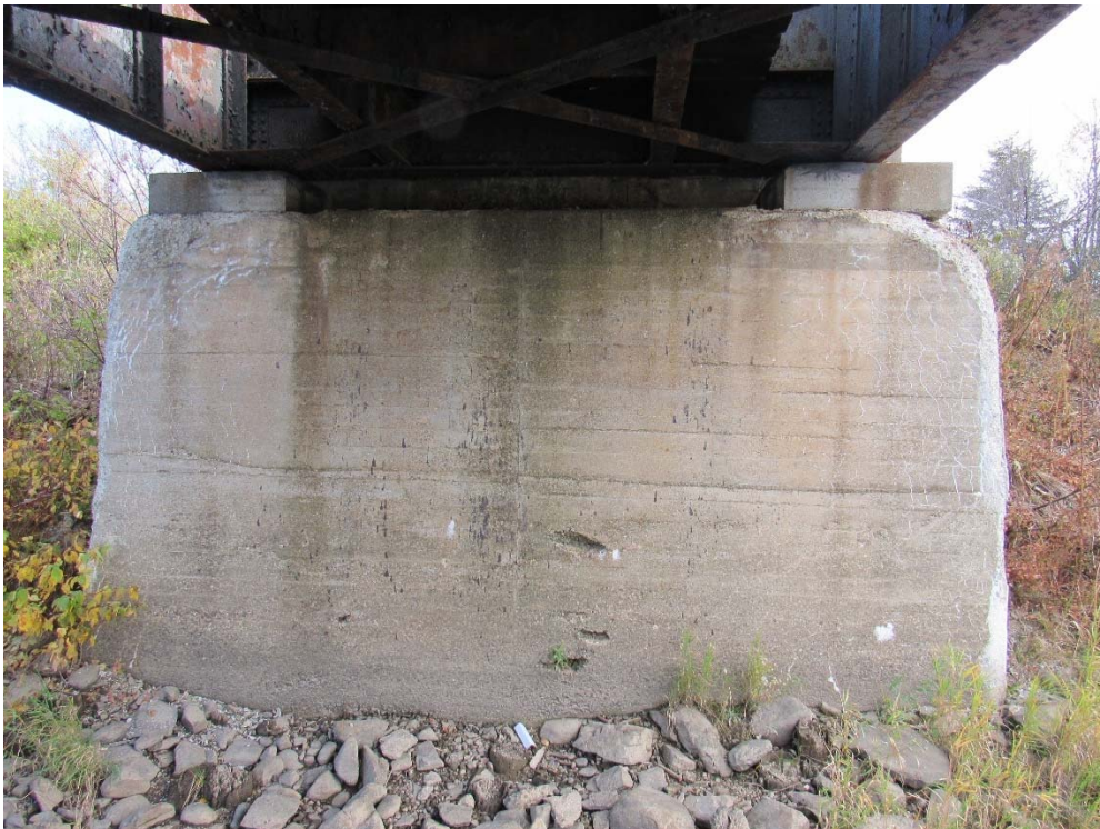
MP 139.56 – Fish River – North Abutment
