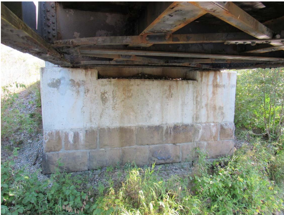
MP 139.66 – W. Branch Mattawamkeag River – North Abutment
