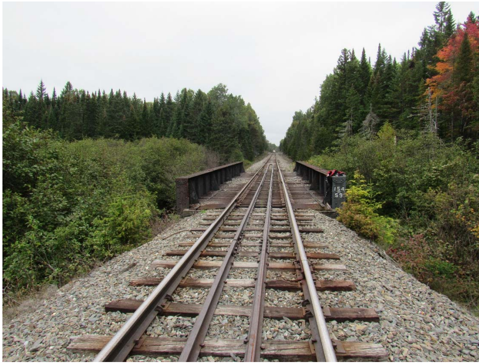
MP 154.59 – Dudley Brook – Looking South
