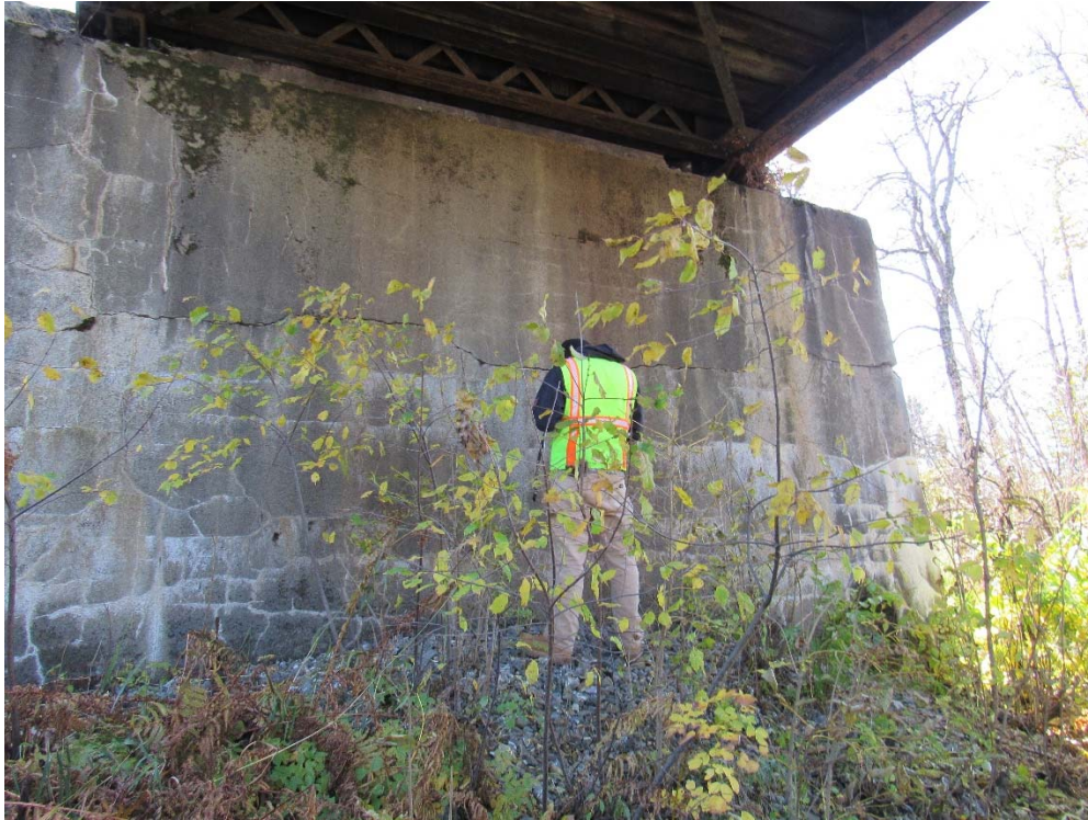
MP 236.44 – Wallagrass Stream – South Abutment
