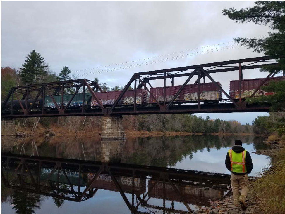
MP 113.14 – Grindstone Truss – Looking North
