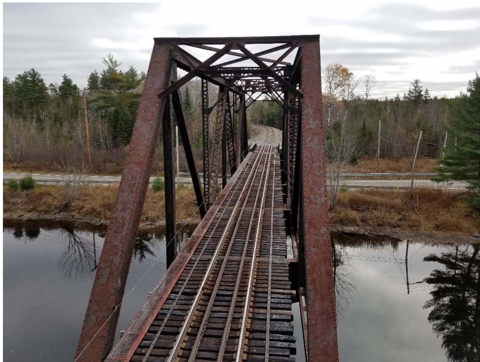
MP 113.14 – Grindstone Truss – Portal Frame
