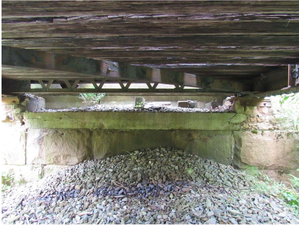
MP 154.59 – Dudley Brook – North Abutment
