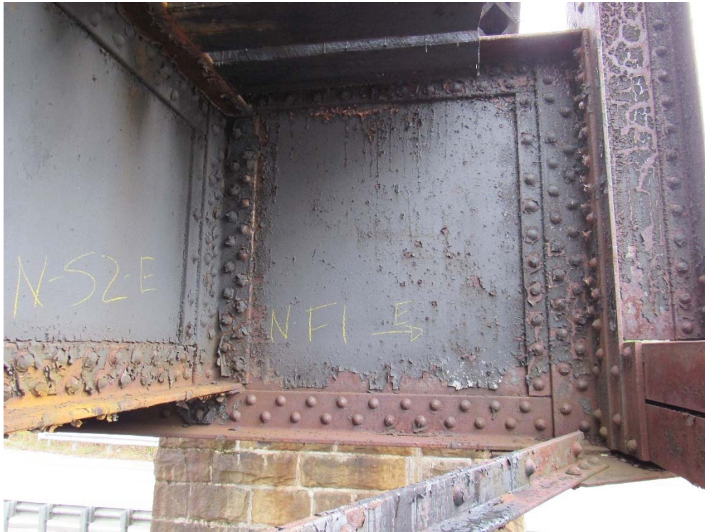
MP 113.14 – Grindstone Truss – Floorbeam and Stringer Connection
