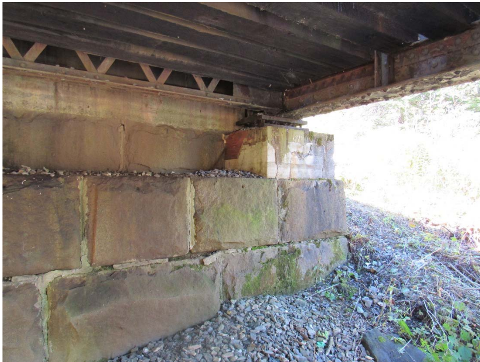
MP 185.84 – Squapan Stream – Typical Bearing Pedestal
