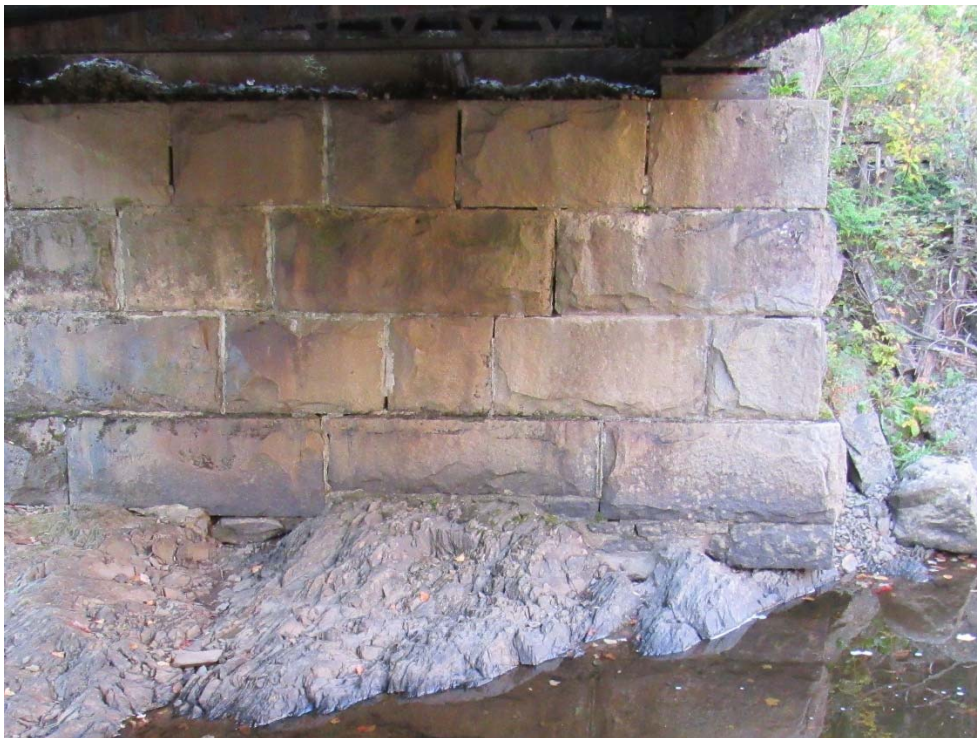
MP 151.54 – E. Branch Mattawamkeag River – South Abutment
