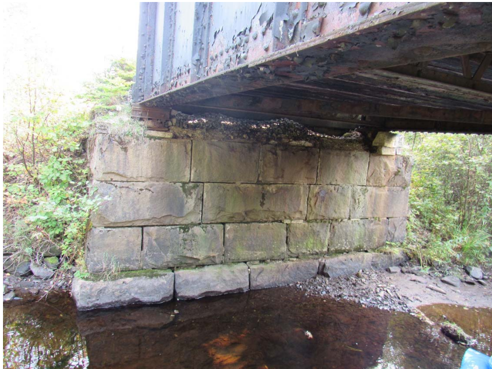
MP 154.59 – Dudley Brook – South Abutment
