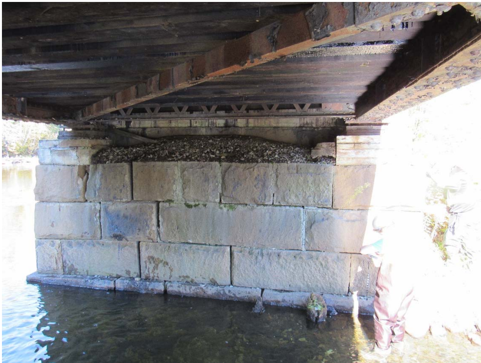
MP 185.84 – Squapan Stream – North Abutment
