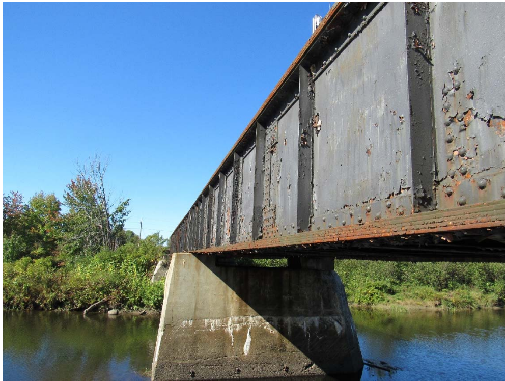
MP 139.66 – W. Branch Mattawamkeag River – East Elevation
