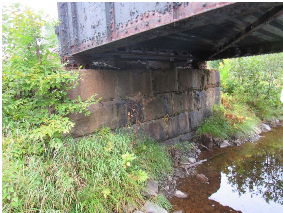
MP 164.74 – Howe Brook – North Abutment
