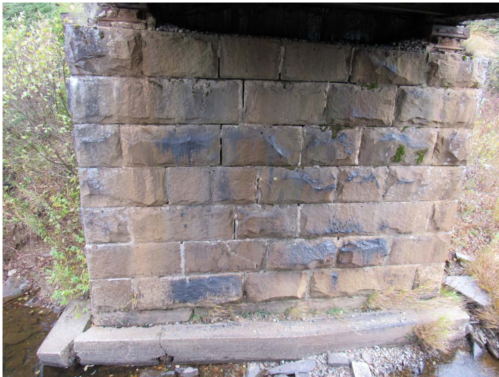
MP 161.03 – Smith Brook – North Abutment
