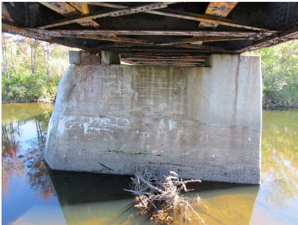
MP 139.66 – W. Branch Mattawamkeag River – Center Pier, Looking North
