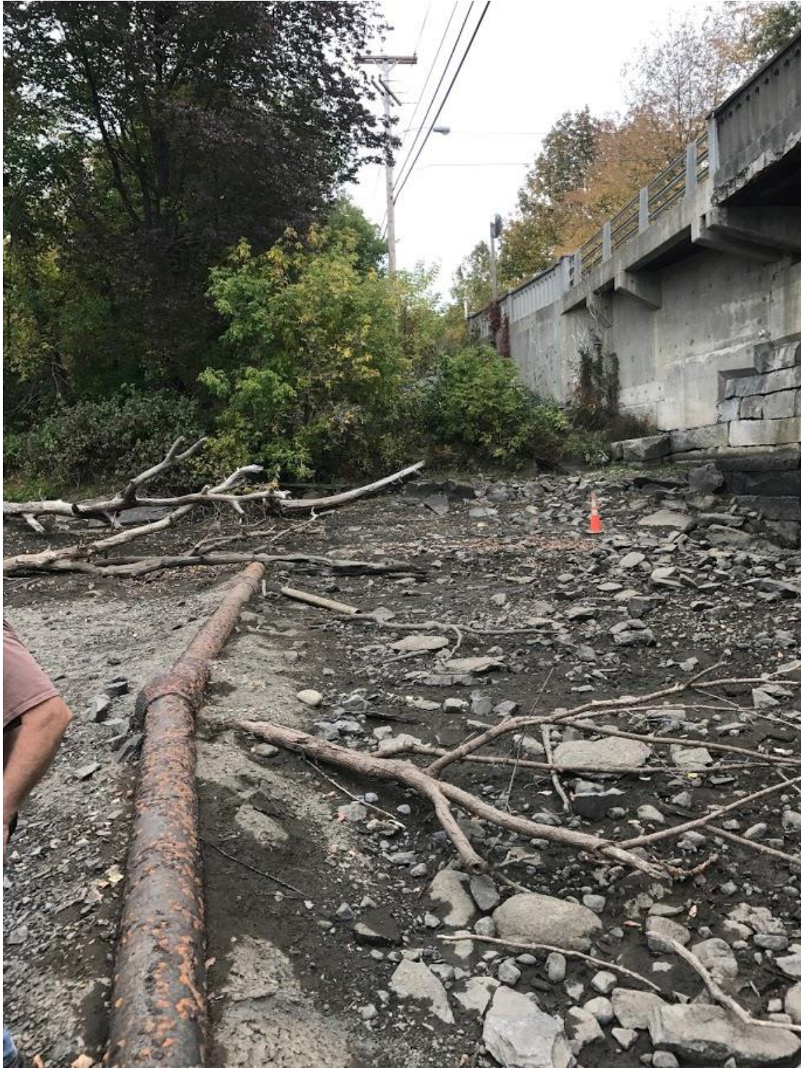
Looking Northerly at water main near northerly abutment
