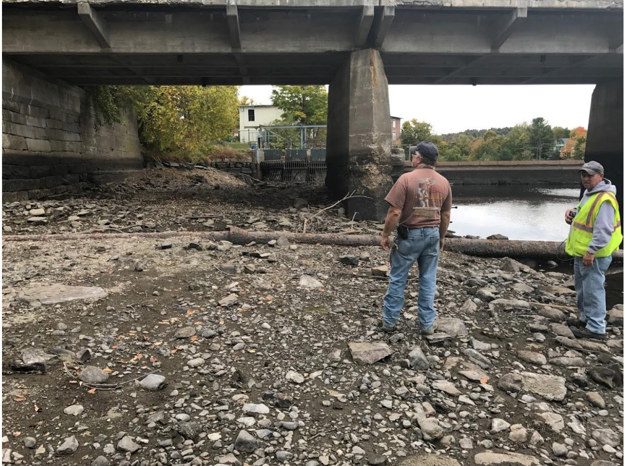
Looking downstream near northwest end of the Dover Bridge
