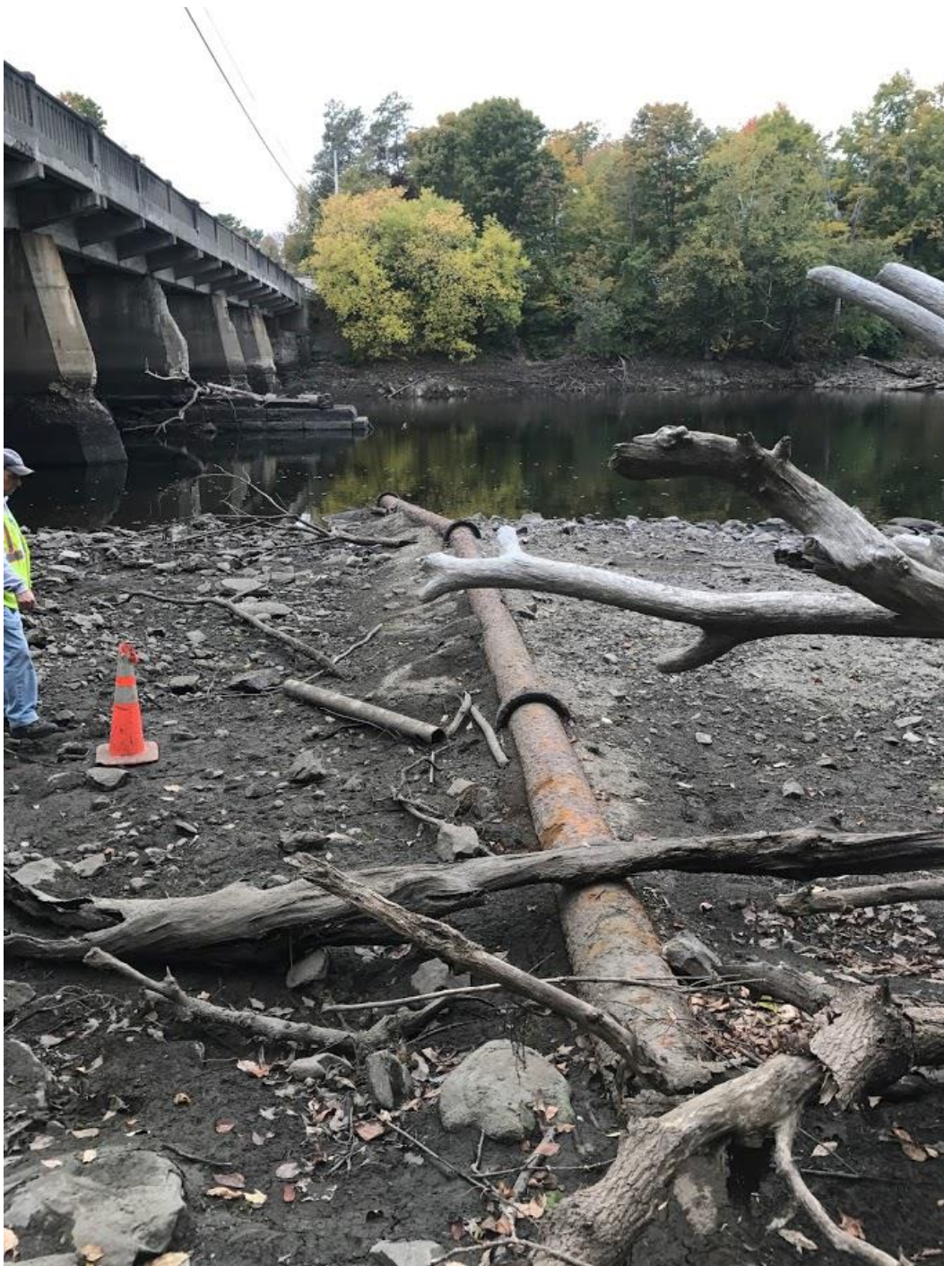
Looking West toward abutment #1 on upstream side of Dover Bridge
