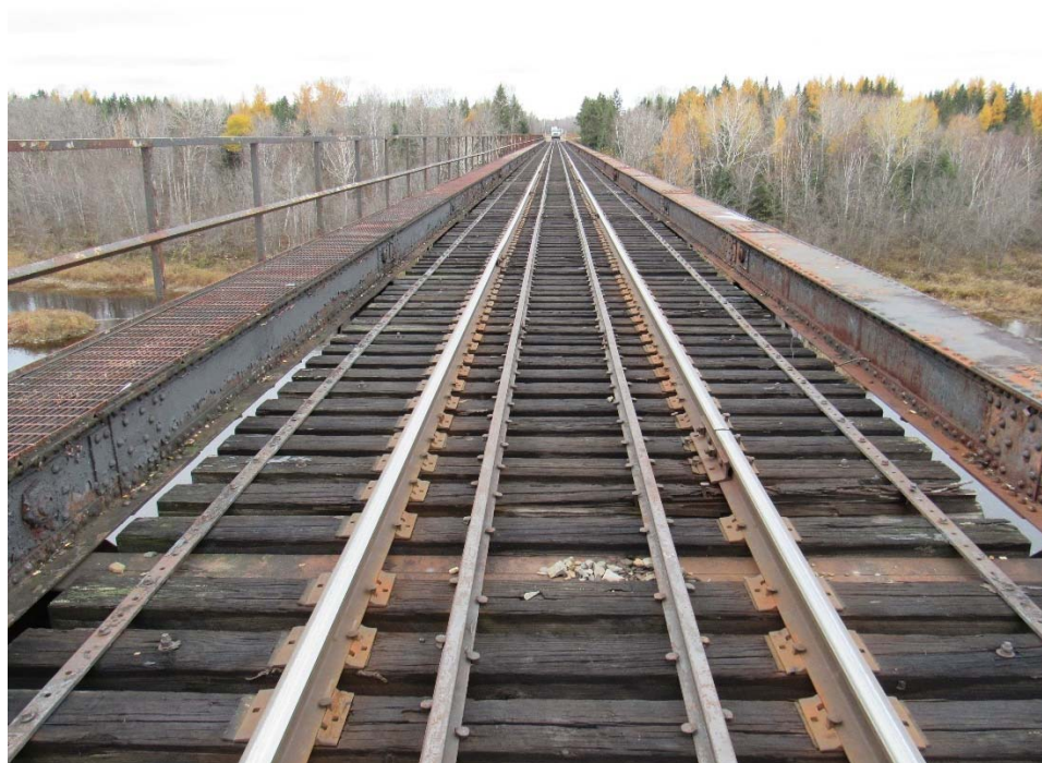
MP 193.50 – Sheridan Truss – Looking North
