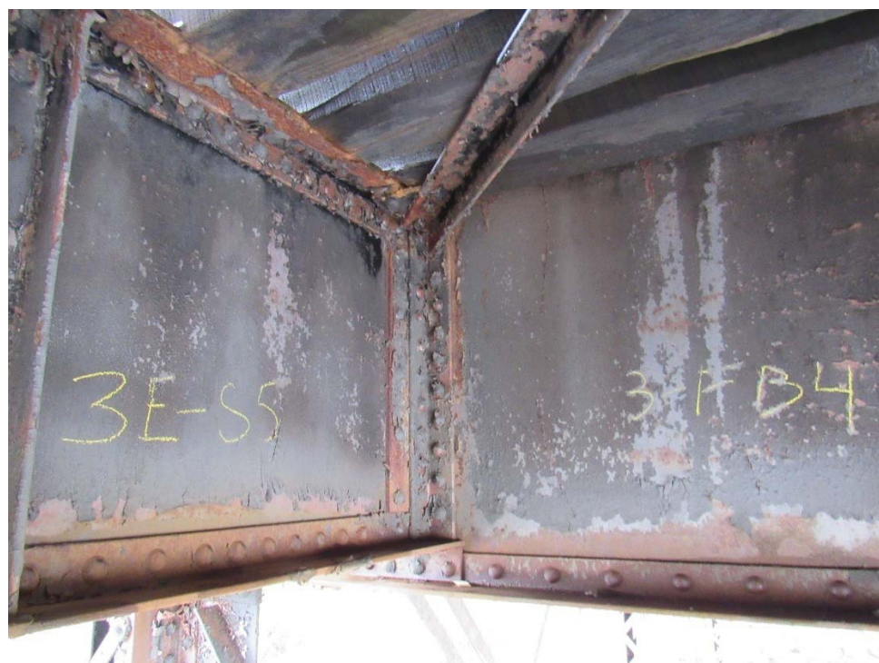
MP 193.50 – Sheridan Truss – Typical Truss Stringer Connection
