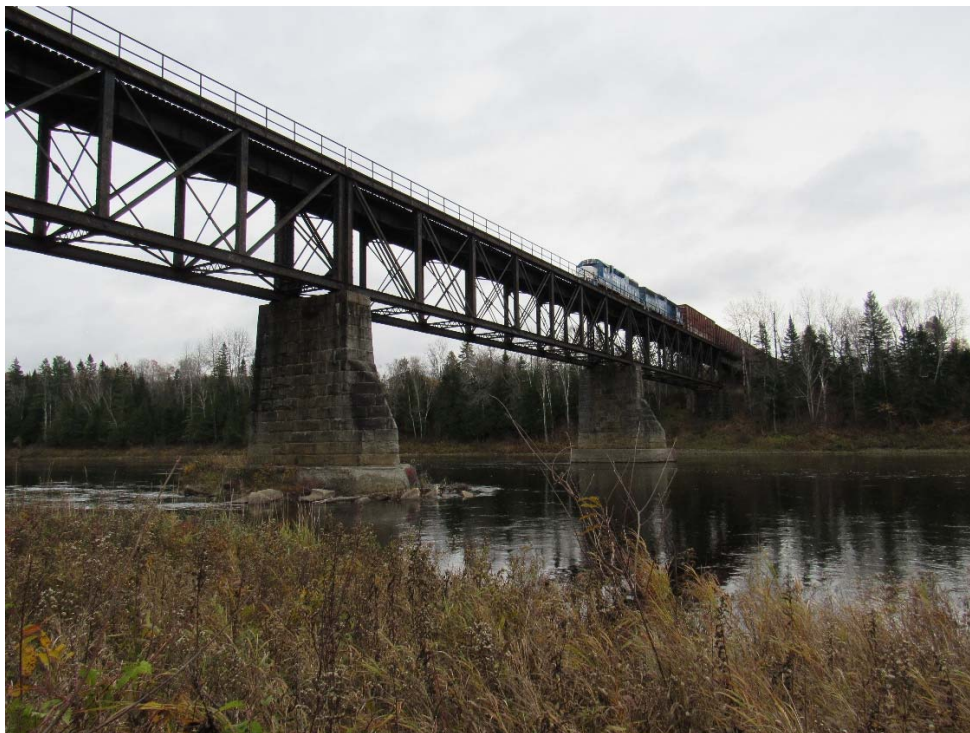
MP 193.50 – Sheridan Truss – East Elevation
