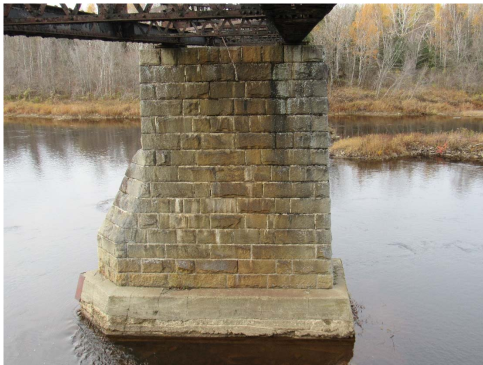
MP 193.50 – Sheridan Truss – Pier 3, South Elevation
