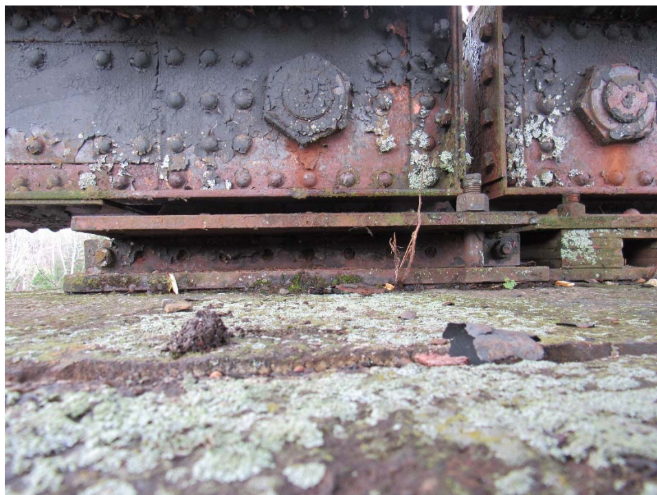
MP 193.50 – Sheridan Truss – Typical Truss Expansion Bearing
