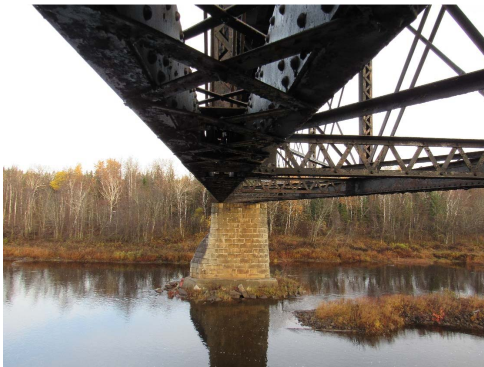
MP 193.50 – Sheridan Truss – Pier 4, North Elevation
