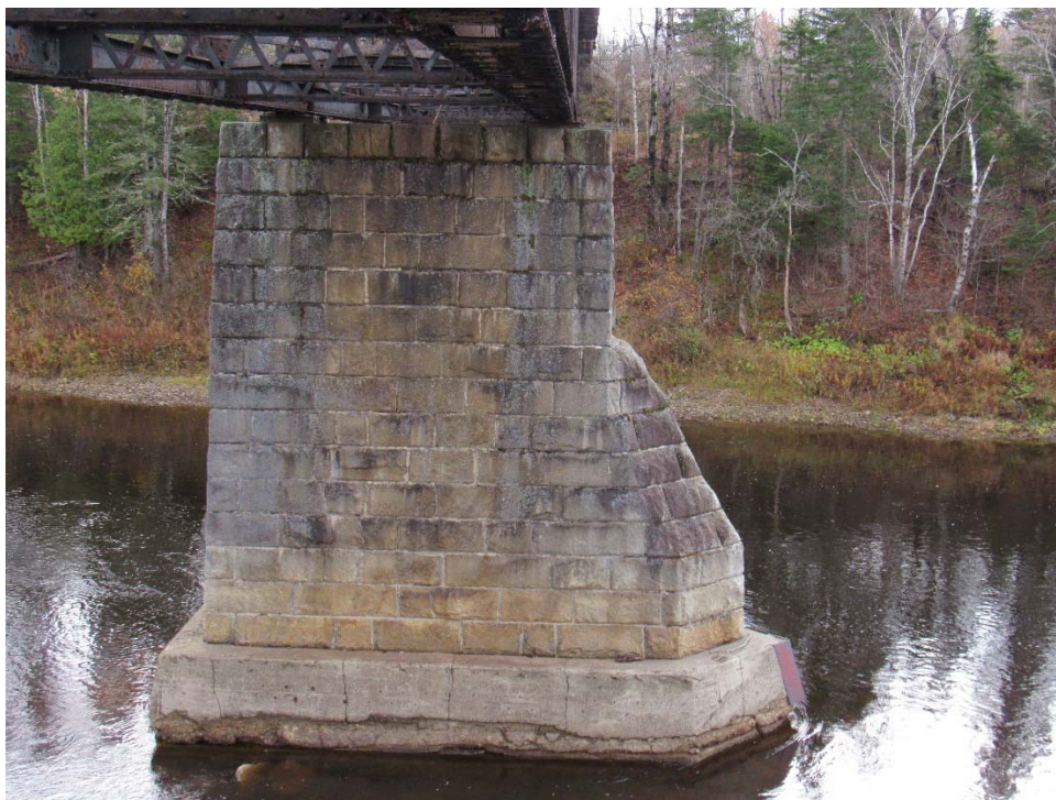
MP 193.50 – Sheridan Truss – Pier 3, North Elevation
