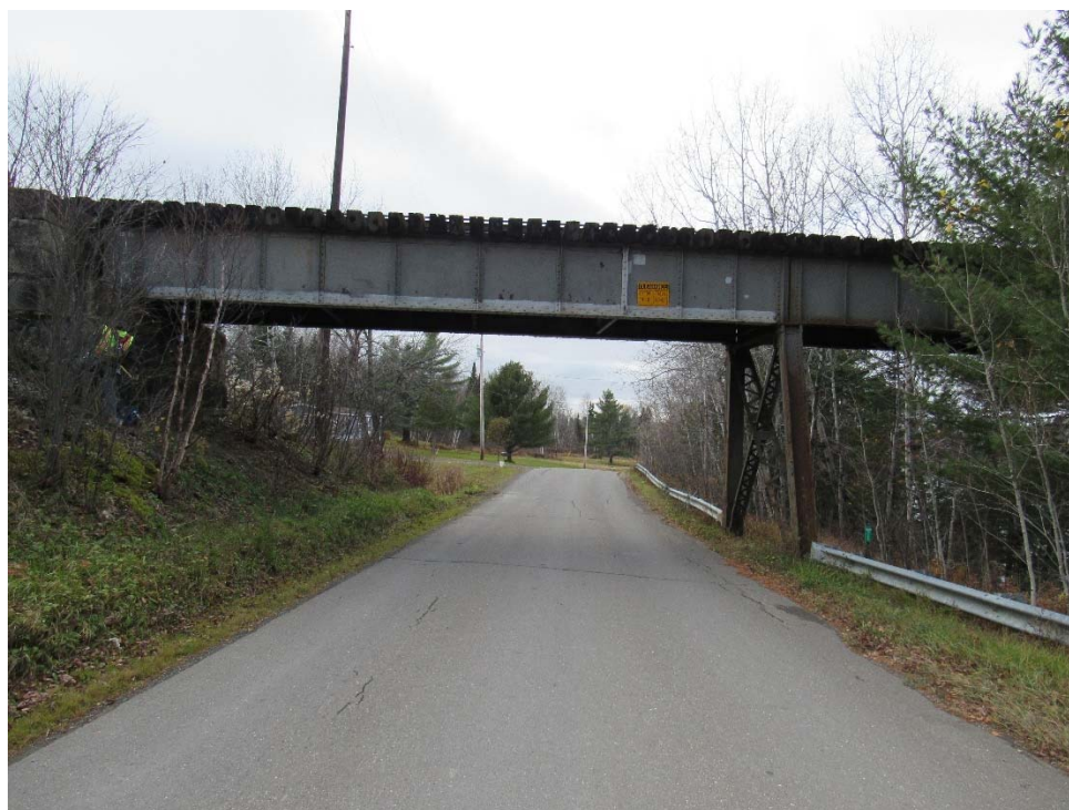
MP 193.50 – Sheridan Truss – South Approach Spans (Spans 1 & 2)
