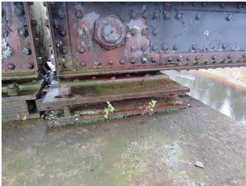
MP 193.50 – Sheridan Truss – Typical Truss Expansion Bearing
