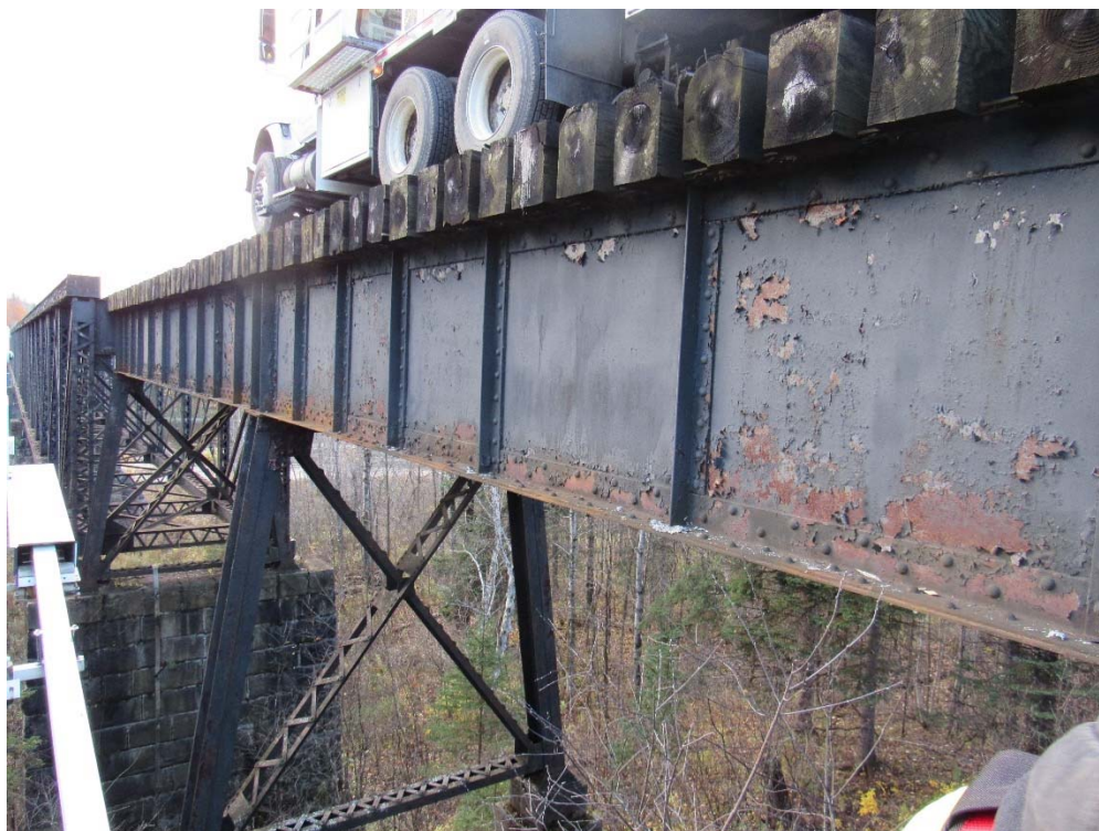
MP 193.50 – Sheridan Truss – North Approach Spans (Spans 7 & 8)
