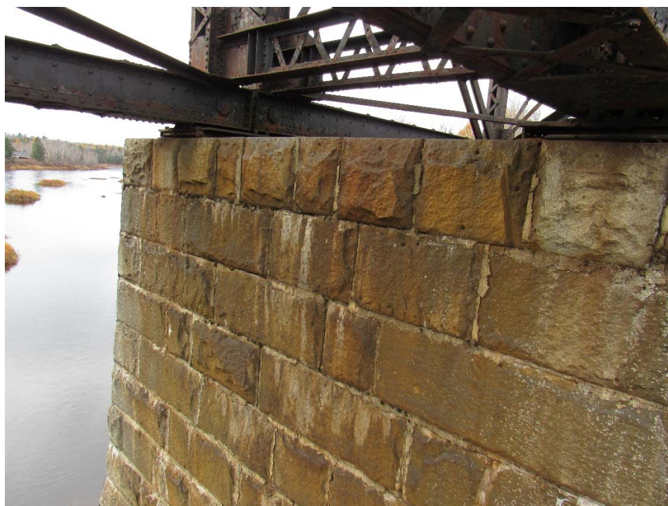
MP 193.50 – Sheridan Truss – Typical Truss Bearing and Jacking Frame
