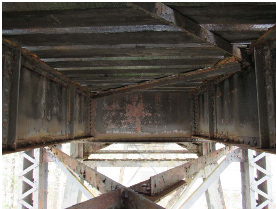
MP 193.50 – Sheridan Truss – Typical Truss Stringer Framing
