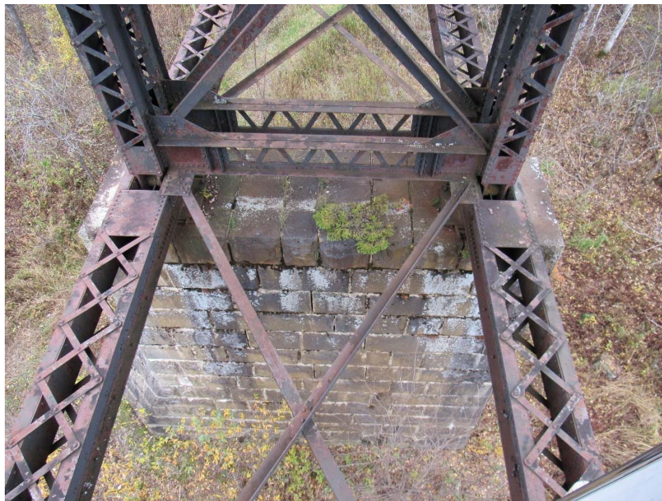
MP 193.50 – Sheridan Truss – Typical Truss Strut and Jacking Frame
