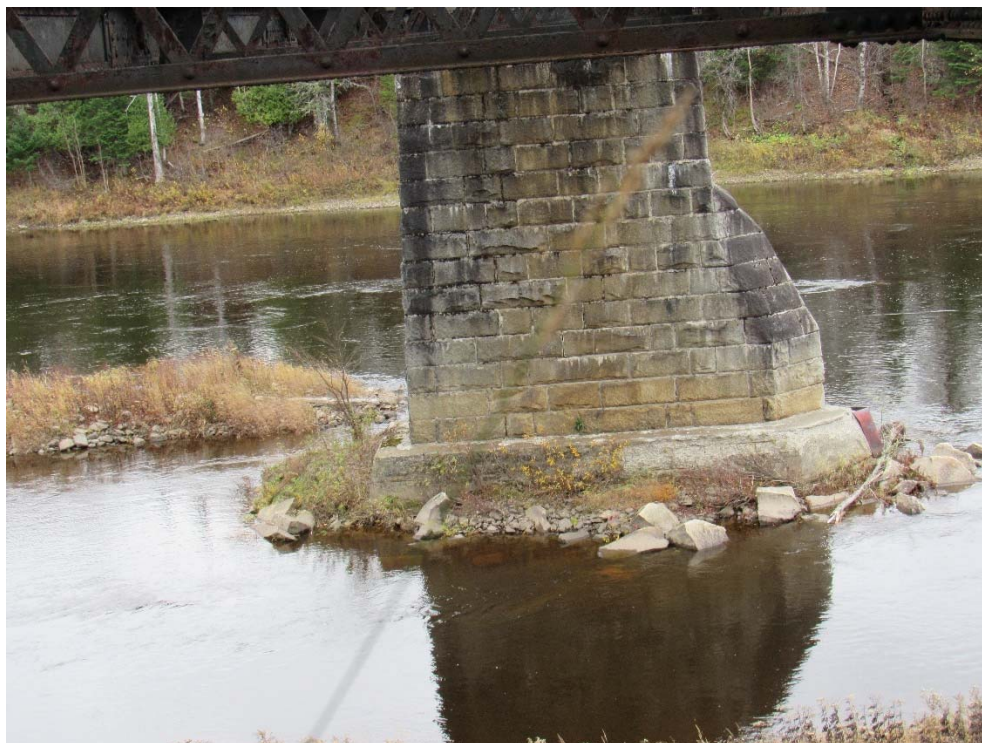
MP 193.50 – Sheridan Truss – Pier 4, South Elevation
