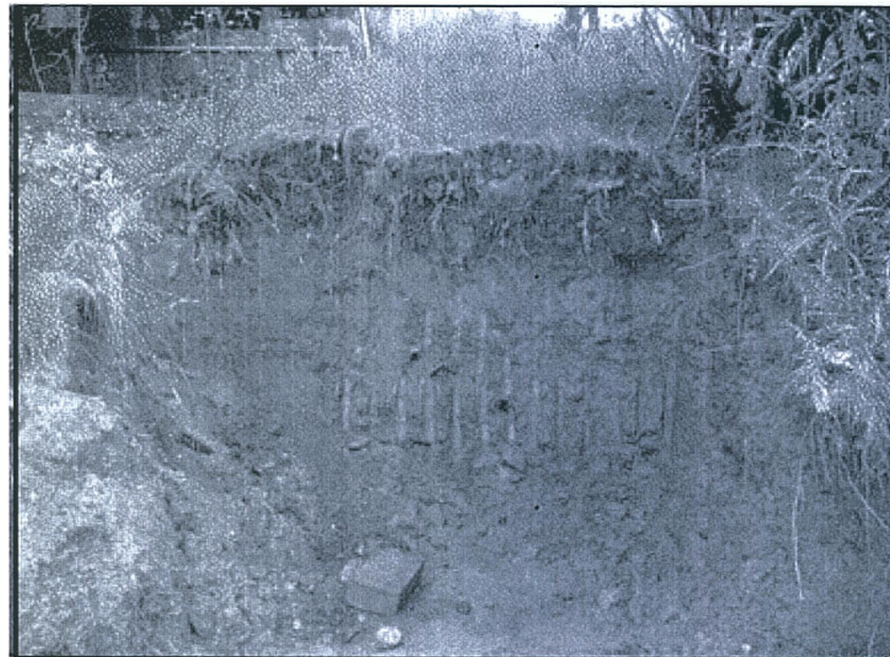
CLOSE-UP VIEW OF TEST PIT NO. 2 EXCAVATED ON THE NORTH SIDE OF THE EXISTING ROUTE 1 OVERPASS BRIDGE APPROXIMATELY ONE WEEK AFTER EXCAVATION, LOOKING EAST, 30 JUNE 2011.
