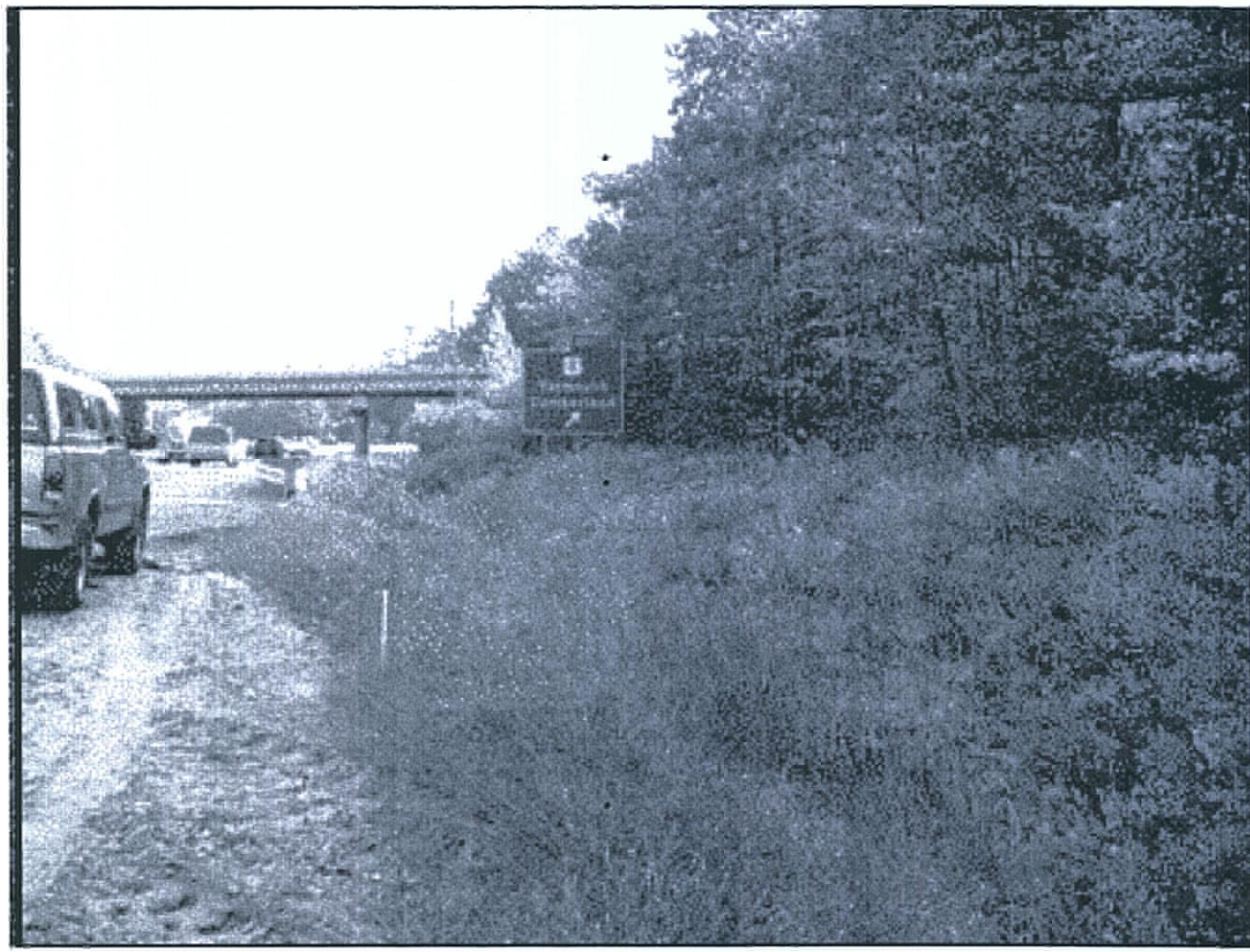
VIEW OF I-295 NB DECELERATION LANE BENEATH THE EXISTING ROUTE 1 OVERPASS BRIDGE WITH PIER NO. 1 (LEFT) VISIBLE, LOOKING NORTH.
