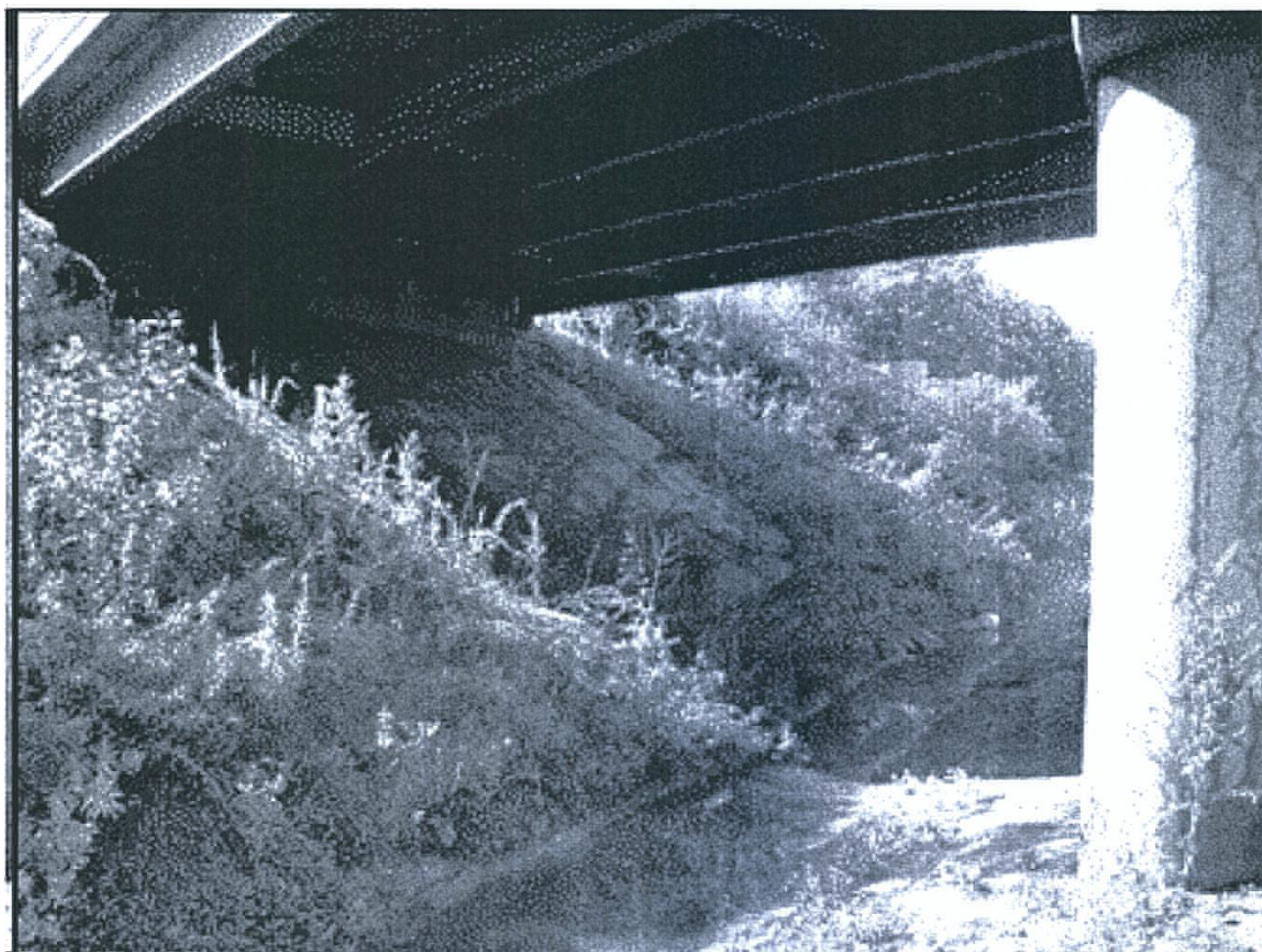
VIEW OF CONCRETE PAVER SLOPE PROTECTION BENEATH THE EXISTING ROUTE 1 OVERPASS BRIDGE WITH ABUTMENT A (LEFT) AND PIER NO. 1 (RIGHT) VISIBLE, LOOKING SOUTHEAST.
