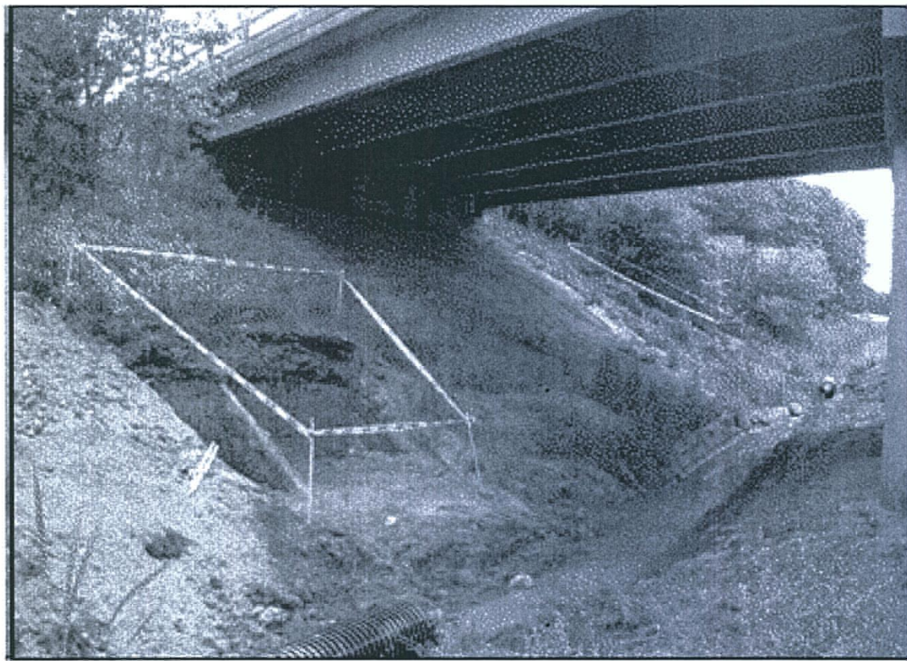
VIEW OF I-295 NB DECELERATION LANE BENEATH THE EXISTING ROUTE 1 OVERPASS BRIDGE WITH PIER NO. 1 (LEFT) VISIBLE, LOOKING NORTH.
