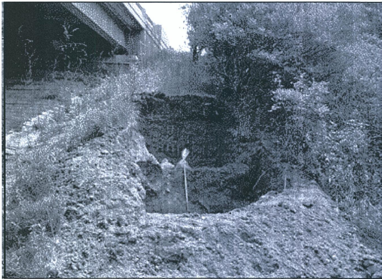
VIEW OF TEST PIT NO. 2 EXCAVATED ON THE SOUTH SIDE OF THE EXISTING ROUTE 1 OVERPASS BRIDGE IMMEDIATELY AFTER EXCAVATION, LOOKING EAST, 20 JUNE 2011.
