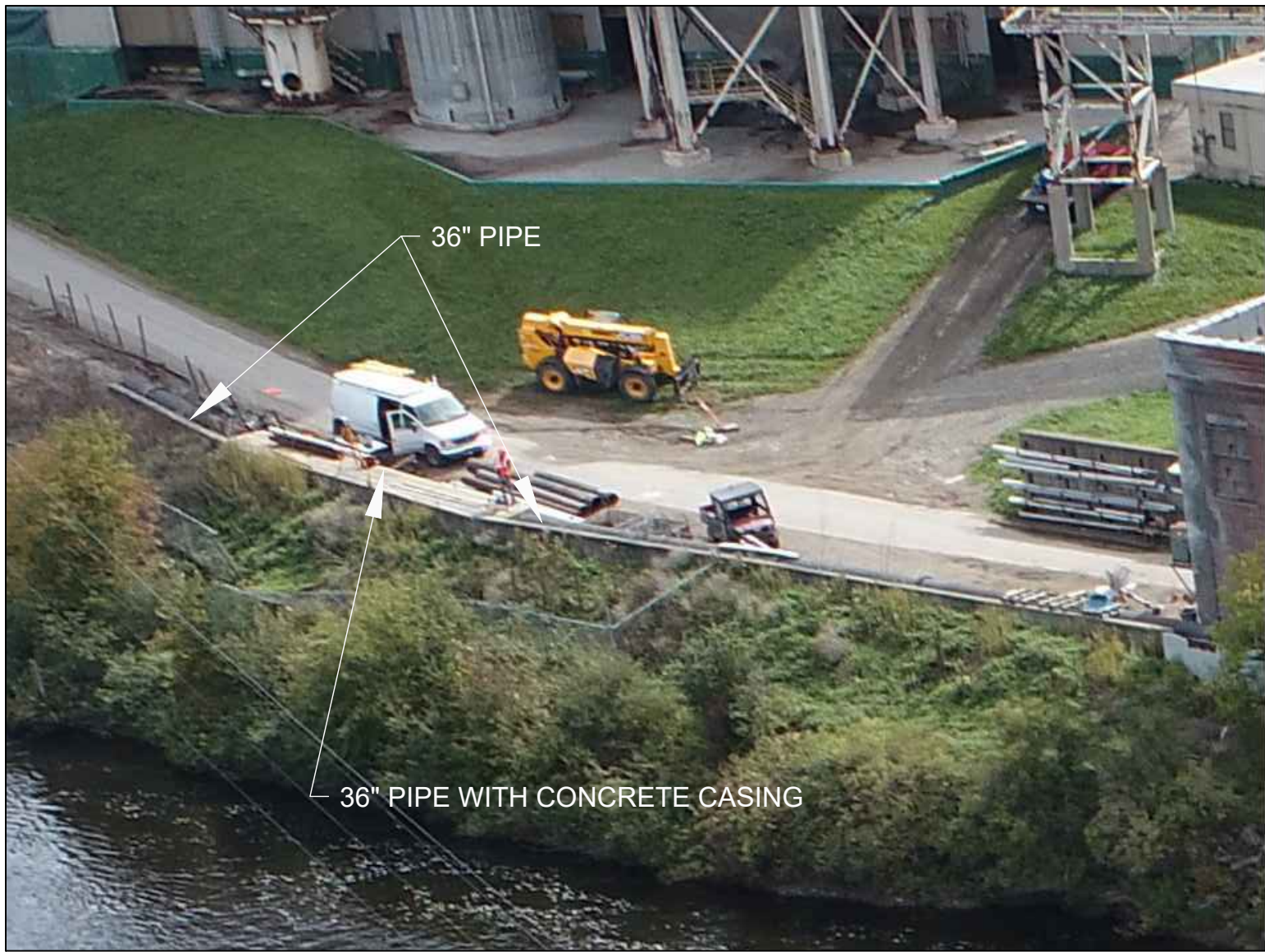
5 36" PIPE WITH CONCRETE CASING G-100 SCALE: NTS
