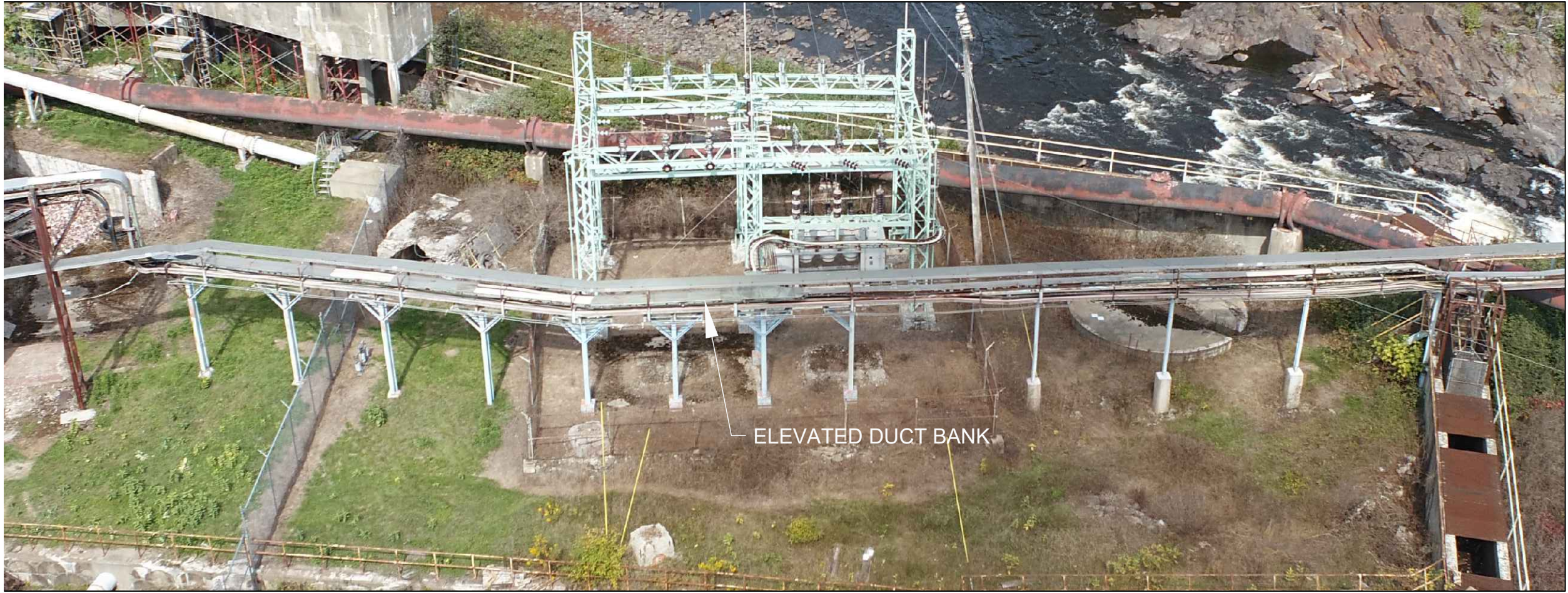
2 ELEVATED DUCT BANK G-100 SCALE: NTS
