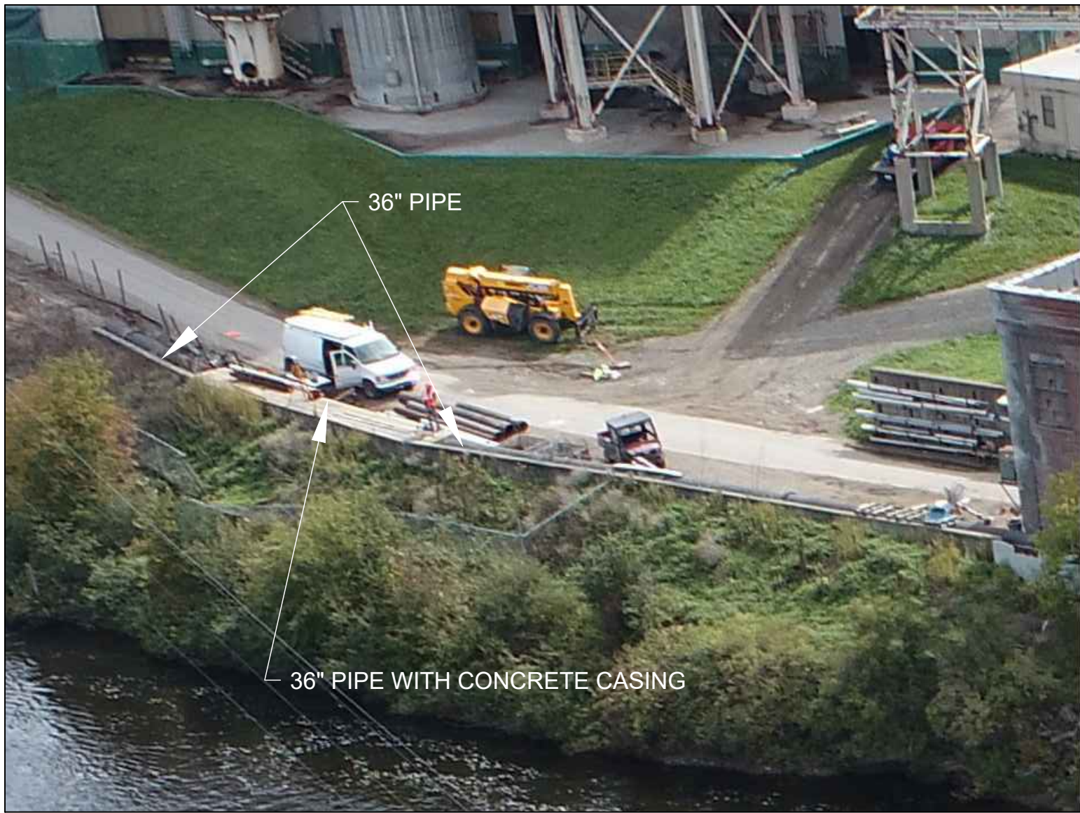
5 36" PIPE WITH CONCRETE CASING G-100 SCALE: NTS
