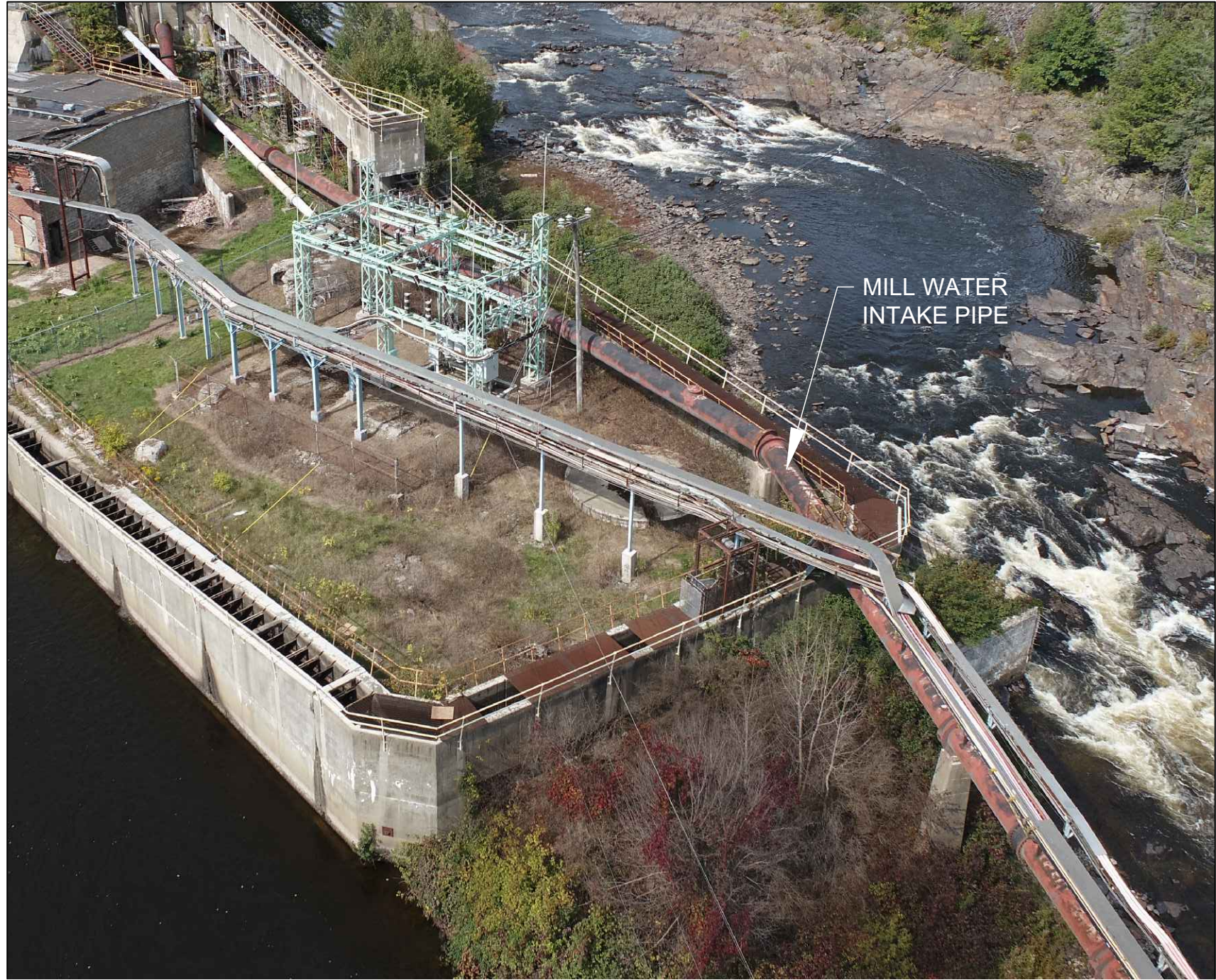
4 MILL WATER INTAKE PIPE G-100 SCALE: NTS
