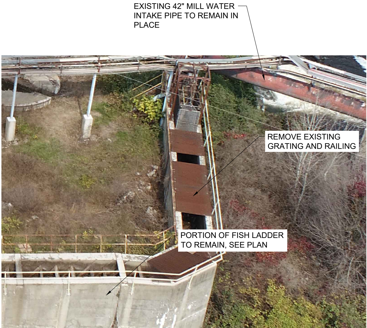
2 EXISTING FISH LADDER AND GRATING D-100 SCALE: NTS
