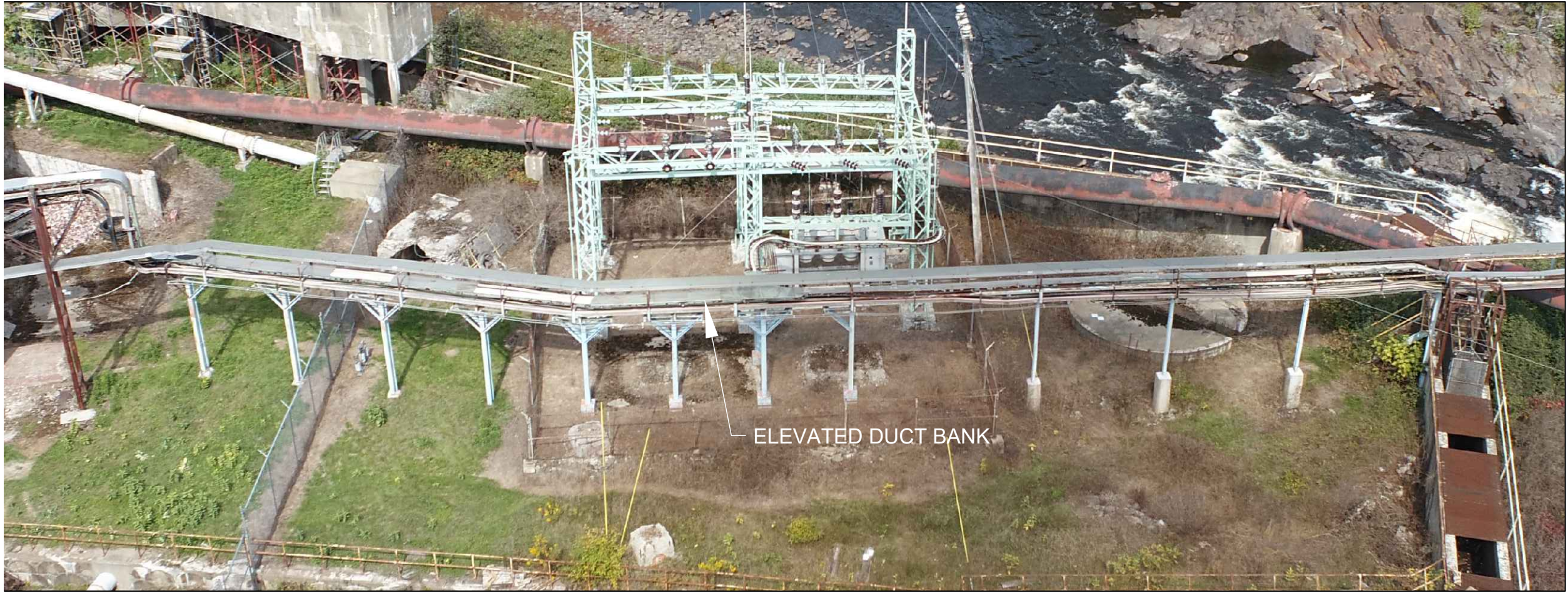
2 ELEVATED DUCT BANK G-100 SCALE: NTS
