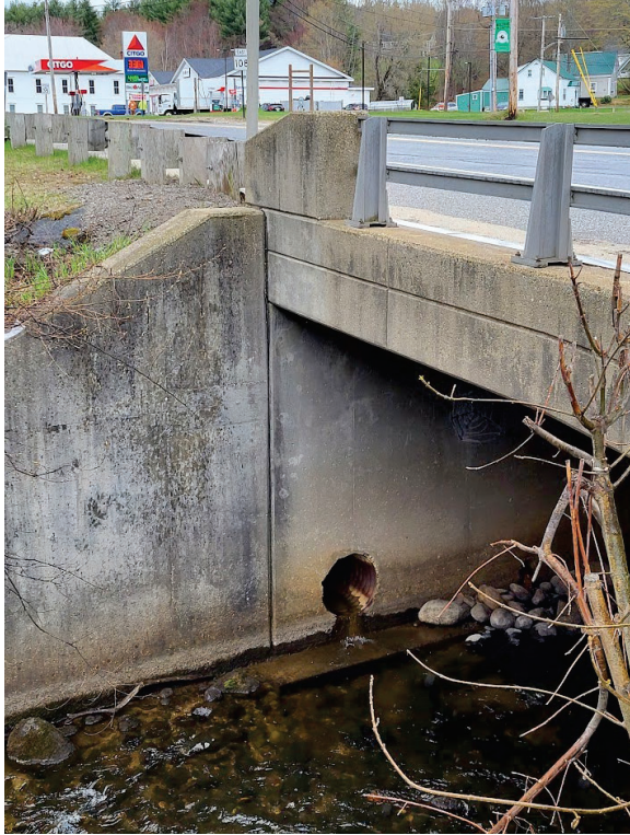
Stormwater outfall pipe along Bridge #2799 wall.
