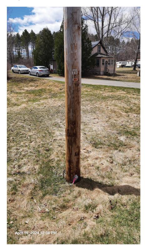
Nail assumed 100-ft elevation in profile survey
