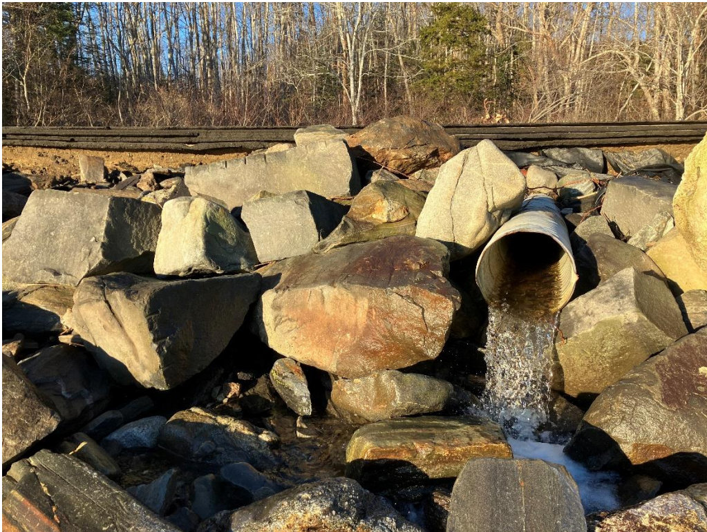
Functioning culvert outlet
