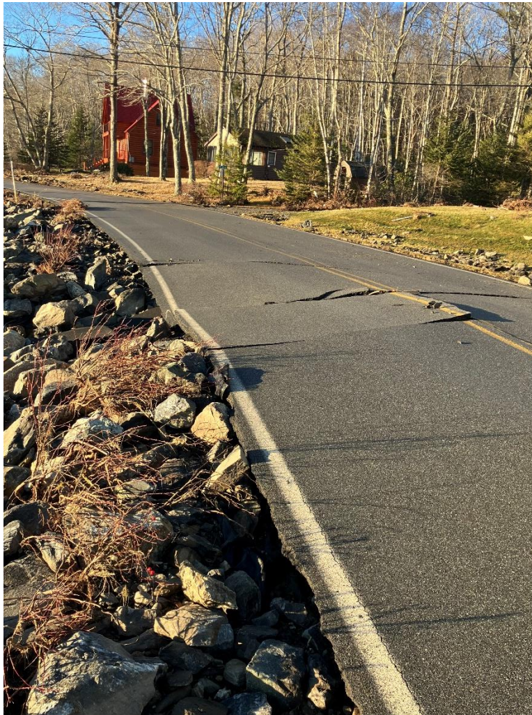
Pavement collapse
