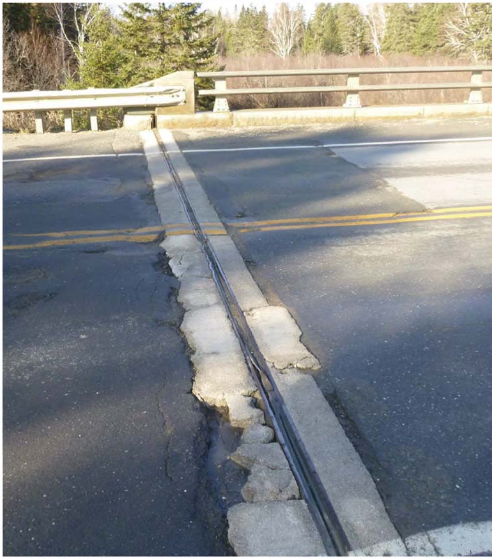
EXISTING BRIDGE JOINT - TYPICAL CONDITION BOTH ABUTMENTS
