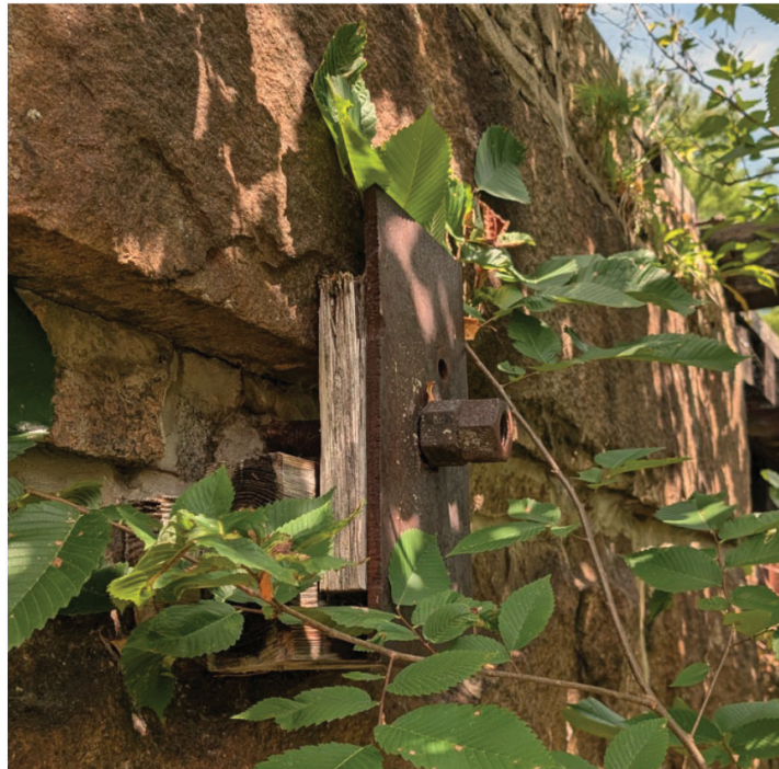
Image 1 – Existing Masonry Tie
