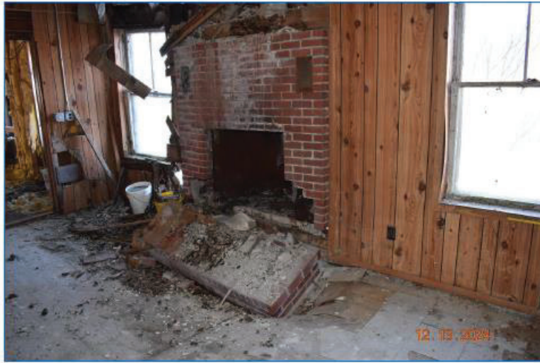
Close up fireplace and detached mantel.
