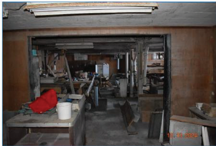
Basement workshop area
