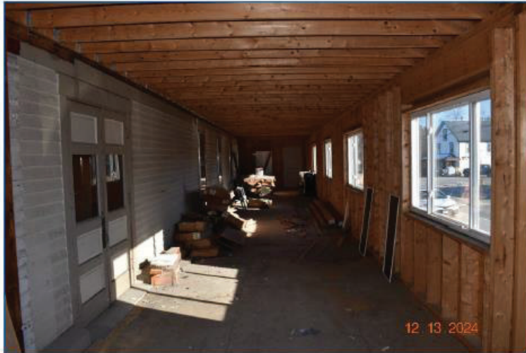
Rebuilt front porch.
