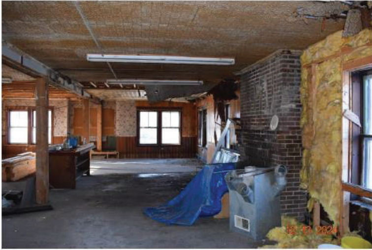
Looking west along north wall 2 nd fireplace
