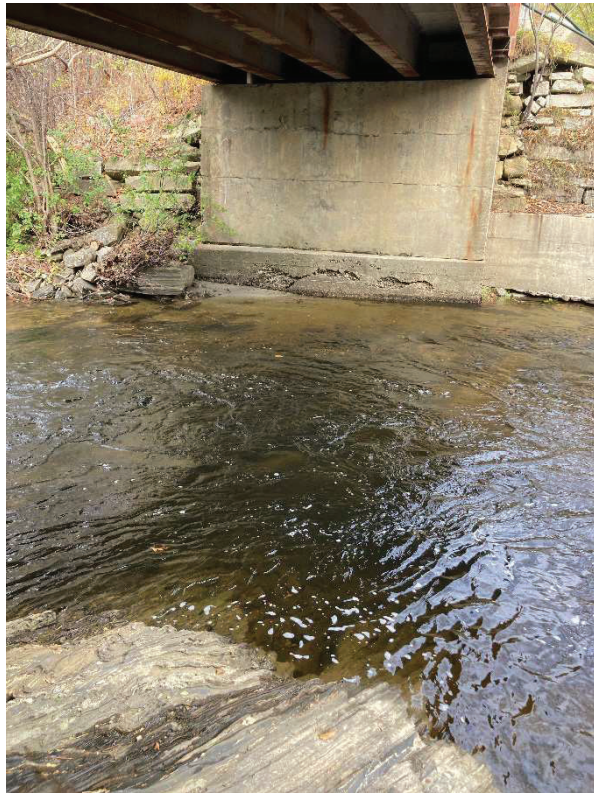
Top: view downstream showing the abutment on the south end of the bridge; Bottom: view of the abutment on the north end of the bridge.
