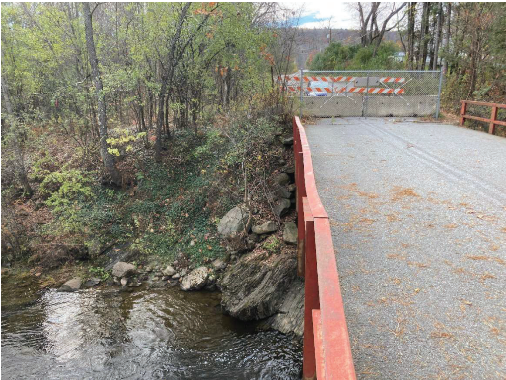
Top: view toward the north end of the bridge showing upstream/river left bank; Bottom: view toward the south end of the bridge showing downstream/river right bank.
