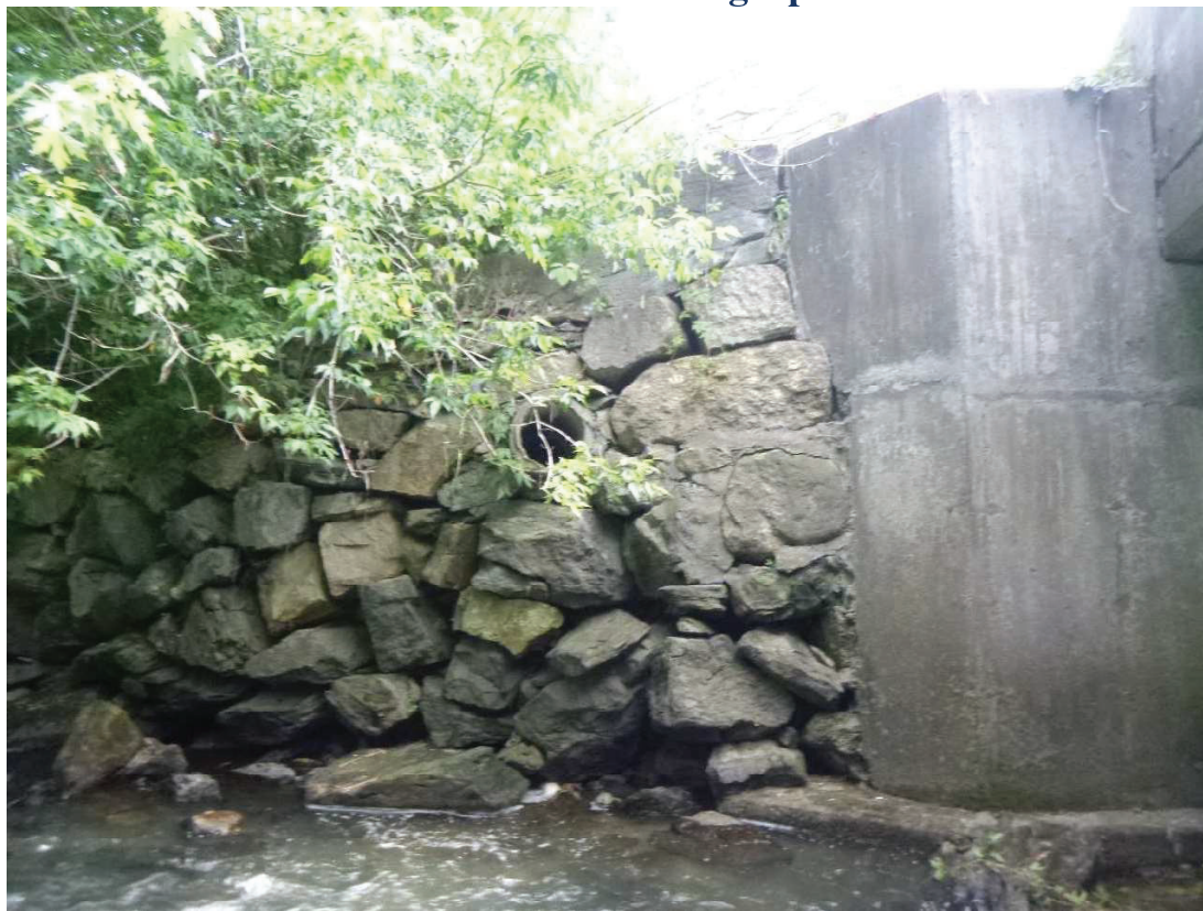
Outfall to be abandoned and flow filled
