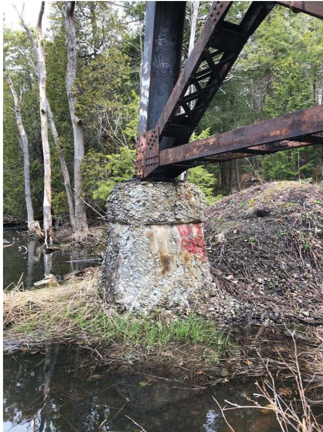
Photo 2. View of northern bent footing at spring high water. MaineDOT, April 28, 2020
