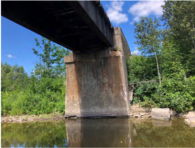
Photo 1. View of northwest abutment and adjacent wetlands at N Br. Presque Isle Stream Br. 7804. MaineDOT, July 29, 2020.
