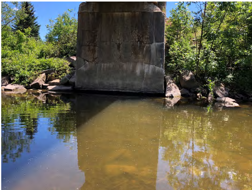
Photo 2. View of southeast abutment and adjacent wetlands at N. Br. Presque Isle Stream Br. 7805. MaineDOT, July ,29 2020
