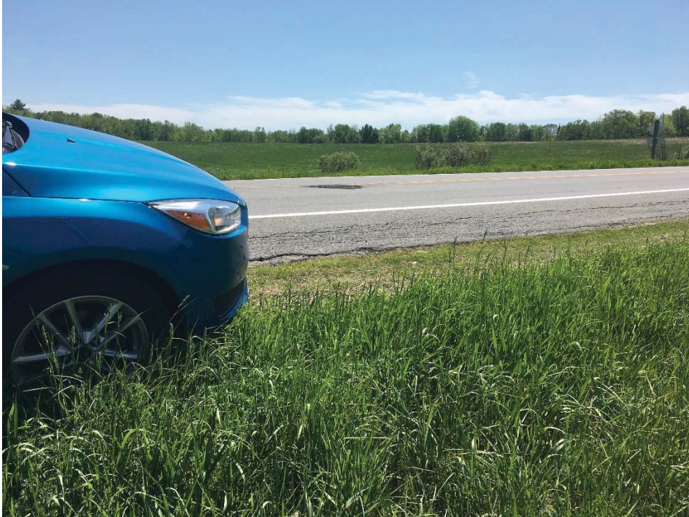
Photo 5. Patched sink hole in the road.
