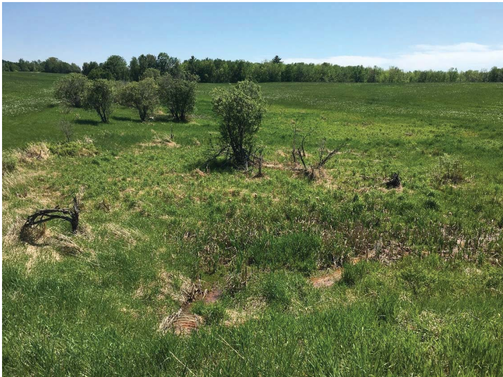
Photo 2. Culvert inlet and wetland above inlet.
