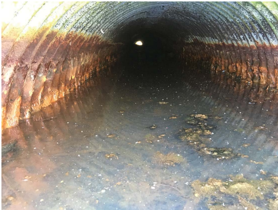
Photo 6. View up culvert from outlet.
