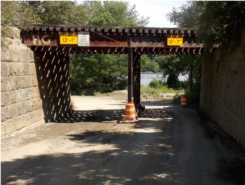
Railroad bridge at easterly end of Dutton Street in Bangor
