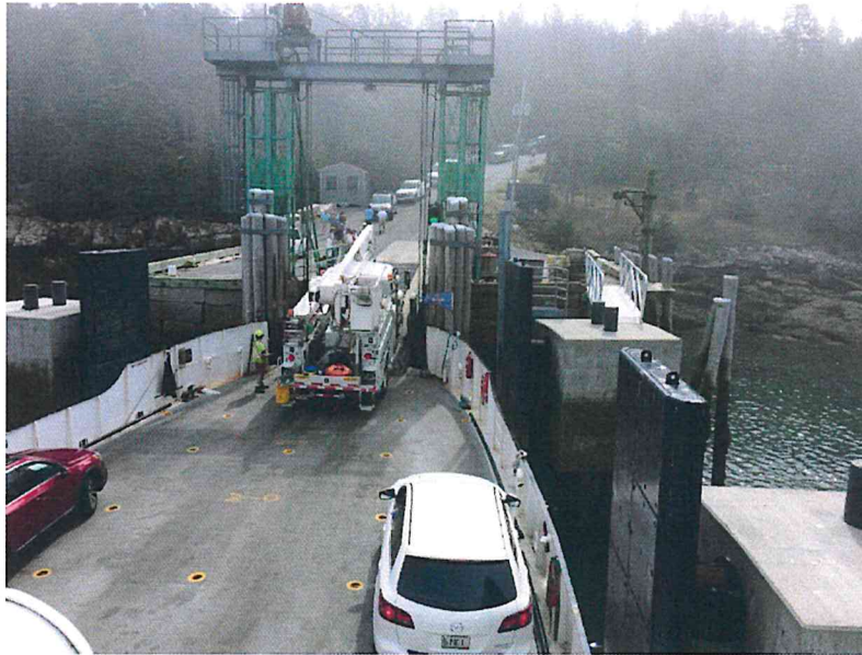
Photo 5. View of 2014 dolphins at ferry terminal, facing east. MaineDOT, August 2018.
