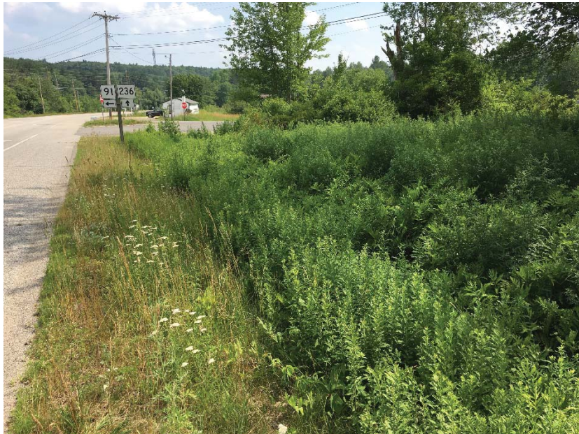
Photo 4. Emergent wetland swale along west side of Route 236 and Old South Road, facing south. Impacts in this area a result of intersection reconstruction. MaineDOT, July 5, 2018
