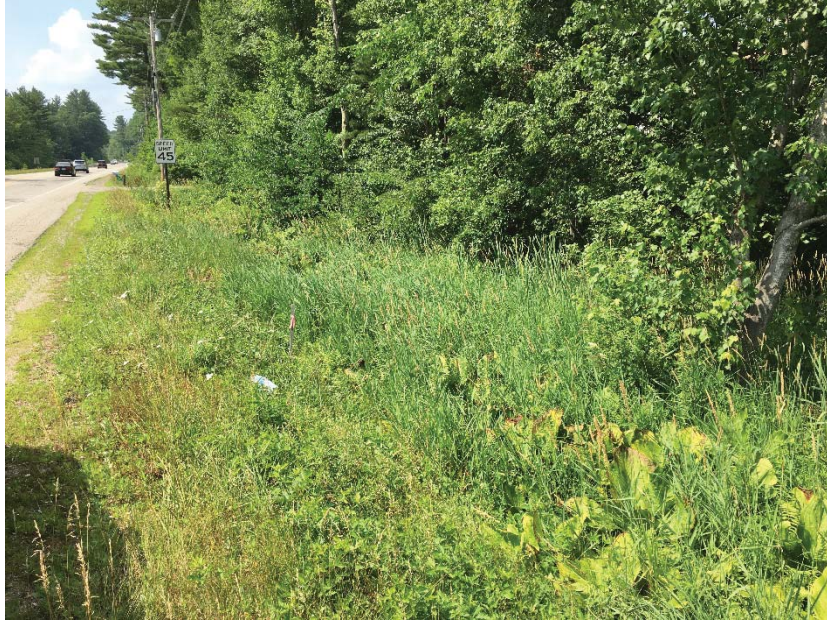
Photo 3. Emergent wetland swale along east side of Route 236, facing north. Impacts in this area a result of shoulder reconstruction and driveway cross pipe replacement. MaineDOT, July 5, 2018
