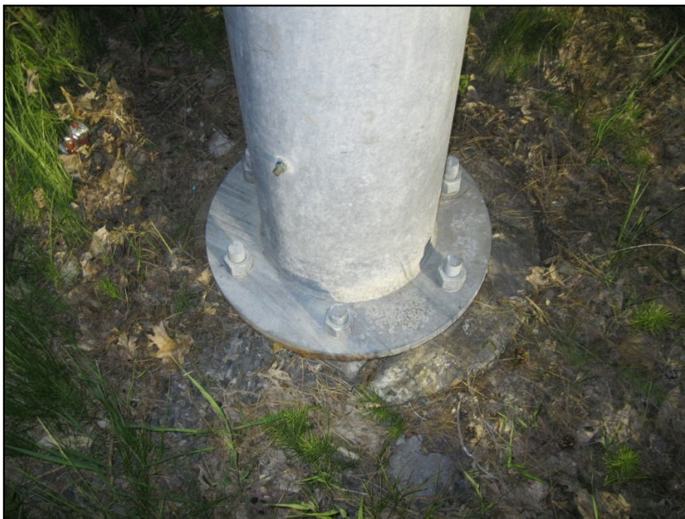
5 General view of west foundation, looking east down.
