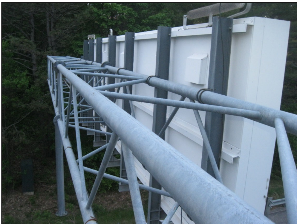
10 Truss chords and struts, looking northwest.
