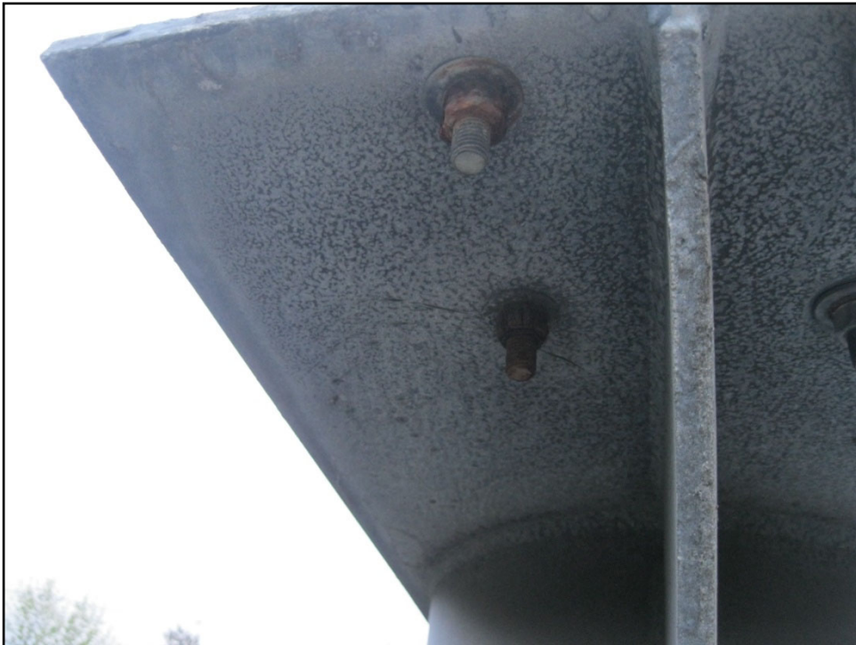
9 North lower chord saddle northeast, looking south up.
