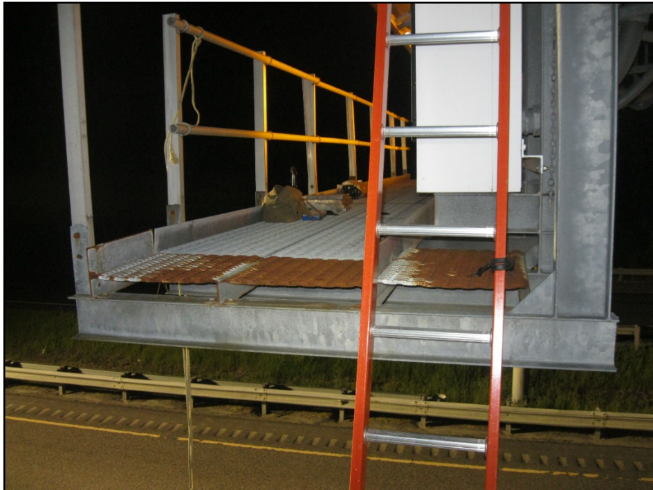
13 General view of catwalk, looking east.
