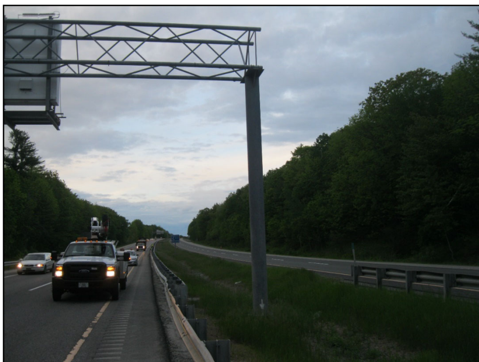
4 General view of east tower, looking north.
