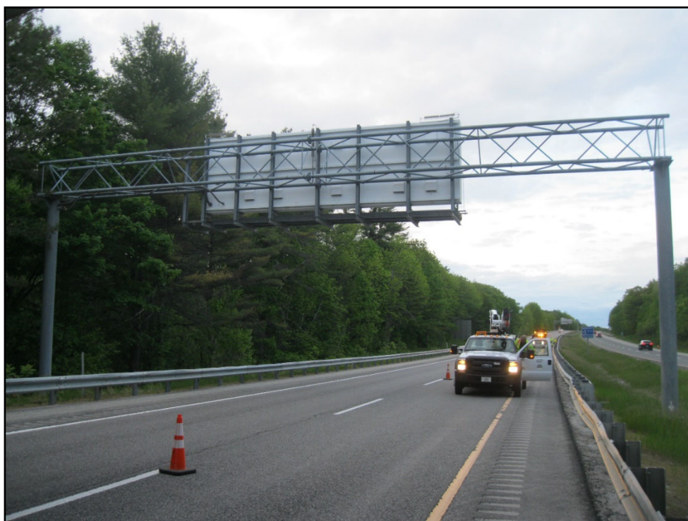
2 General view of back side of structure, looking north.
