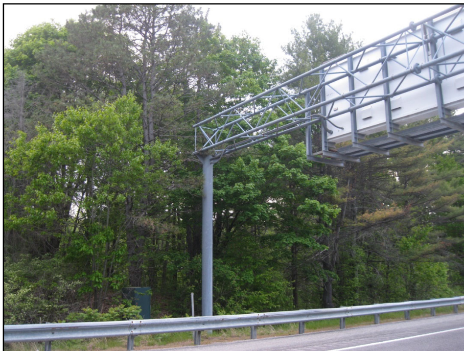
3 General view of west tower, looking northwest.
