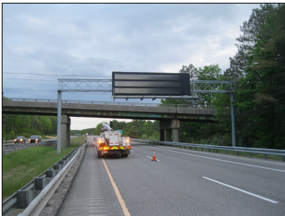
1 General view of front face of structure, looking south.
