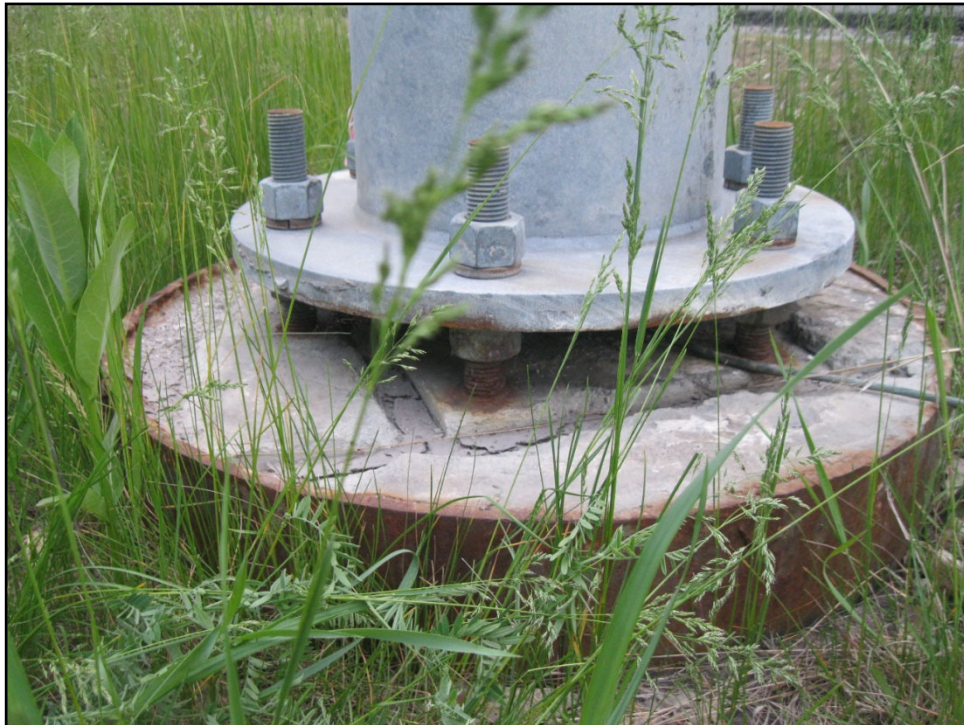
7 east foundation at base looking southwest.
