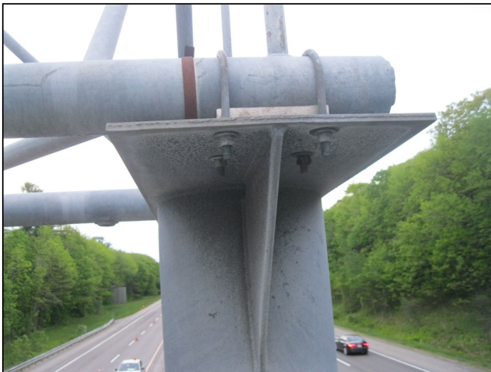
8 South lower chord saddle, looking north.
