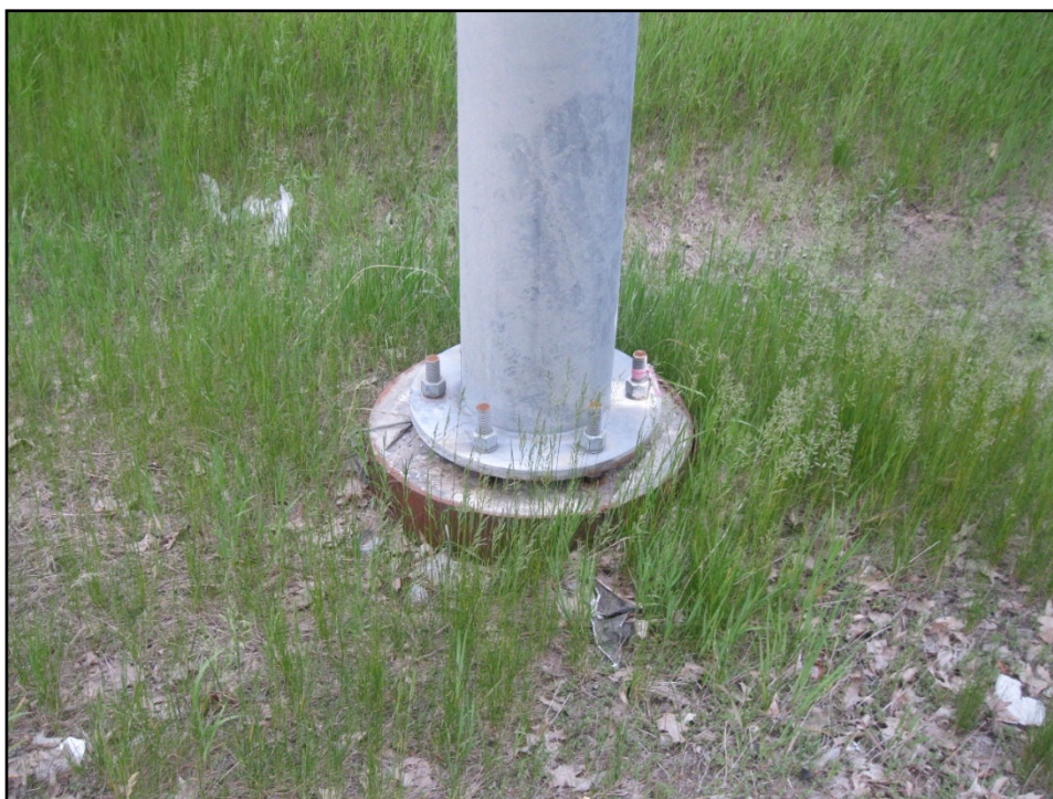
6 General view of east foundation, looking east.
