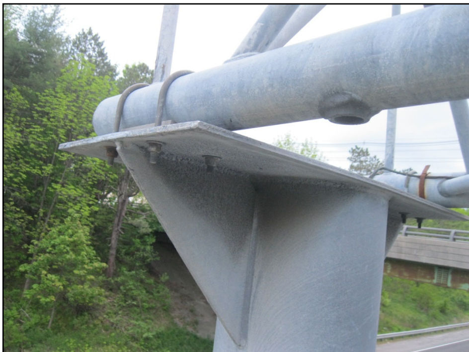
14 North lower chord west end, looking southeast.
