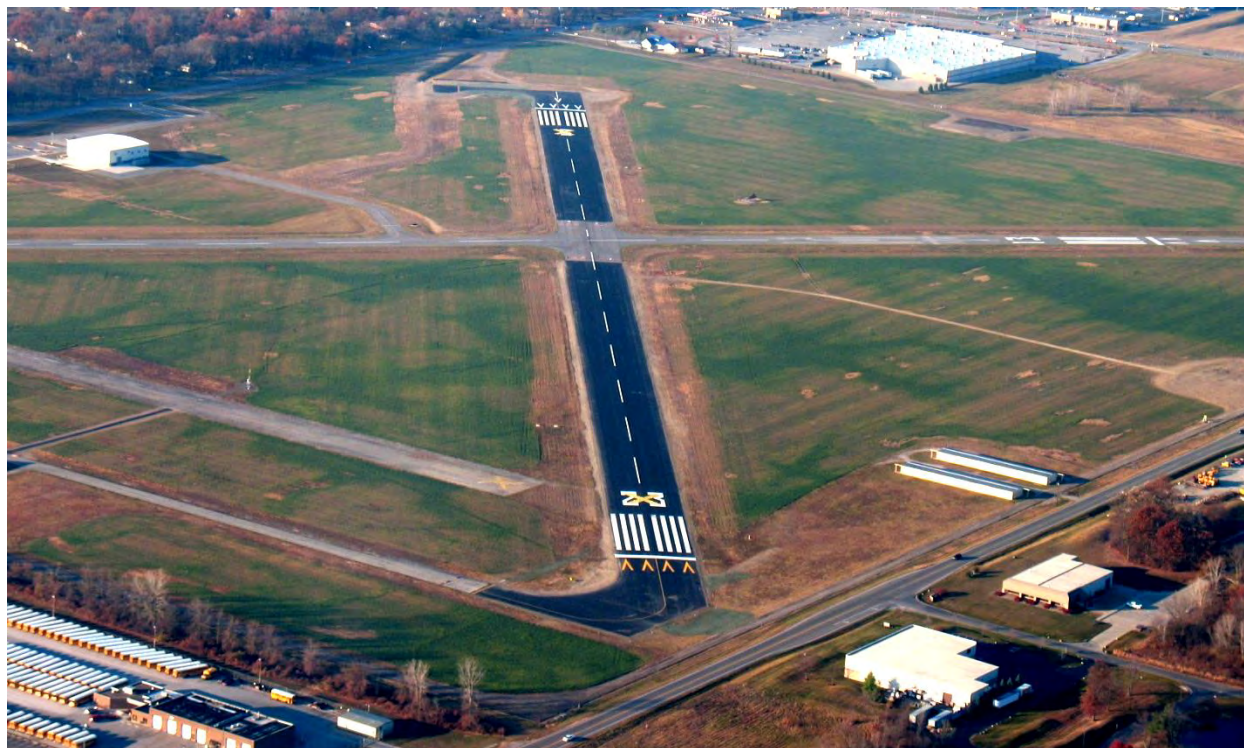
Figure 2-3. Markings for a Temporarily Closed Runway
