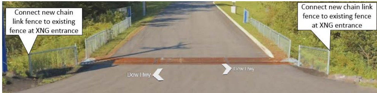
Figure 2. Fence connection points at XNG gas facility.
