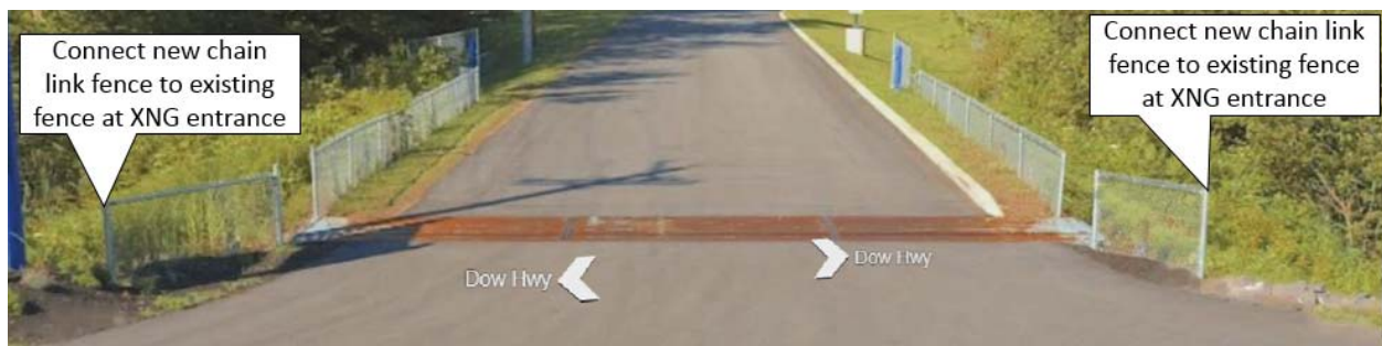
Figure 2. Fence connection points at XNG gas facility.
