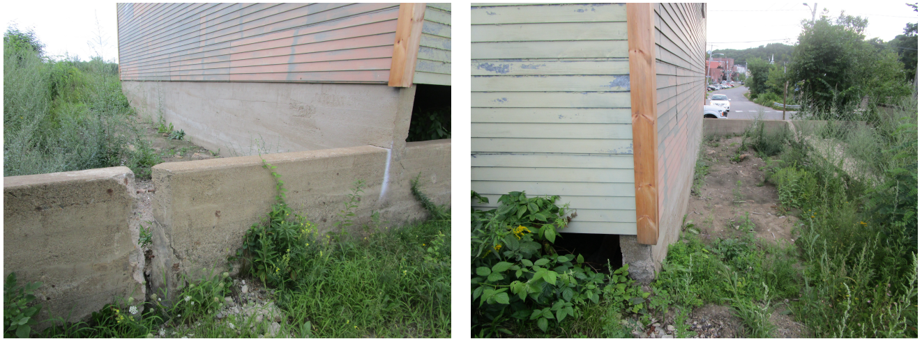
Figure 1: Building No. 3 Walls & Foundations
