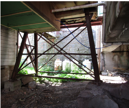
Figure 1 Below A1 Diner Looking South Towards Frosty's Foundation
