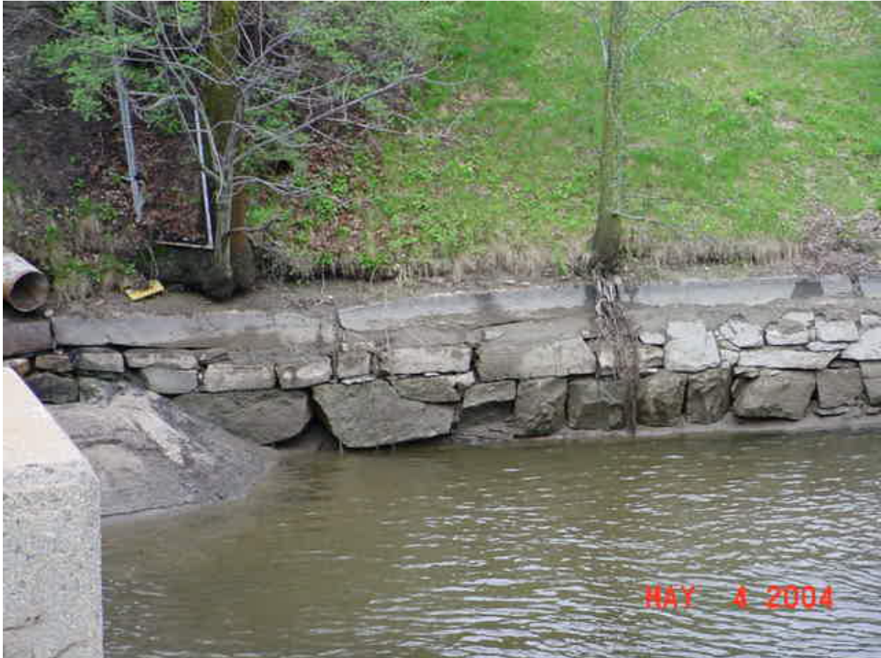
Wing 1 location from bridge
