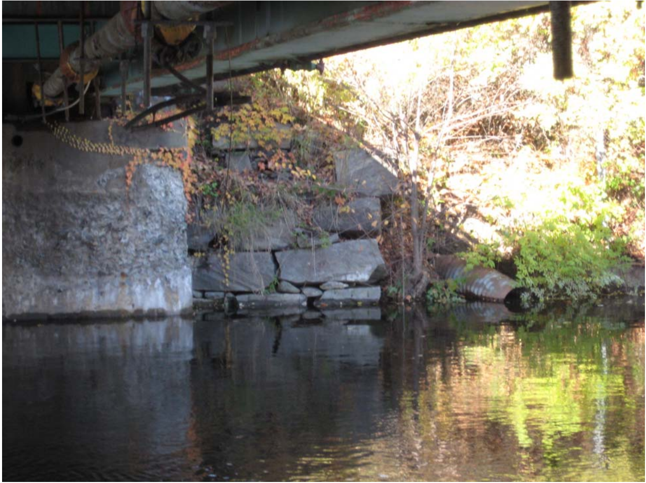
Wing 1 location from under bridge
