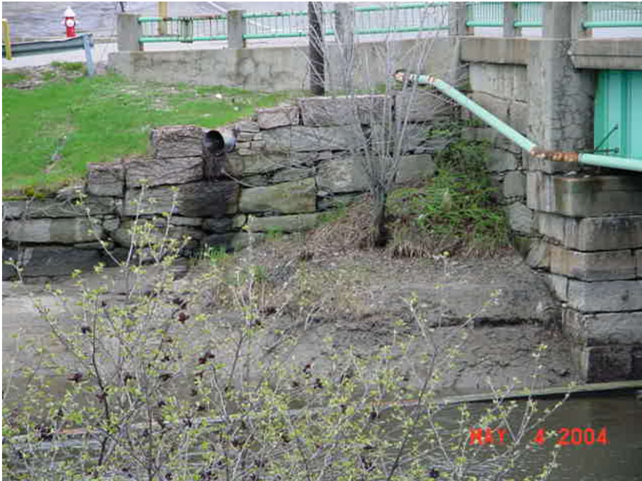
Wing 7 location, close up from the island
