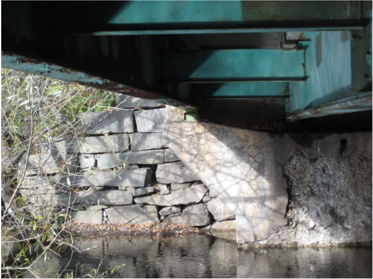
Wing 2 location from under bridge
