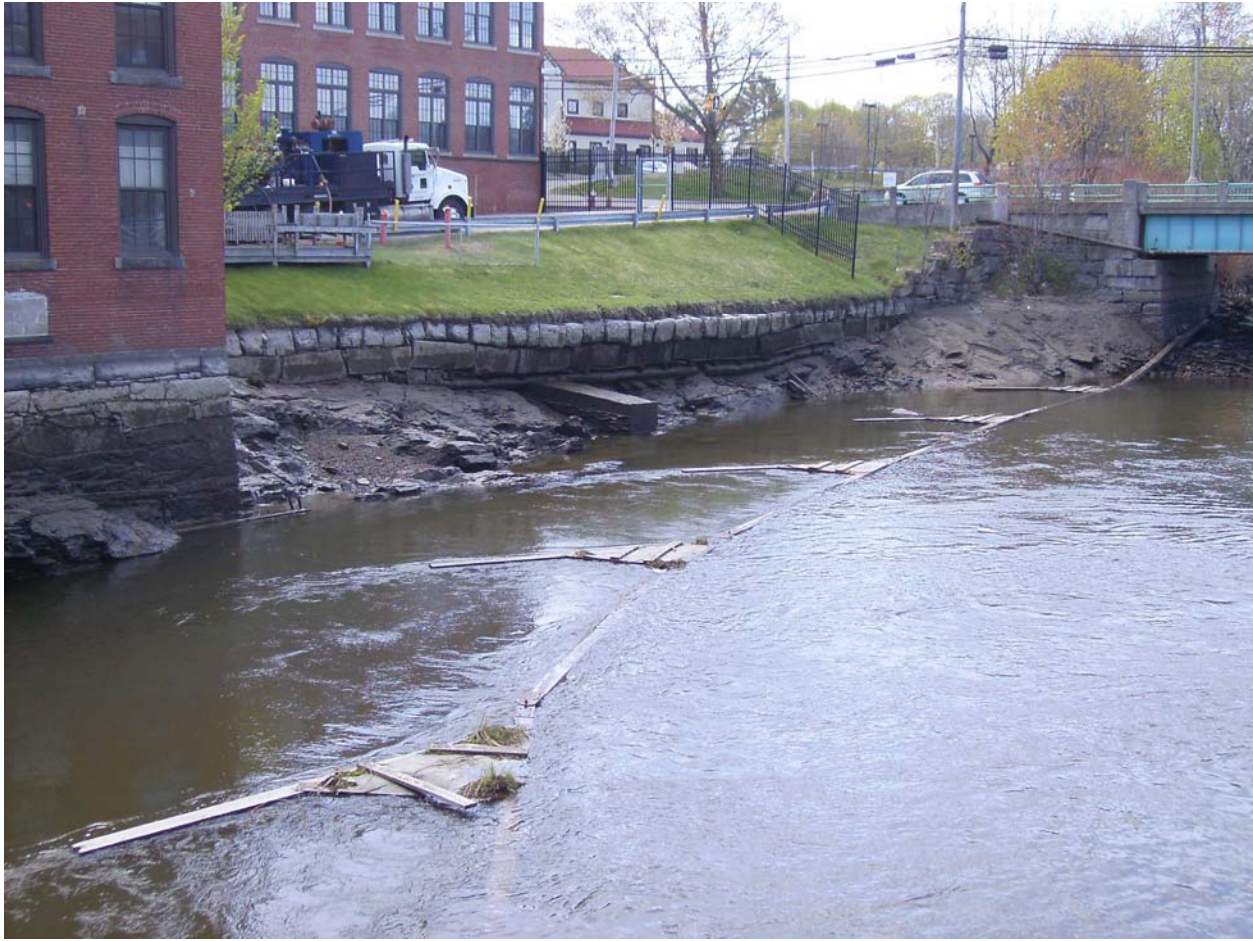
Wing 7 location, general upstream view
