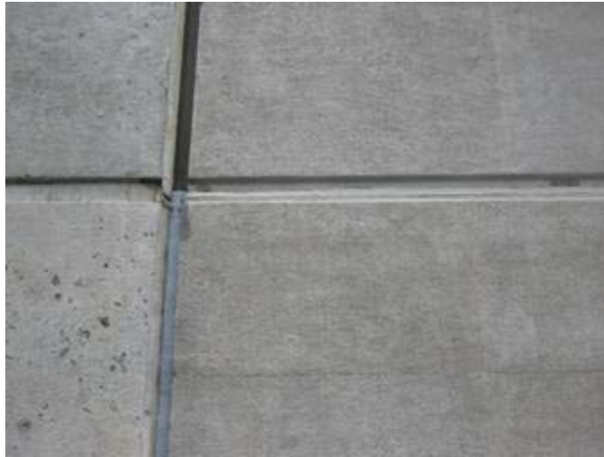
FINISHED JOINT ON BOTTOM
