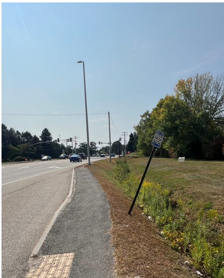
FIGURE 6 BUS STOP LOCATION WITH MISSING INFRASTRUCTURE
