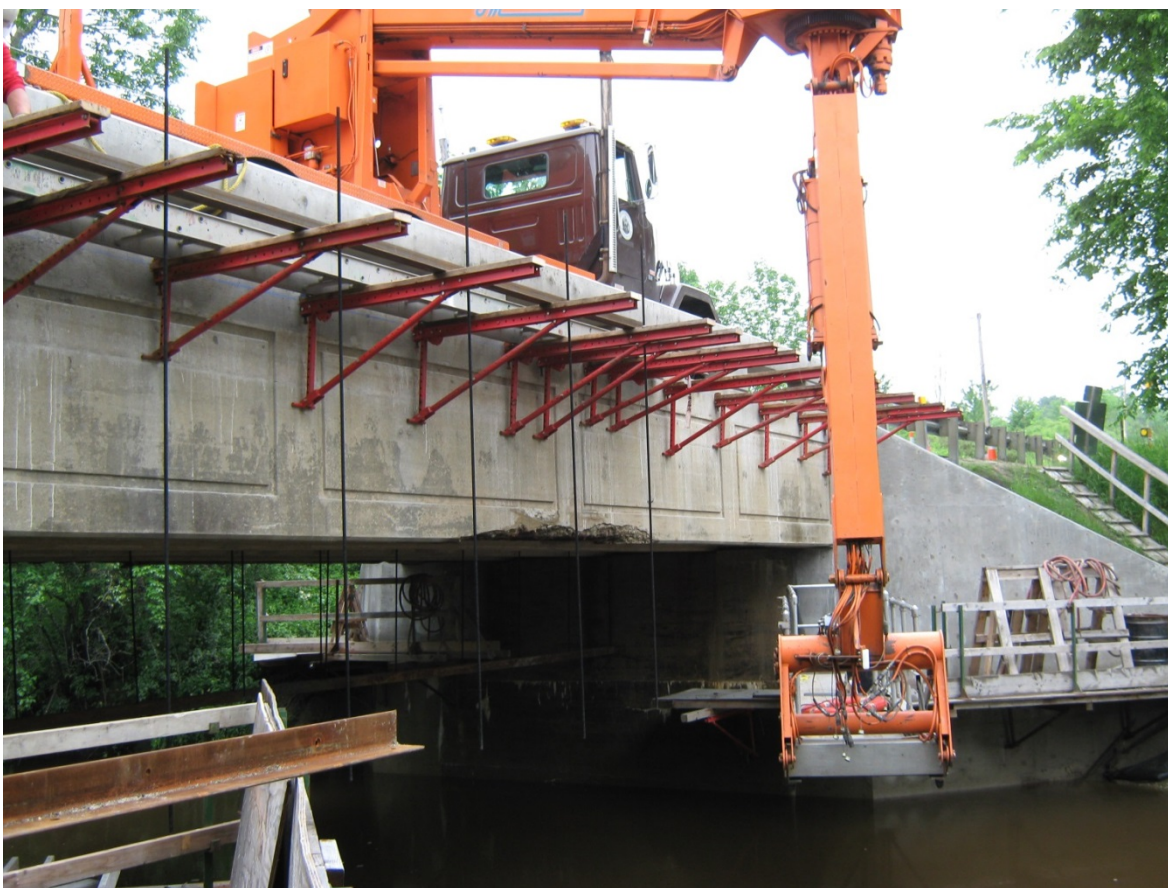
Figure 3-34. Concrete repairs on beams will be completed from staging. In this photo, the staging is attached to the wing wall.
