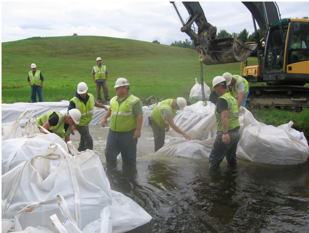
Figure 3-3. Placement of plastic sheeting under sandbag cofferdam.
