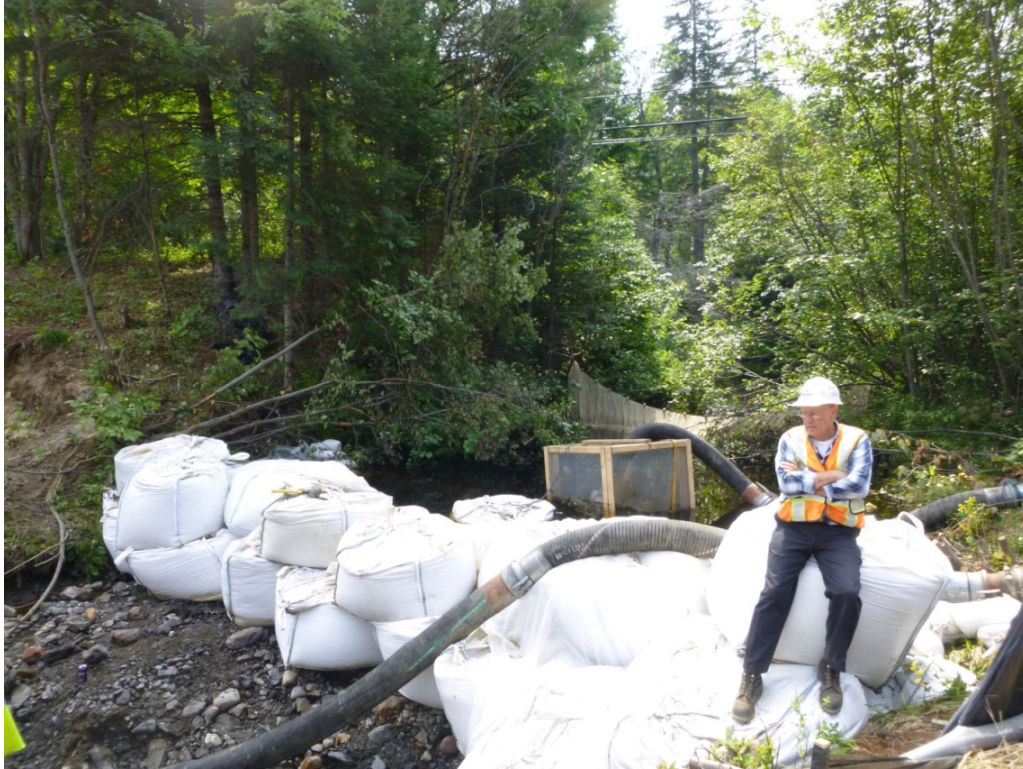
Figure 3-2. Cofferdam made of industrial sandbags. Bypass pump intake upstream of the cofferdam.
