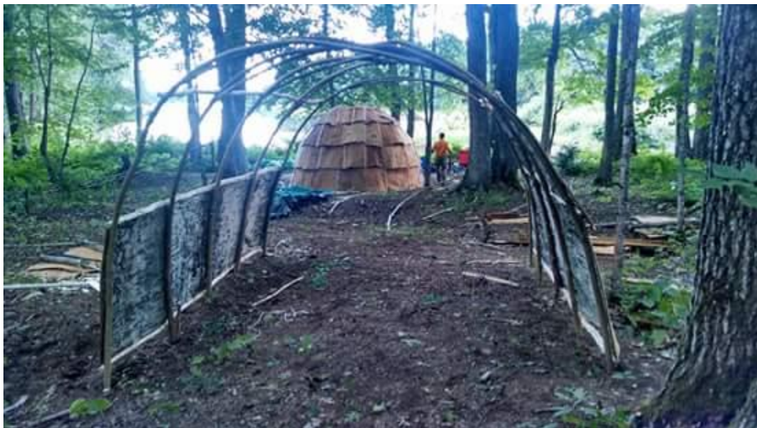
Wigwams in the construction process using geometry and measuring by the Penobscot Nation.
