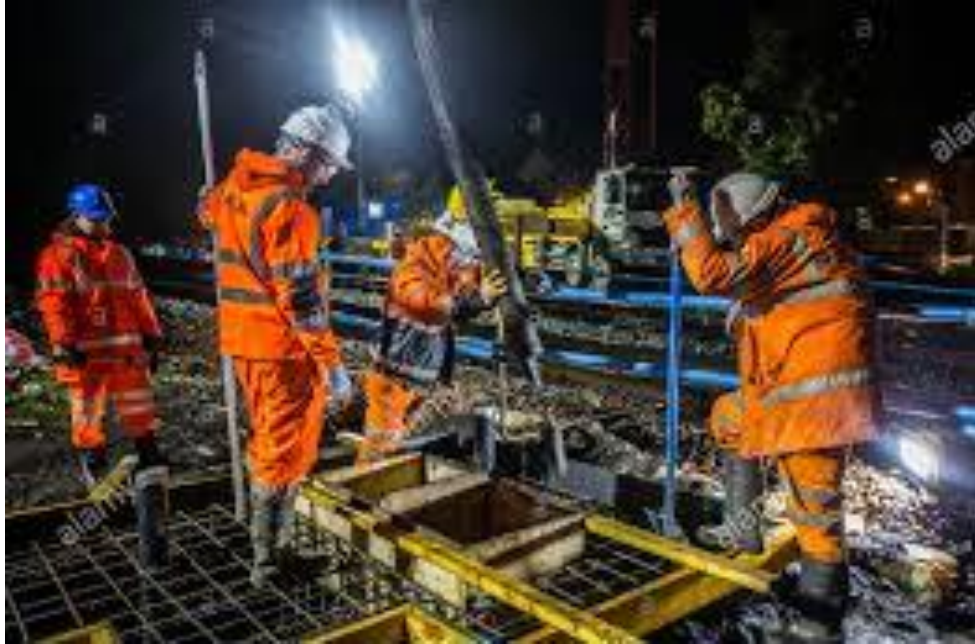
Construction workers work at night.
