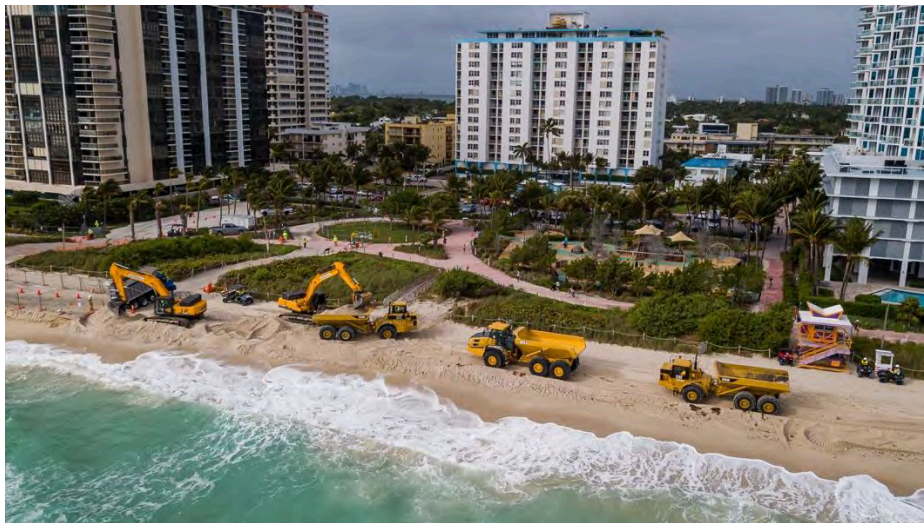
Photograph 2: In Miami Beach, people are trying to slow down the erosion caused by sea level rise, storms, and apartment buildings by adding more sand on the beach.
