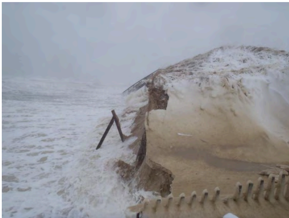
Erosion underway at Cold Storage Beach in Dennis
