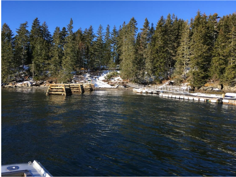
Image 3: Ramps, floats, and partially constructed pier located on the eastern shore of Seal Island (December 20, 2017). 6
