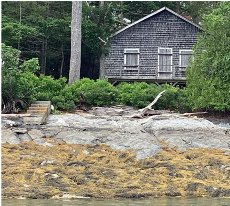
Image 1. Concrete stairs leading to the shoreline
