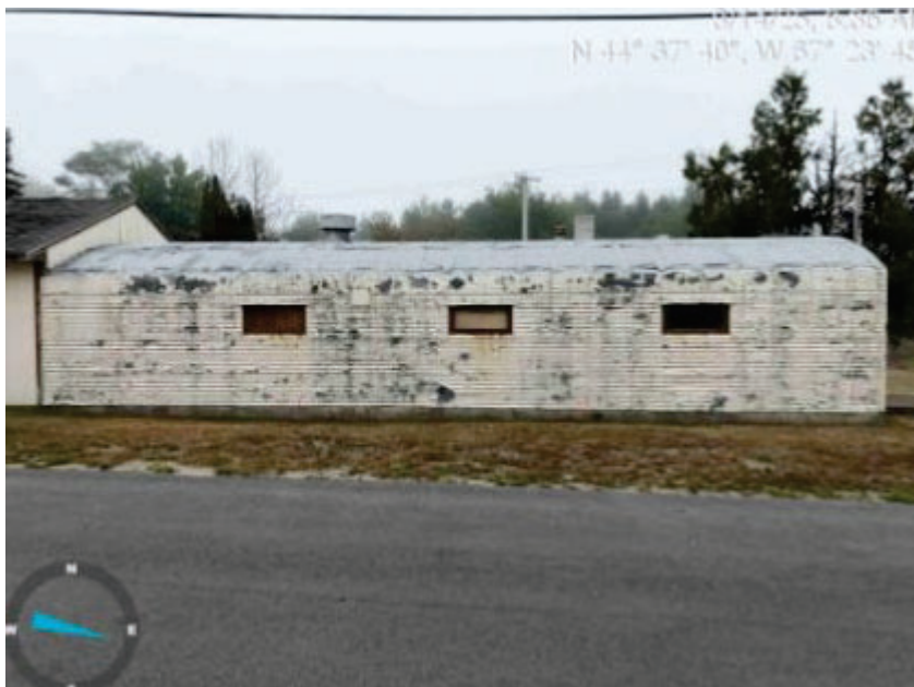
Figure 2. View of the QYA ARSR building D West exterior.
