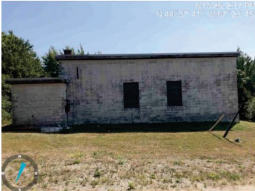
Figure 3. View of the QYA ARSR Building A exterior looking North.
