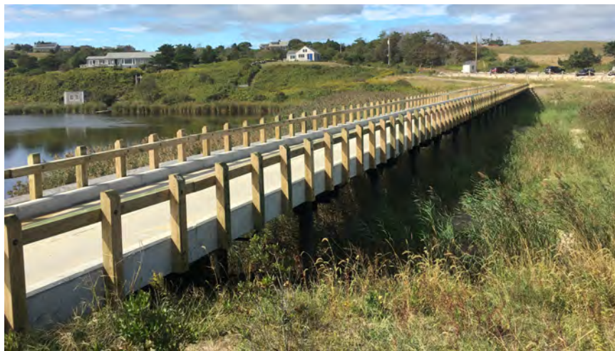
FIGURE B.2 - Single-lane bridge on piers in Chilmark, Massachusetts, that spans an area projected to flood more frequently with sea level rise. Photo by Slade Moore.
