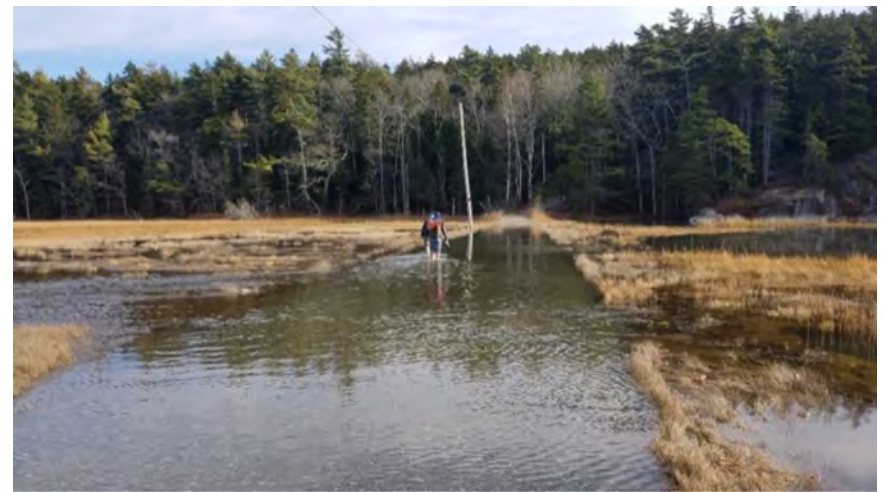
FIGURE B.3 - Example of a "fair-weather" road that overtops with a similar frequency as the adjacent marsh in Phippsburg. Photo by Erno Bonebakker.
