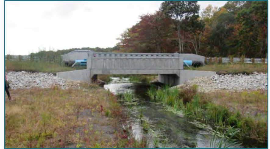
FIGURE B.6- A three-sided concrete rigid frame structure, installed on pre-cast footings. Clear span of 24 feet. Structure includes a pre-cast modular design with six-foot-long sections. Due to cover limitations within the road prism, an insulated water line was attached to side of headwall. Coonamesett River, Falmouth, MA. Image source: Inter-Fluve.
