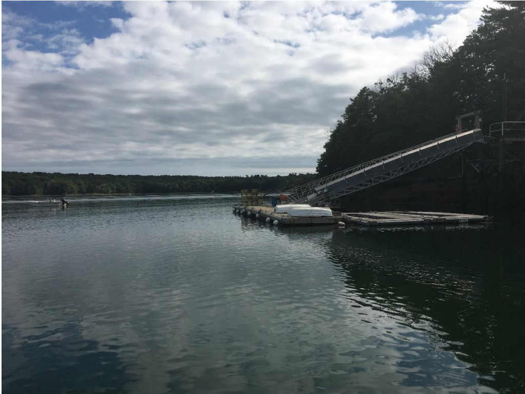
Image 5: Facing south toward the applicant’s dock from near the center of the proposed lease site (September 17, 2021).
