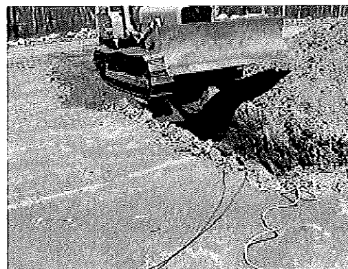
Backfill with Dozer
