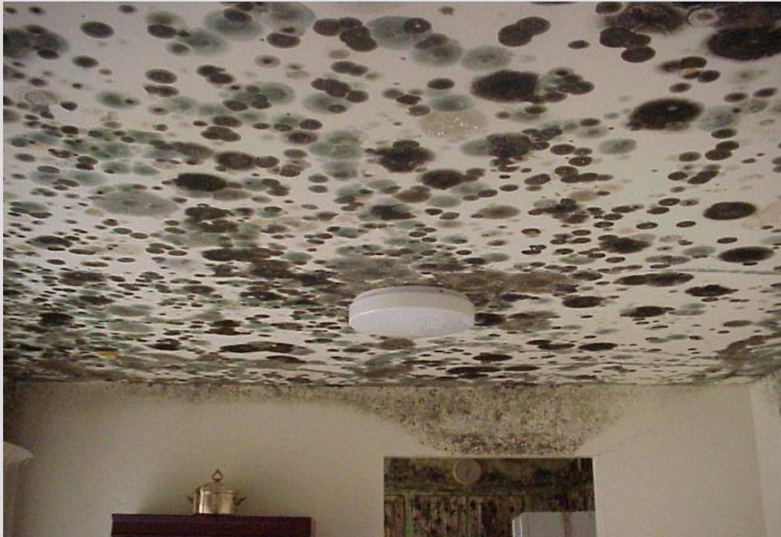
Mold growing on the ceiling.
