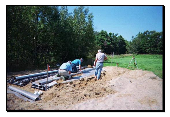
Figure 18. Installation of a cuspated block gravel-less bed.
