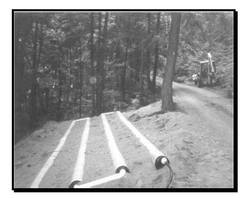
Figure 16. Fabric covered tubes installed for serial distribution.
