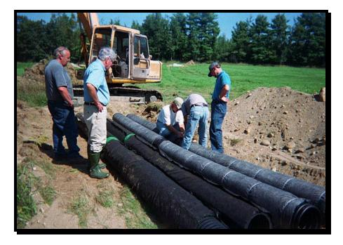
Figure 15. Fabric covered tube installation
